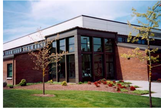
Figure 3.1: Typical building entrance
