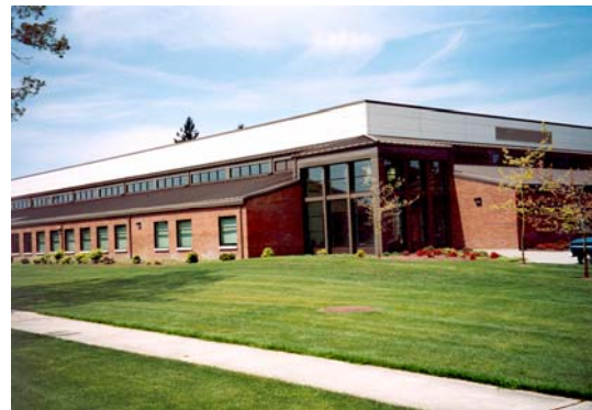
Figure 3.2: Typical view of building entrance from access point
