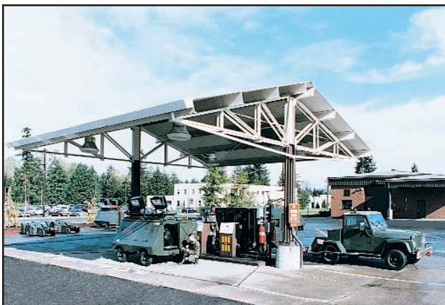
A covered refueling island provides shelter from the elements.
