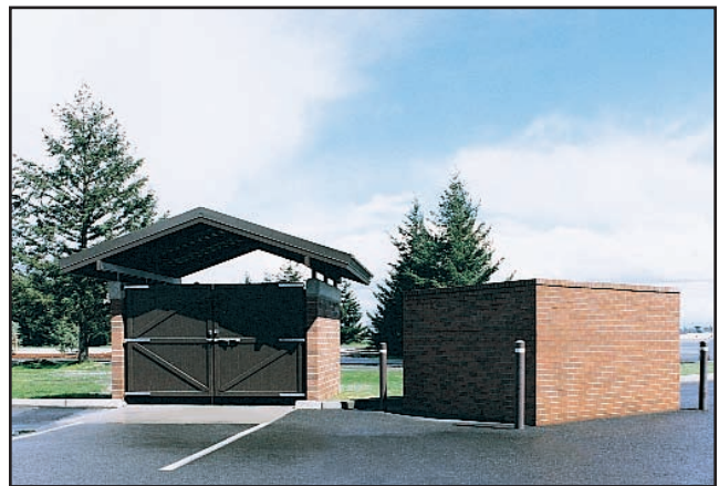
Architectural screening of utilitarian items enhances overall appearance.
