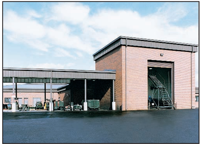
High bay access is required for oversized equipment.
