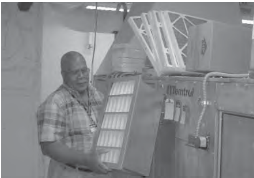
Building equipment maintenance
