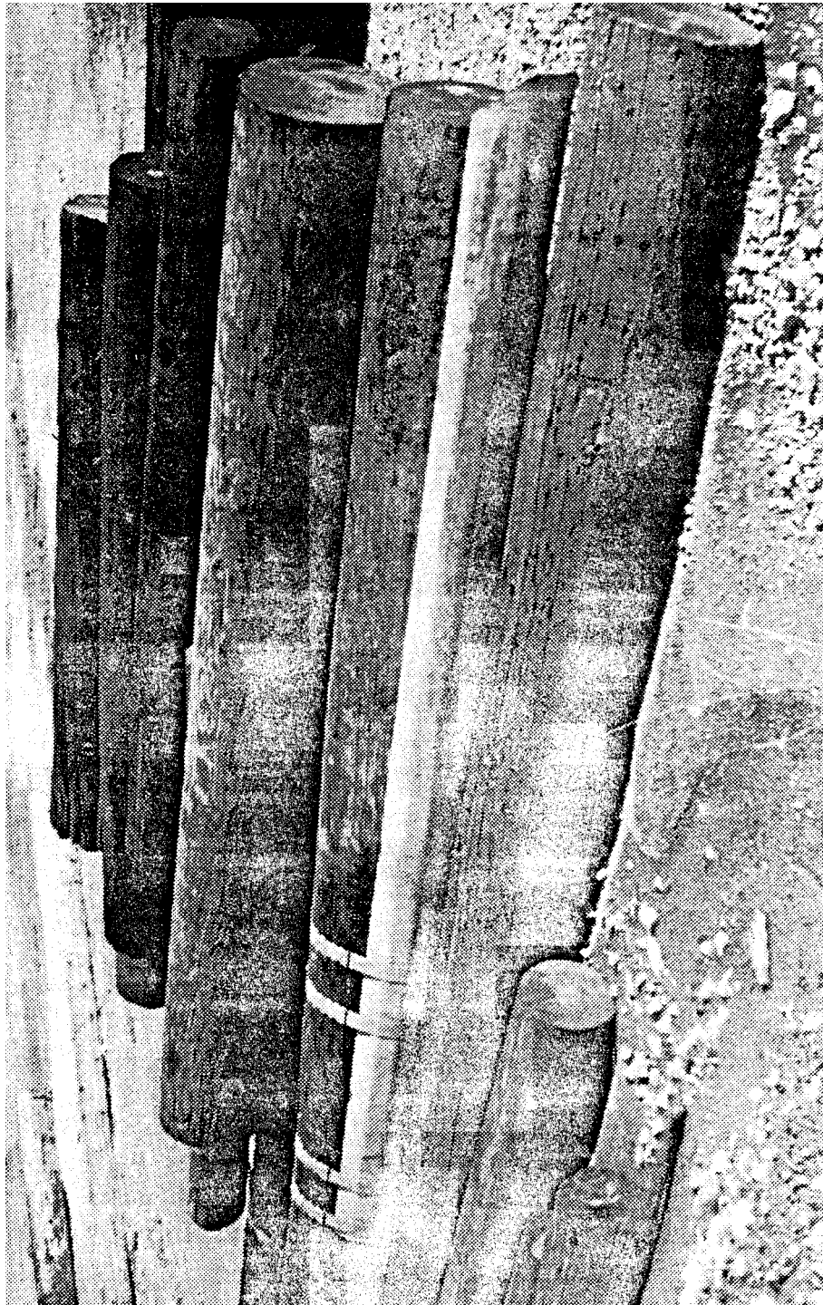
FIGURE 7-7 A Metal Stub was used to Reinforce this Pole Before it was Removed from Service
