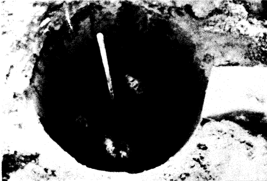
Figure 2-31. Installation of an Electrode During the Process of Backfilling with a Salt-Soil Mixture
