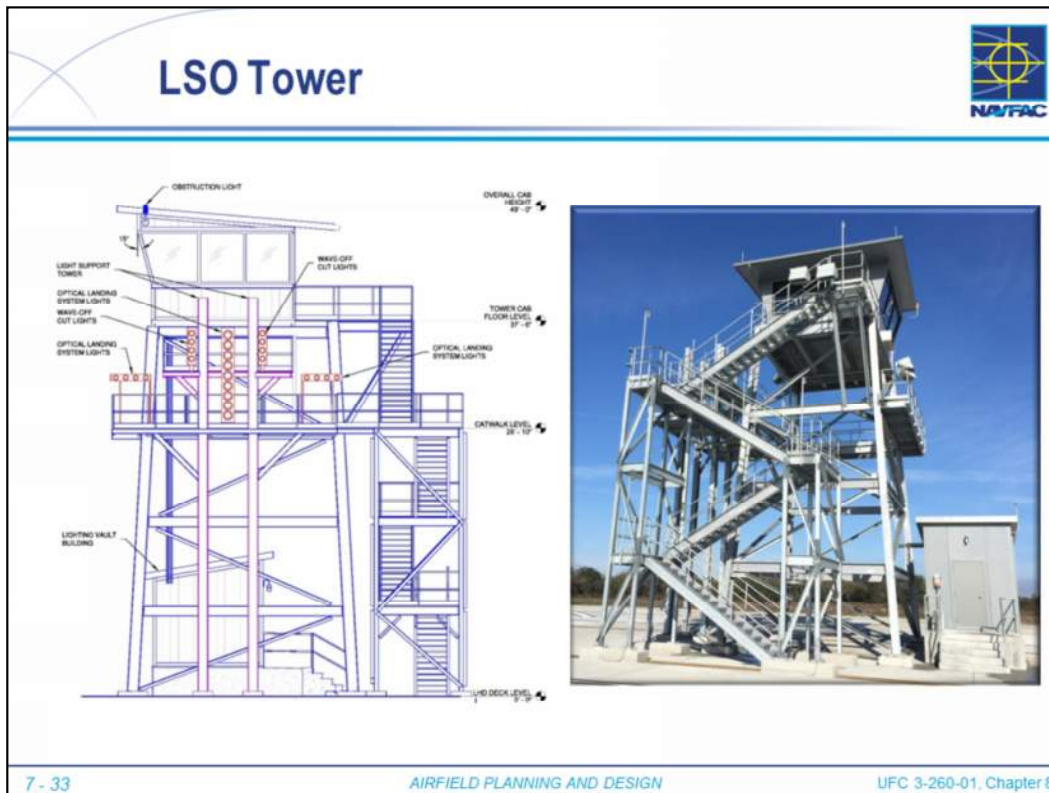
Figure 8-20. LHD LSO Tower.
