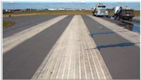
IPRF Figure 4-1. Before Cleaning Loose and Poorly Bonded Paint
