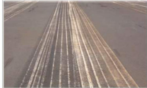
IPRF Figure 4-2. After Cleaning Loose and Poorly Bonded Paint by Waterblasting
