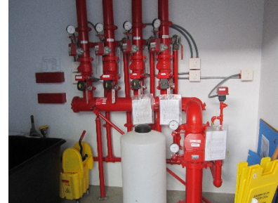
Figure 28 –Sprinkler Lines
