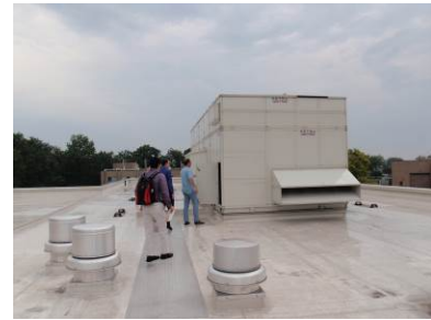
Figure 35 - Rooftop AHU
