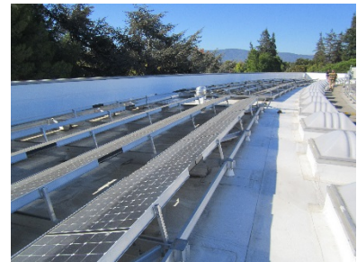
Figure 5 – Photovoltaic Panel Array
