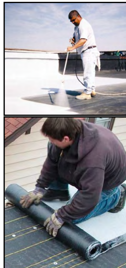
Figure 6: Two Cool Roof Installations
