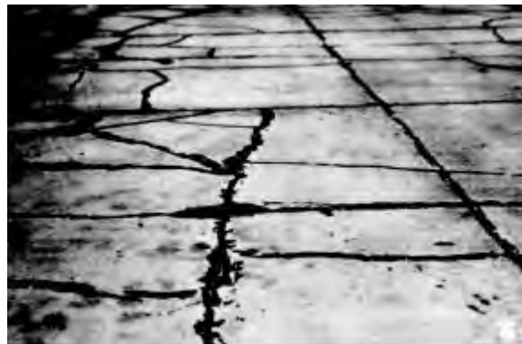
Figure 14.6. Shattered slab
