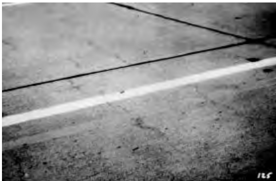
Figure 15.3. Shrinkage cracks
