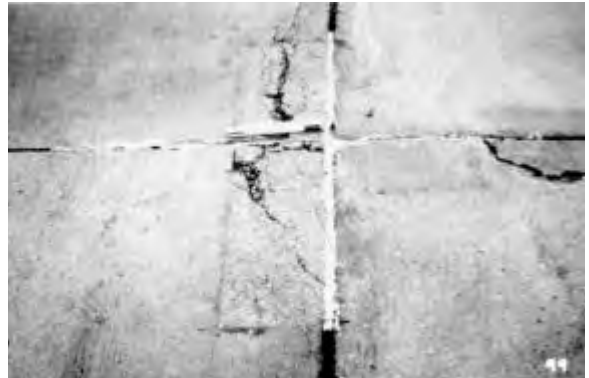
Figure 8.6. High-severity small patch
