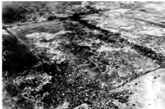
Figure 12.4. High-severity scaling
