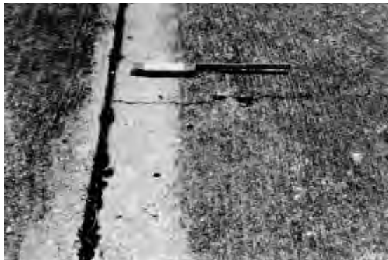
Figure 15.2. Shrinkage crack
