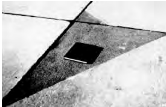
Figure 9.2. Low-severity patch
