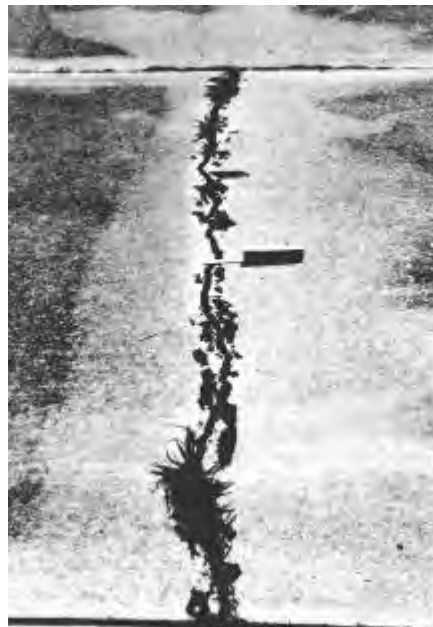
Figure 5.10. High-severity crack
