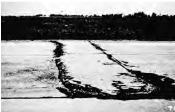
Figure 3.3. Medium-severity blowup
