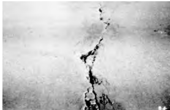
Figure 5.8. High-severity crack
