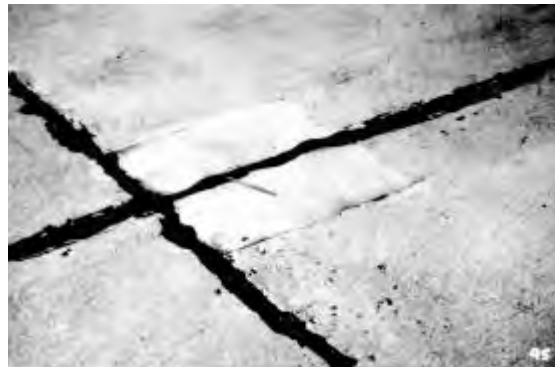
Figure 8.2. Low-severity small patch
