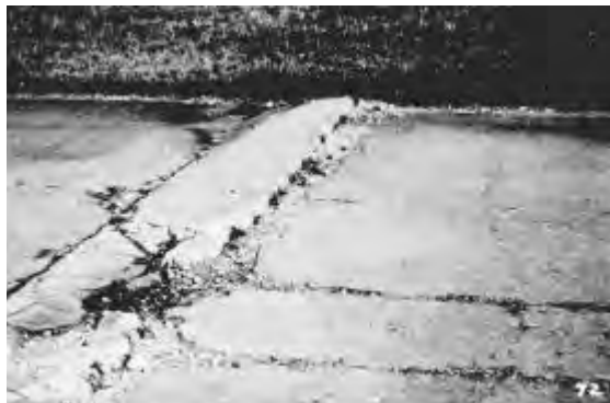
Figure 3.4. High-severity blowup
