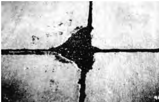
Figure 8.3. Low-severity small patch
