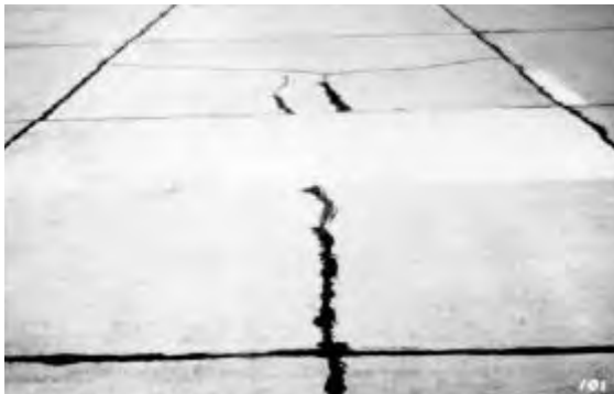
Figure 9.3. Low-severity patch
