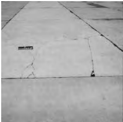
Figure 4.1. Shattered slab
