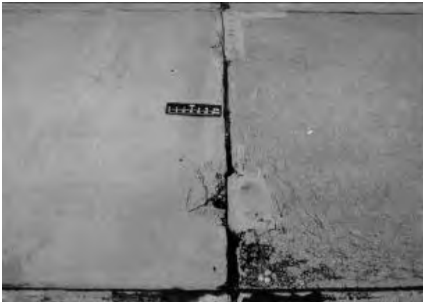
Figure 5.8. Point bearing causing failure
