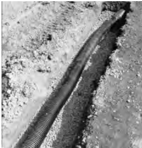
Figure 12.3. Flexible drainage pipe
