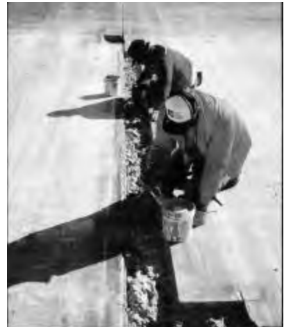
Figure 5.9 Application of bonding agent
