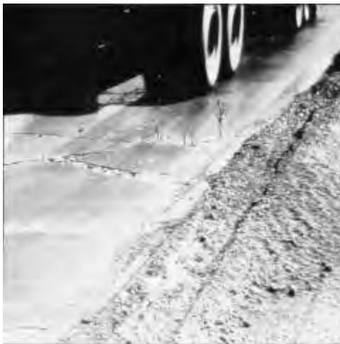
Figure 12.1. Pavement pumping
