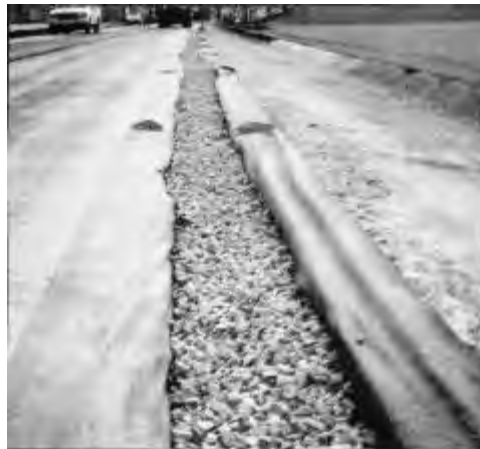
Figure 12.6. Lined trench with coarse backfill
