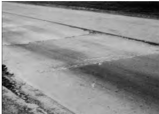
Figure 5.2. Severe spalling
