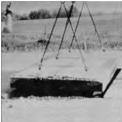
Figure 4.9. Lift-out method
