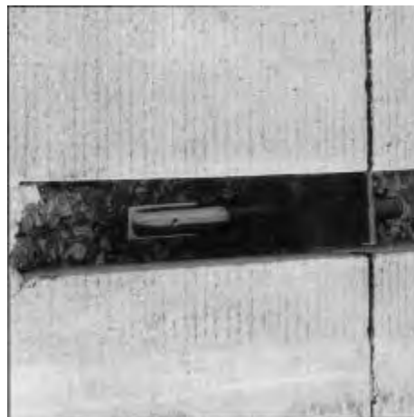
Figure 10.2. Forming joint in slot
