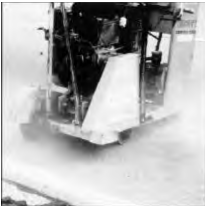
Figure 4.5, Diamond blade sawing
