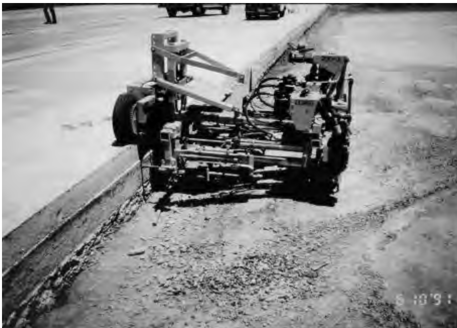
Figure 4.14. Drilling multiple holes
