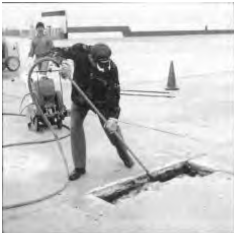
Figure 5.6. Cleaning exposed faces
