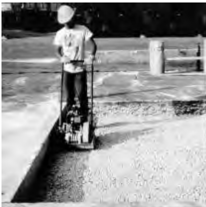
Figure 4.11. Patch area compaction
