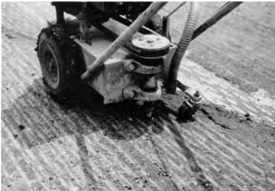
Figure 6.1. Vertical spindle router
