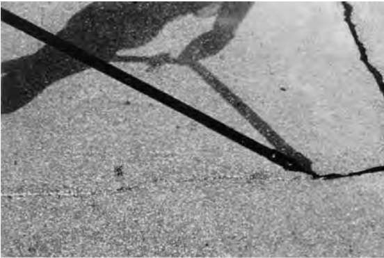
Figure 9.3. Sealing the crack
