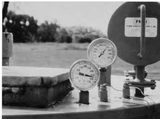
Figure 8.2. Thermometers measuring sealant and oil bath temperature
