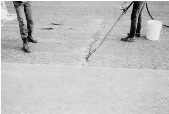
Figure 9.1. Filling crack with sand emulsion mixture
