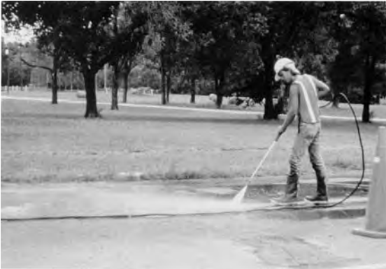
Figure 6.5. High-pressure water cleaning equipment
