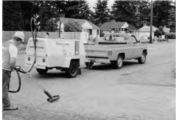
Figure 6.6. Hot compressed-air heat lance
