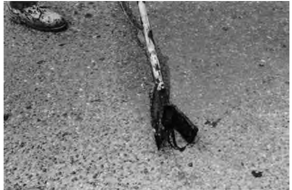
Figure 9.4. Using a squeegee to remove excess sealant
