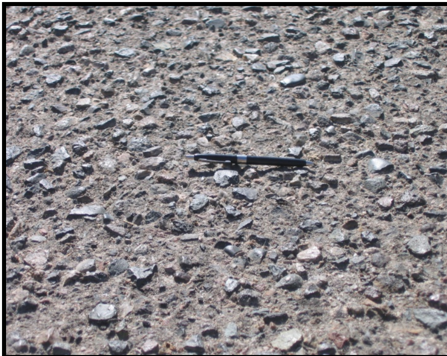
Figure A-56 High-Severity Weathering
