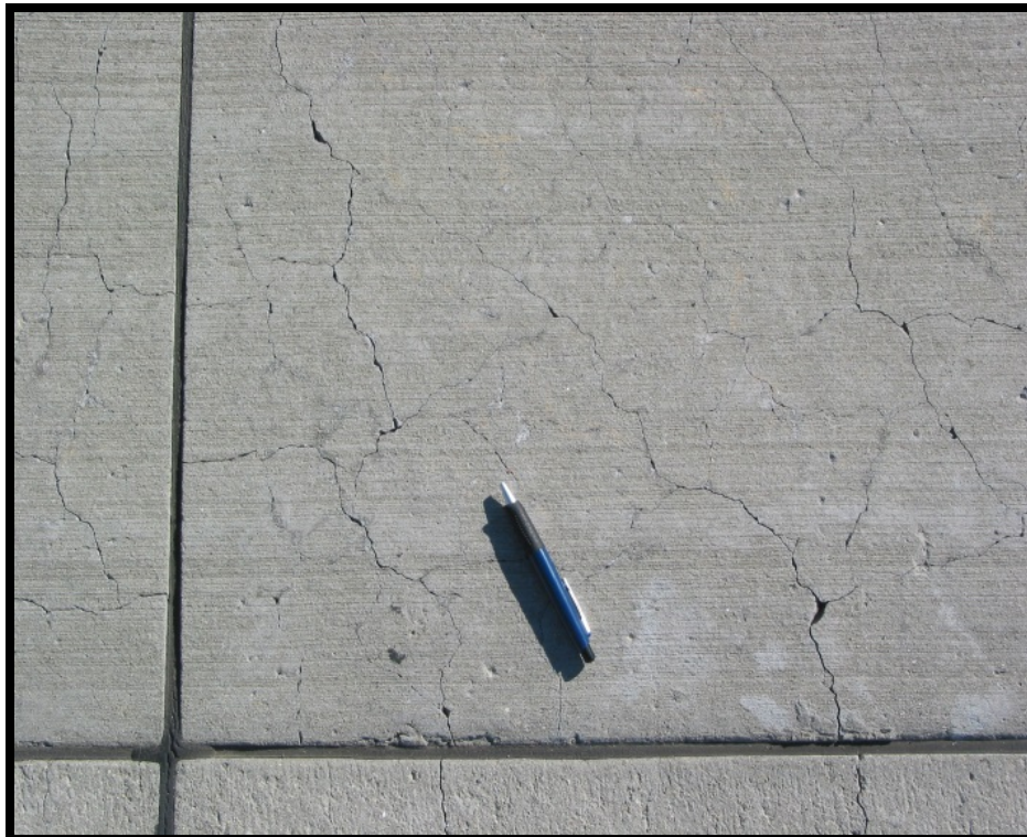
Figure B-45 Medium-Severity ASR
