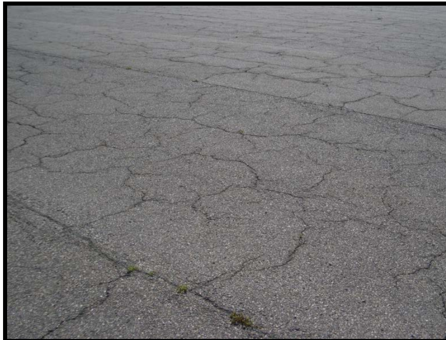
Figure A-10 High-Severity Block Cracking
