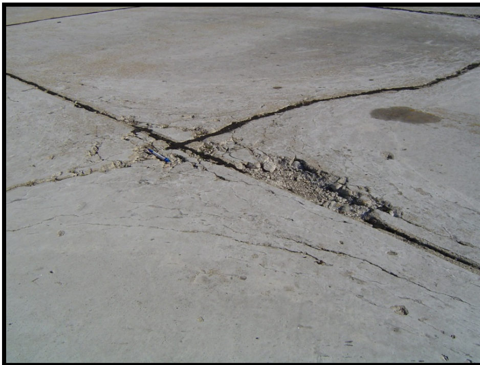
Figure B-14 High-Severity “D” Cracking
