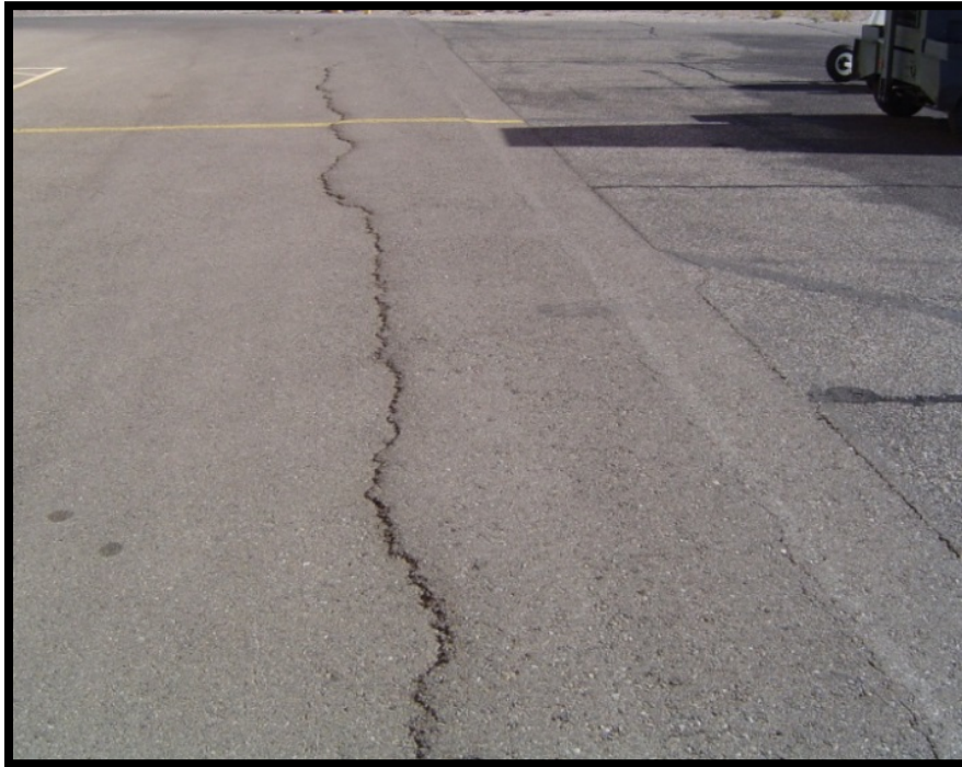
Figure A-48 Medium-Severity Shoving
