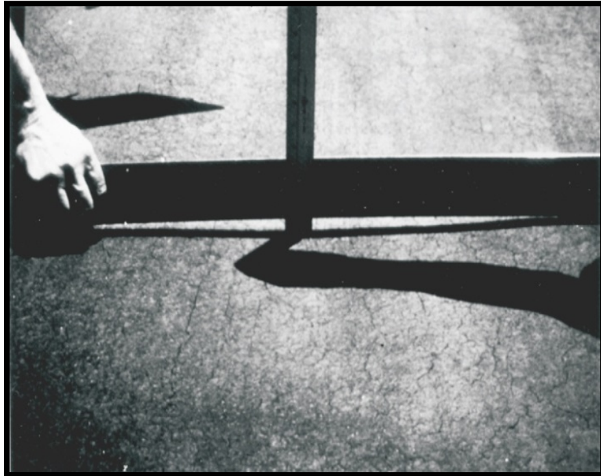
Figure A-18 High-Severity Depression
