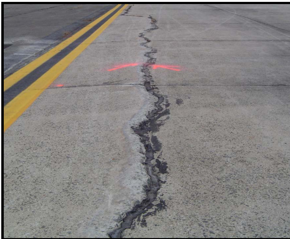
Figure B-2 Low-Severity Blowup
