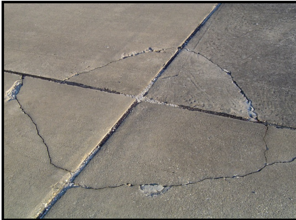
Figure B-6 Medium-Severity Corner Break
