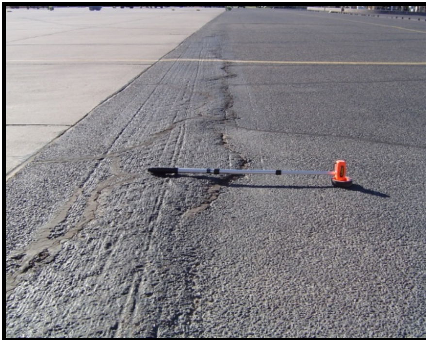
Figure A-48 Medium-Severity Shoving
