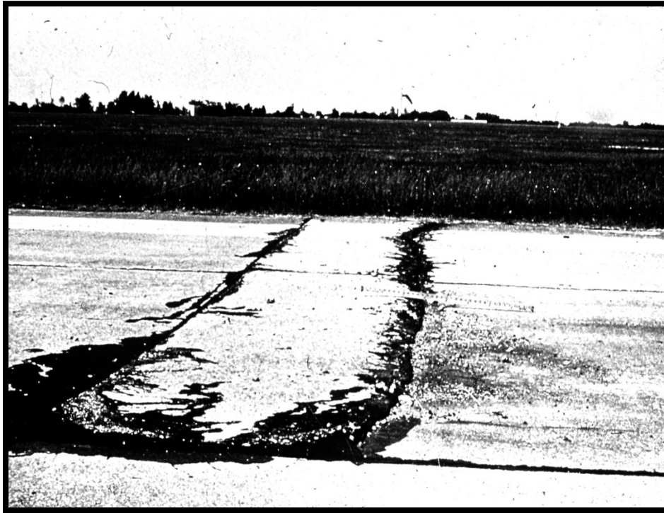
Figure B-4 High-Severity Blowup
