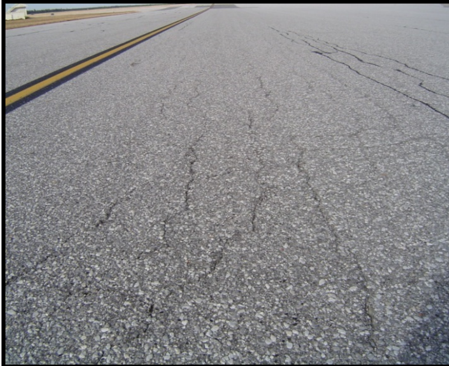
Figure A-2 Medium-Severity Alligator Cracking
