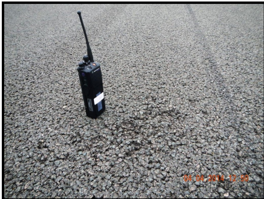
Figure A-44 Medium-Severity Raveling (PFC)
