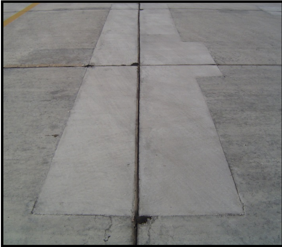
Figure B-22 Medium-Severity Large Patch
