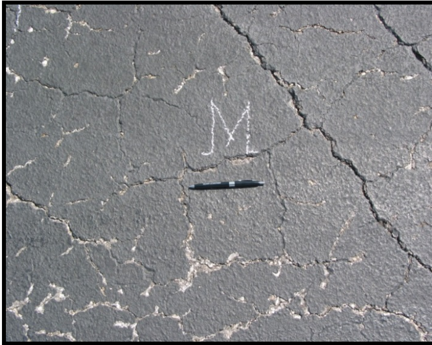
Figure A-41 High-Severity Raveling (Slurry Seal/Coal Tar Over Dense Mix)
