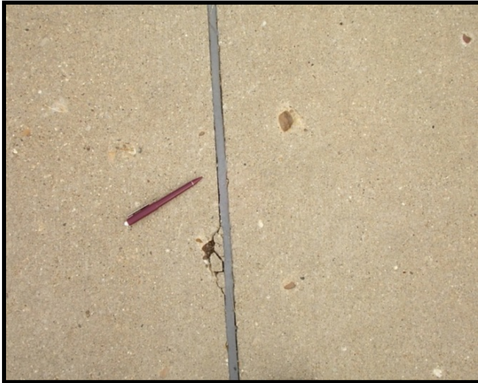
Figure B-38 Medium-Severity Joint Spall
