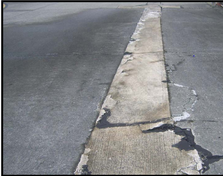
Figure B-2 Low-Severity Blowup
