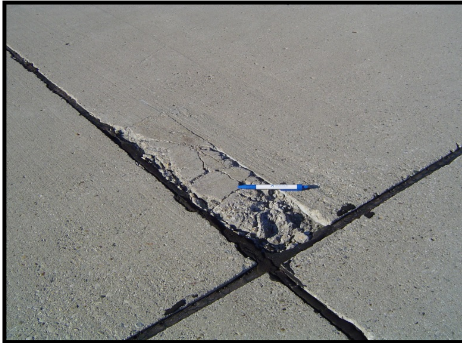
Figure B-20 High-Severity Small Patch
