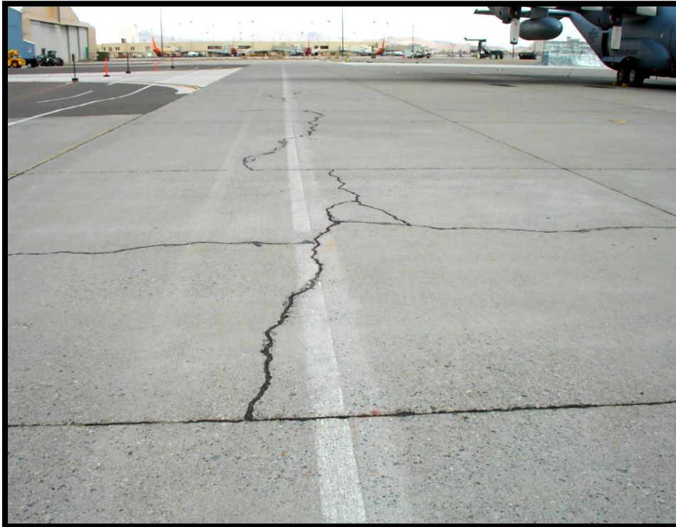
Figure B-35 High-Severity Shattered Slab/Intersecting Cracks
