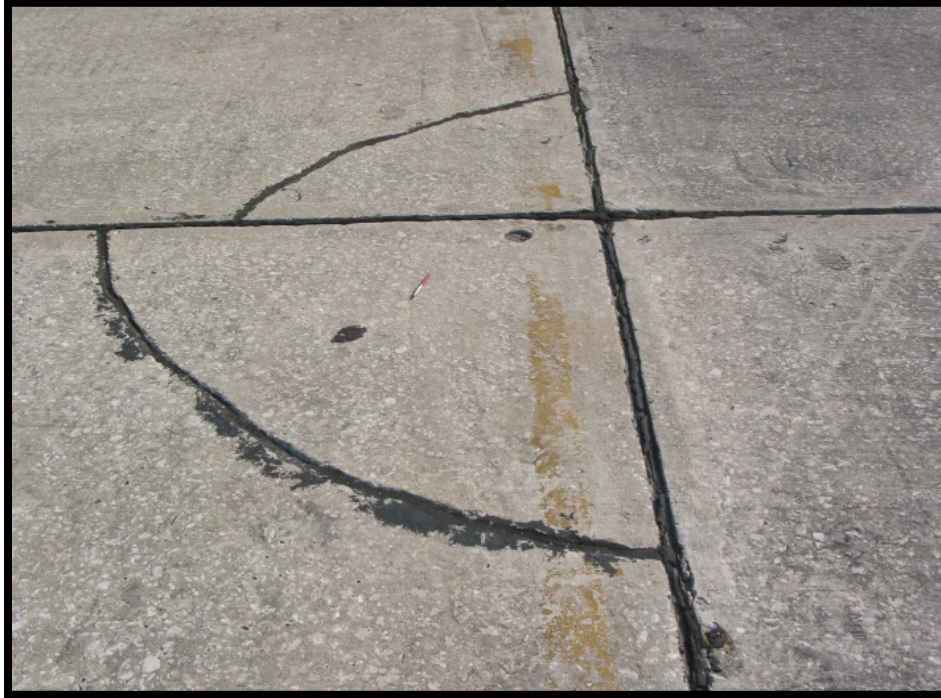
Figure B-6 Medium-Severity Corner Break
