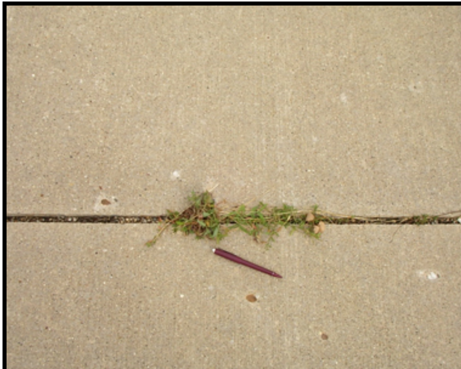
Figure B-17 High-Severity Joint Seal Damage
