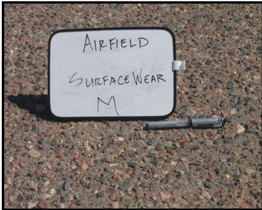
Figure A-56 High-Severity Weathering
