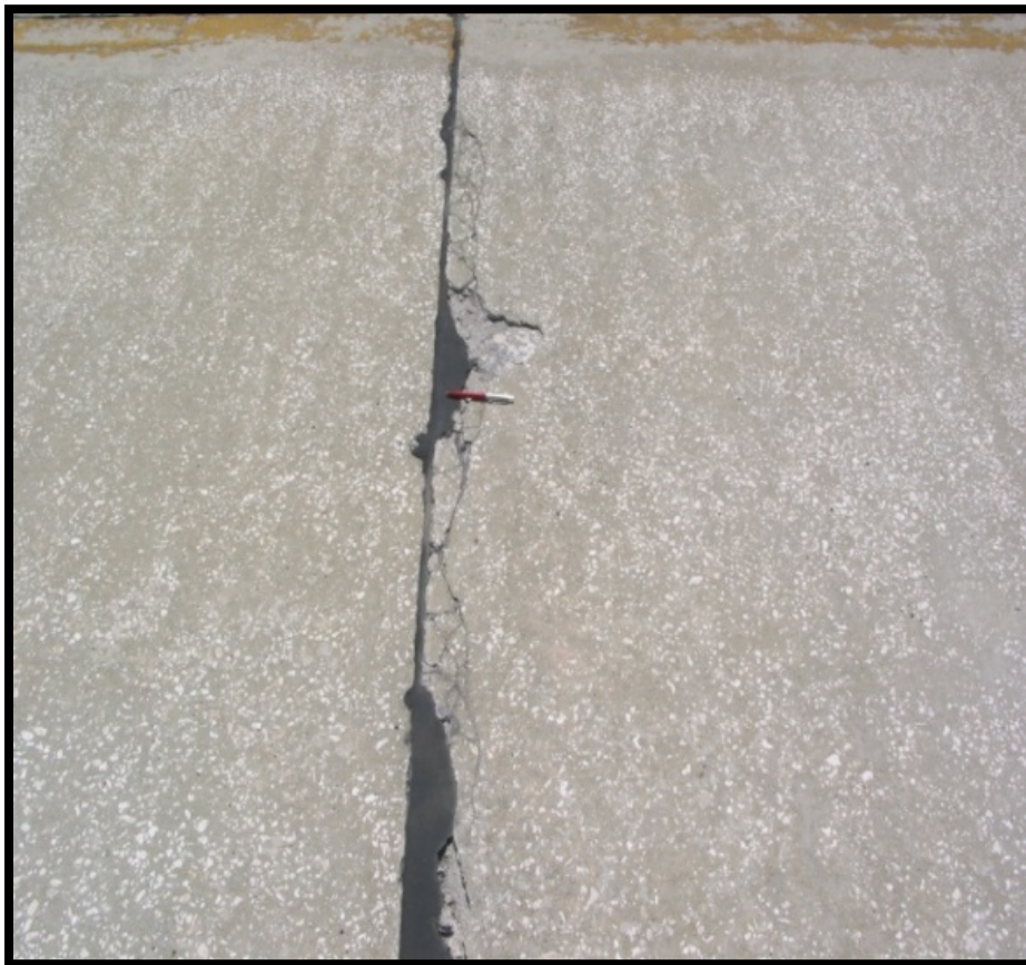
Figure B-40 High-Severity Joint Spall
