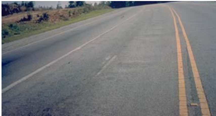
Figure A-14 Medium-Severity Corrugation
