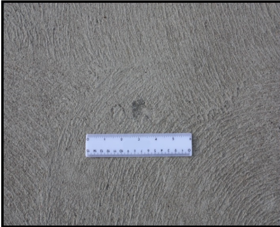
Figure B-28 Medium-Severity Scaling
