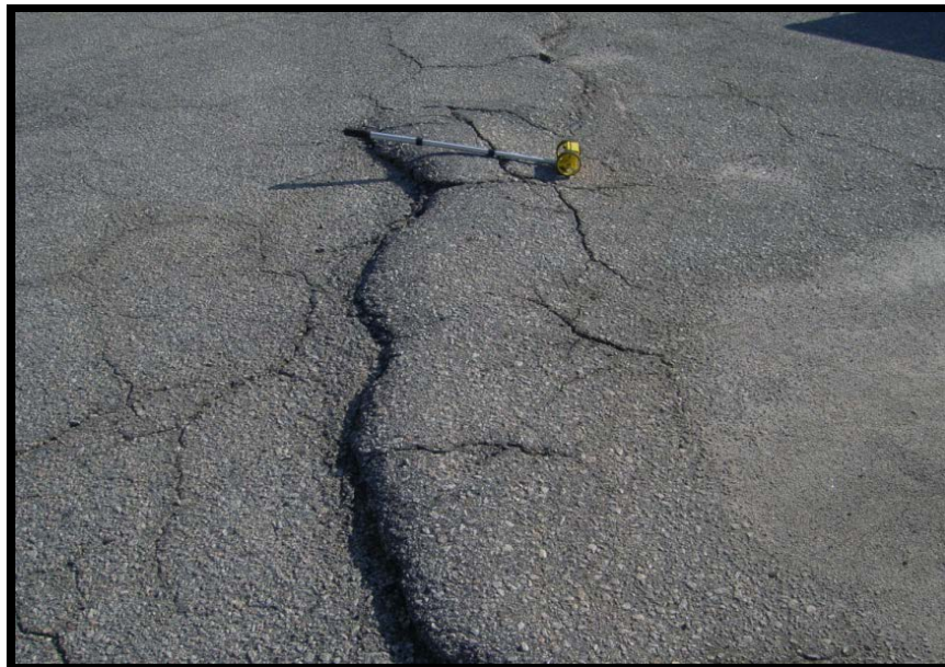
Figure A-53 High-Severity Swell
