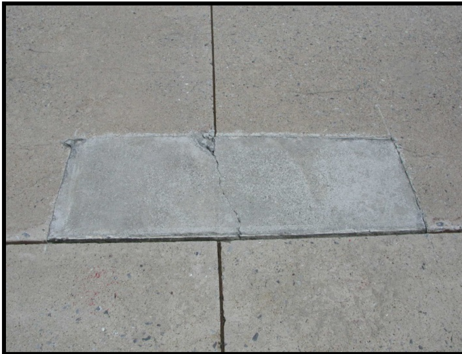
Figure B-19 Medium-Severity Small Patch
