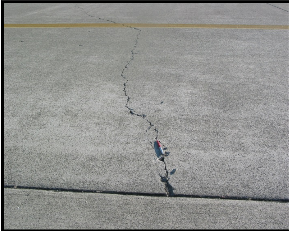
Figure B-10 High-Severity Linear Cracks
