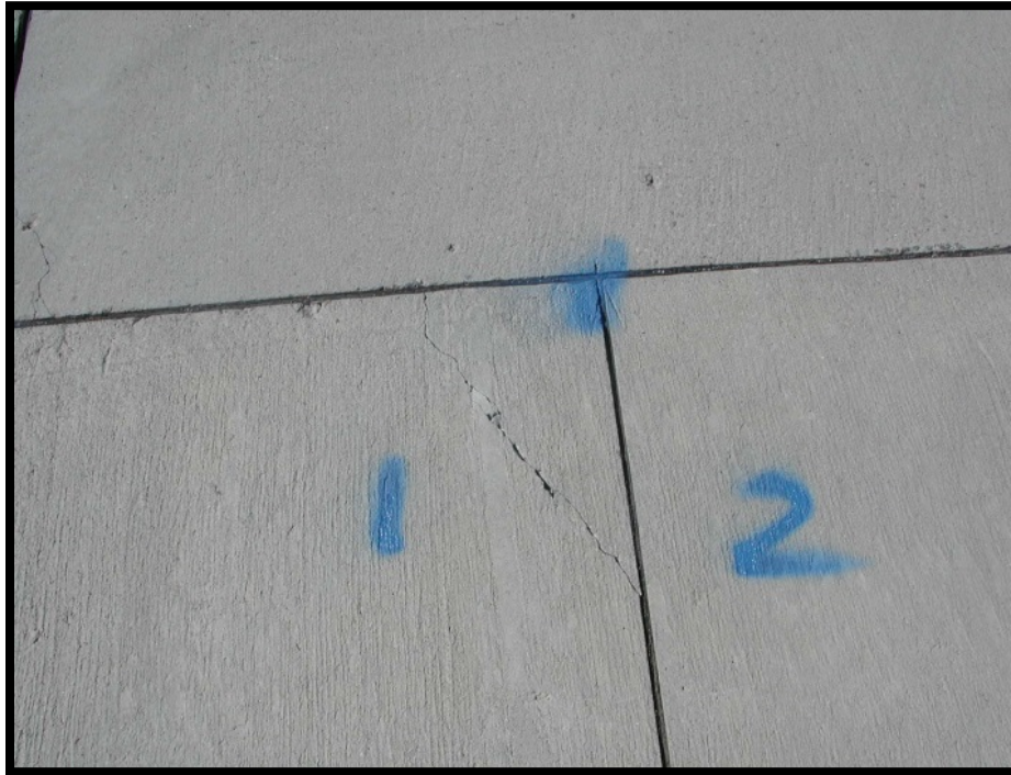
Figure B-42 Medium-Severity Corner Spall
