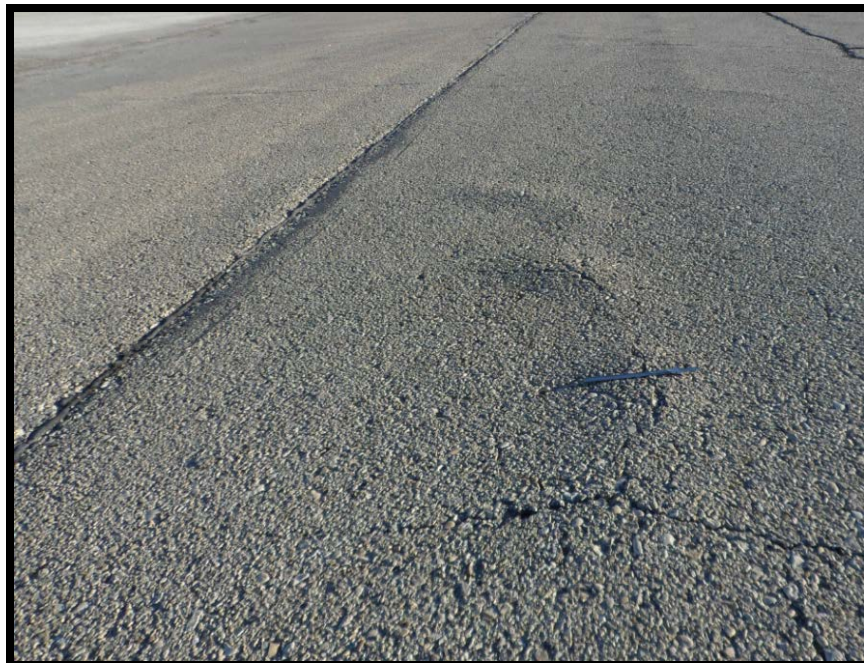
Figure A-51 Low-Severity Swell
