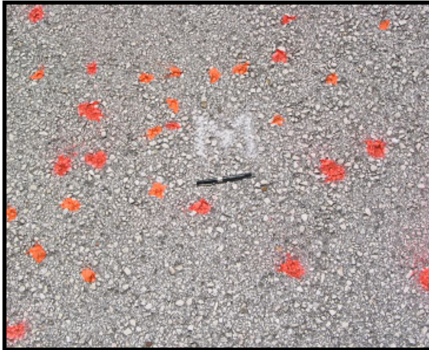
Figure A-38 High-Severity Raveling (Dense Mix)
