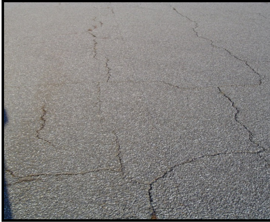
Figure A-10 High-Severity Block Cracking
