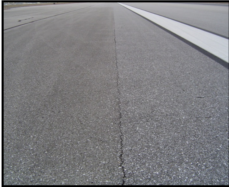
Figure A-25 Medium-Severity L&T Cracking
