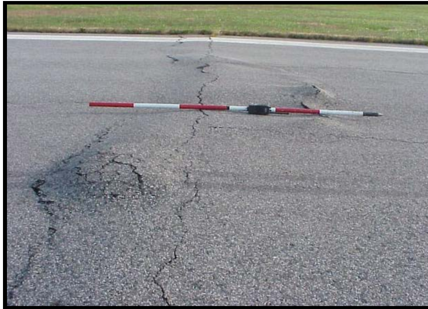
Figure A-53 High-Severity Swell
