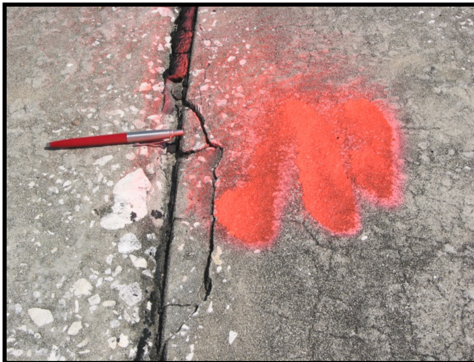
Figure B-38 Medium-Severity Joint Spall
