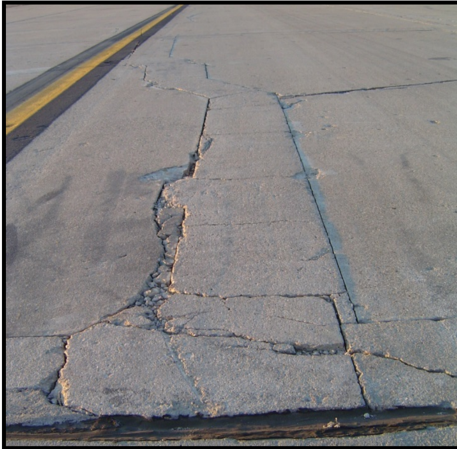
Figure B-23 High Severity Large Patch
