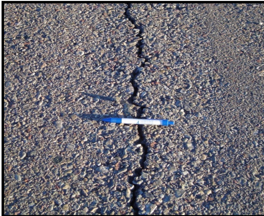
Figure A-25 Medium-Severity L&T Cracking
