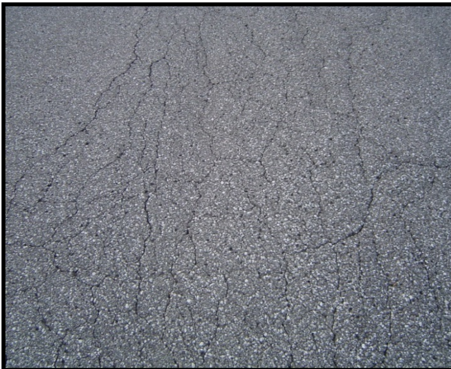
Figure A-2 Medium-Severity Alligator Cracking
