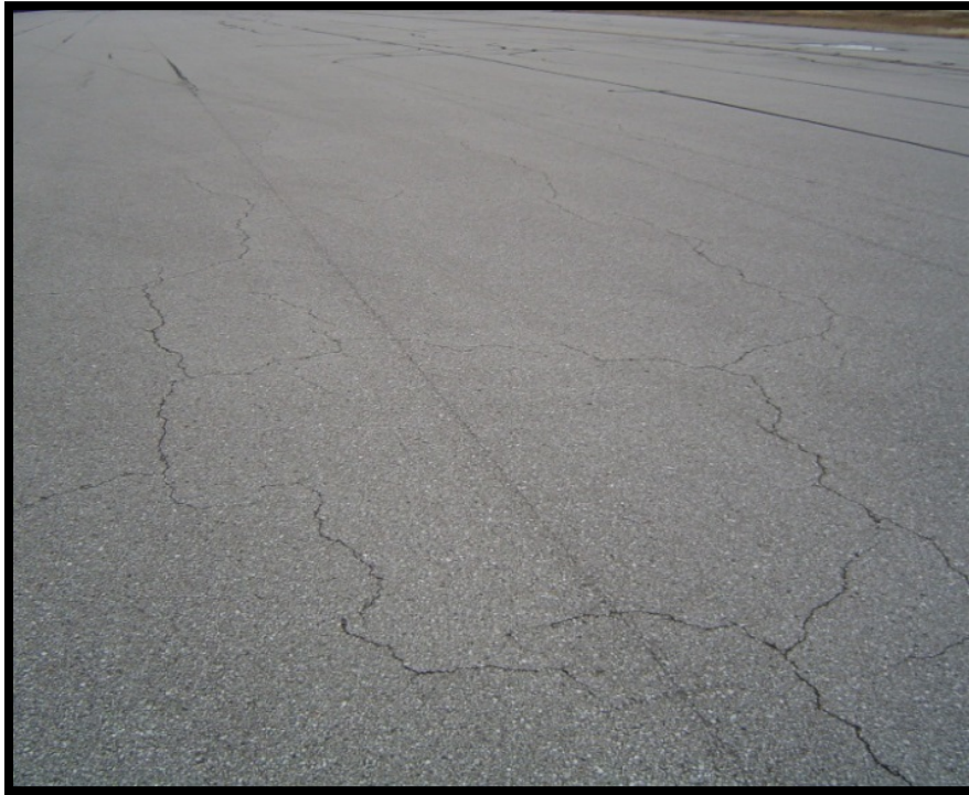
Figure A-8 Medium-Severity Block Cracking
