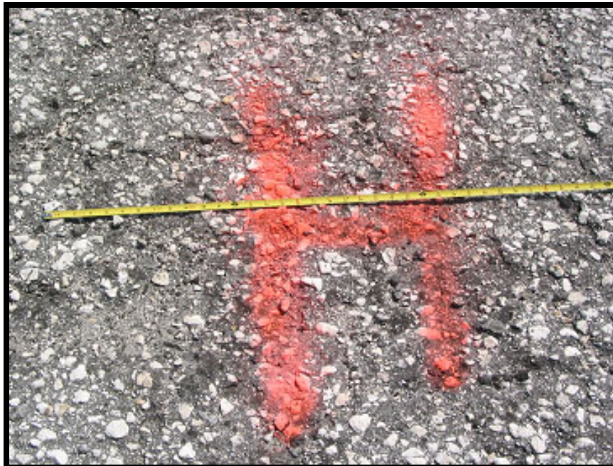
Figure A-38 High-Severity Raveling (Dense Mix)
