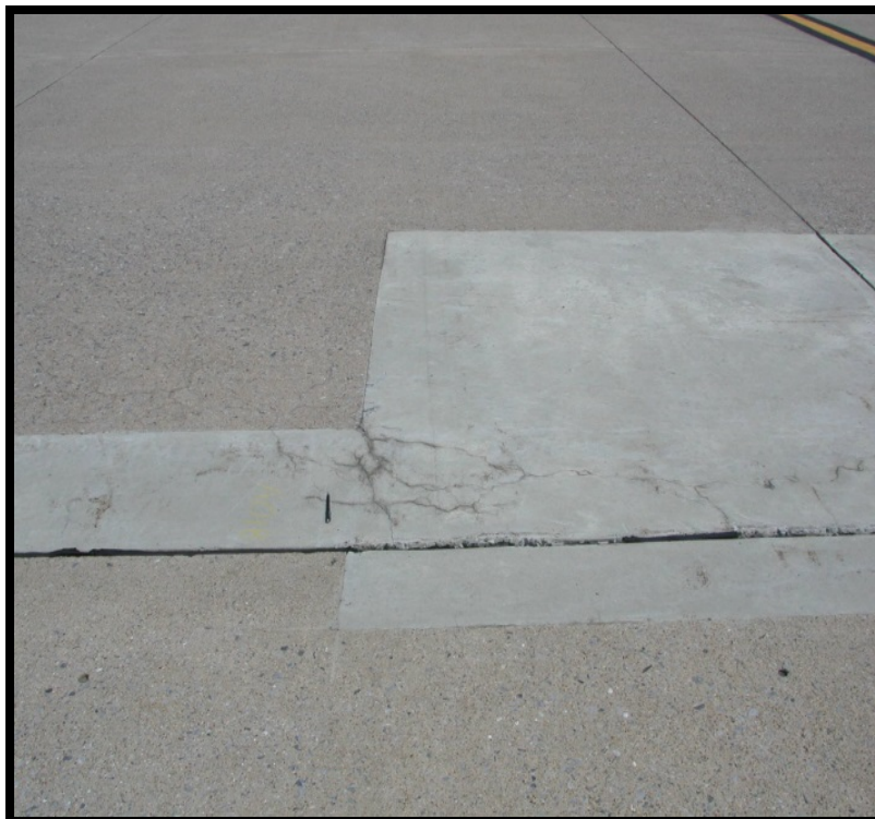
Figure B-22 Medium-Severity Large Patch
