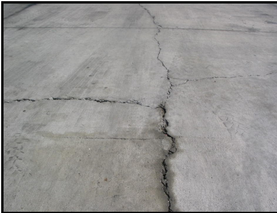
Figure B-35 High-Severity Shattered Slab/Intersecting Cracks
