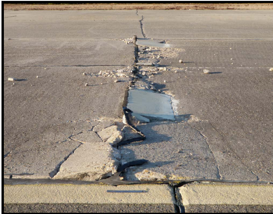
Figure B-4 High-Severity Blowup
