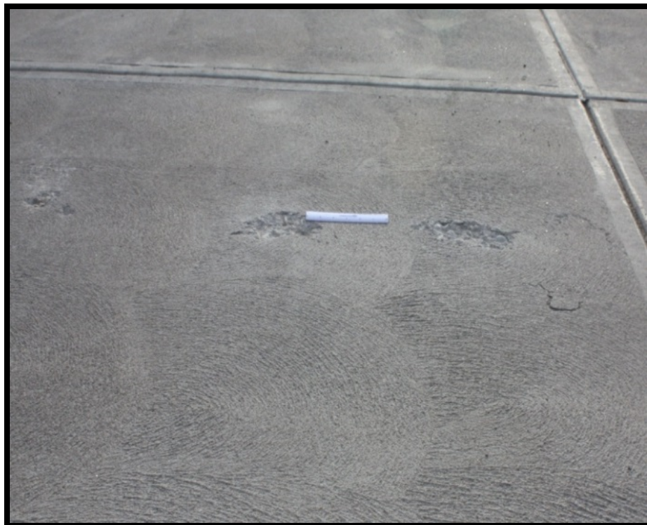
Figure B-28 Medium-Severity Scaling
