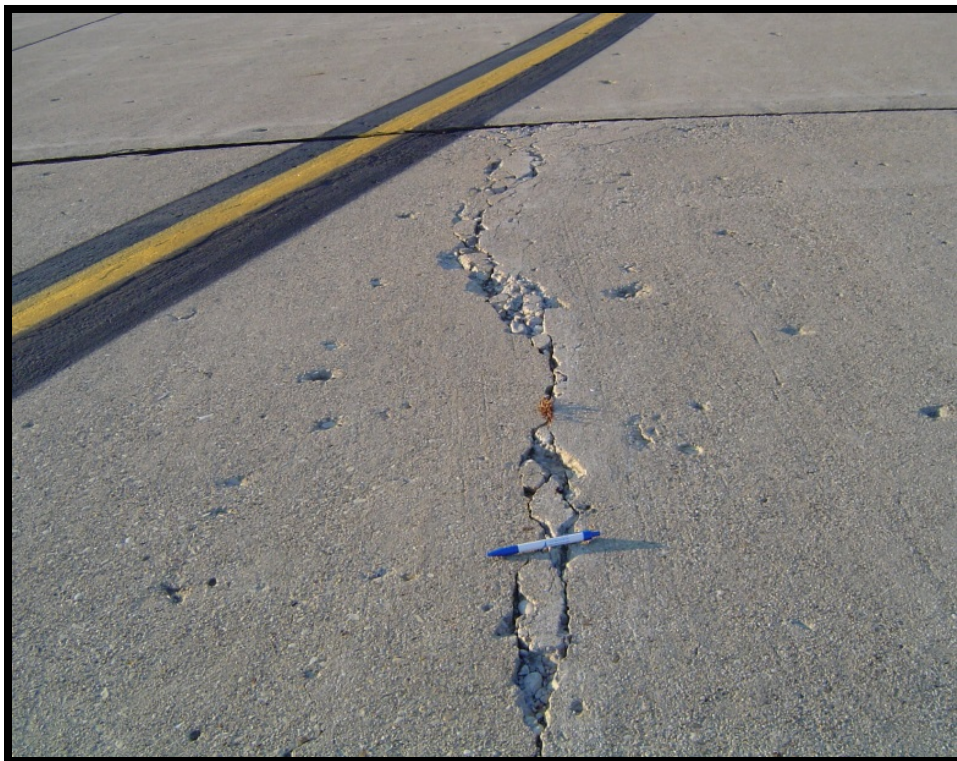
Figure B-10 High-Severity Linear Cracks
