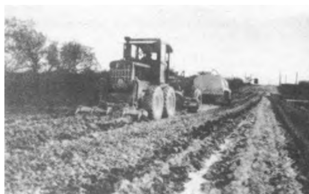
Figure 4-33. Grader-scarifier cutting slurry into stone base.
