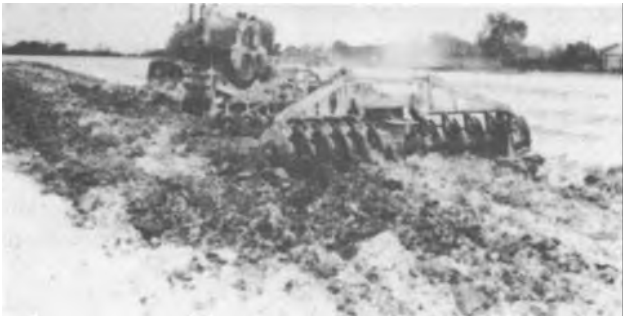
Figure 4-36. Mixing with a disc harrow.
