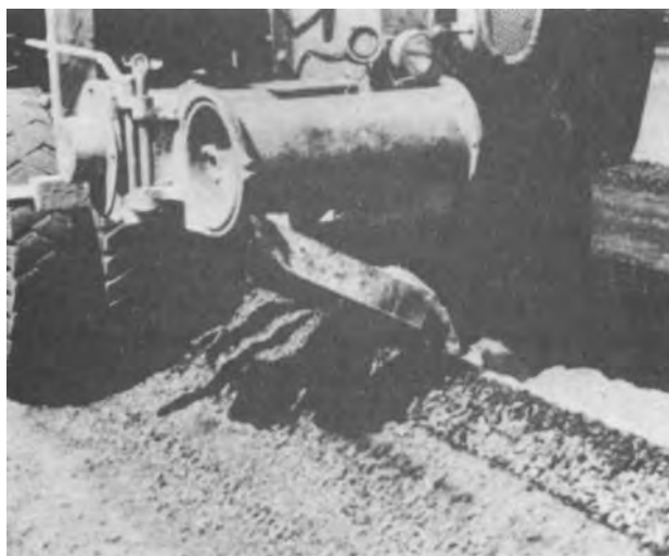
Figure 4-9. Windrow-type mechanical spreader placing cement on windrow.
