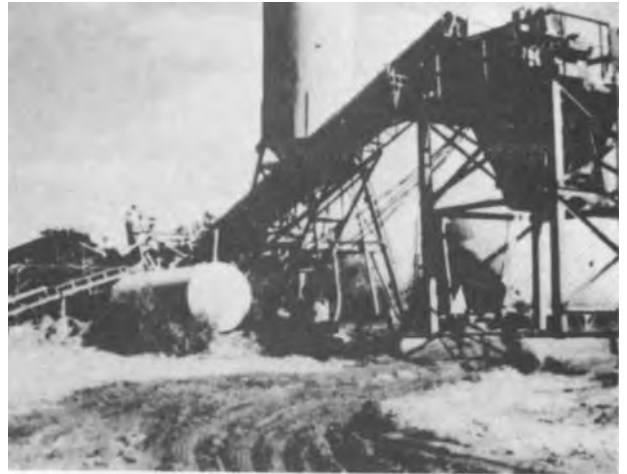
Figure 4-4. Twin-shaft, continuous-flow central mixing plant mixing soil, cement, and water.
