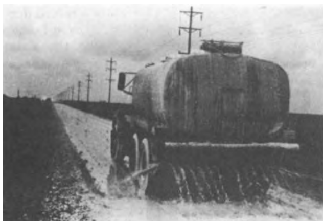
Figure 4-31. Spreading of lime slurry.
