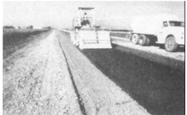
Figure 4-39. Rotary mixer on primary road project.
