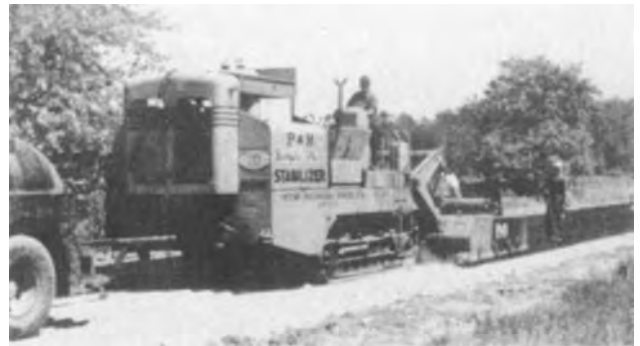
Figure 4-46. Multiple rotary mixer.
