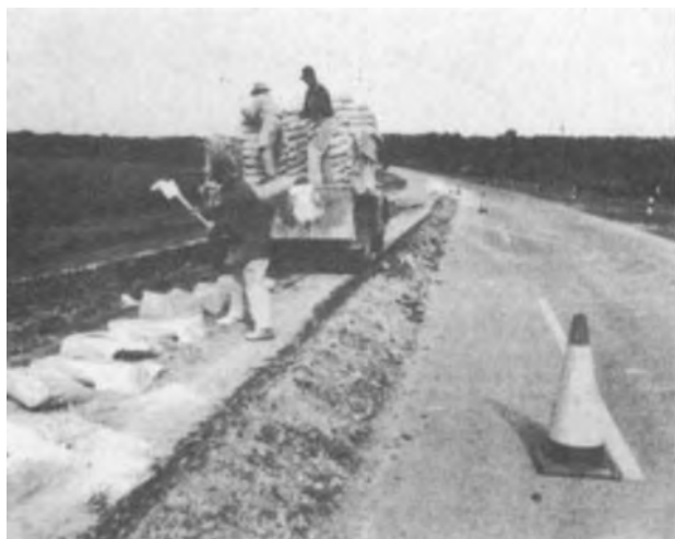
Figure 4-24. Application of lime by the bag for a small maintenance project.
