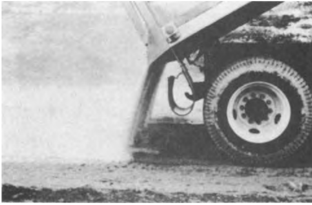
Figure 4-28. Spreading of granular quicklime.
