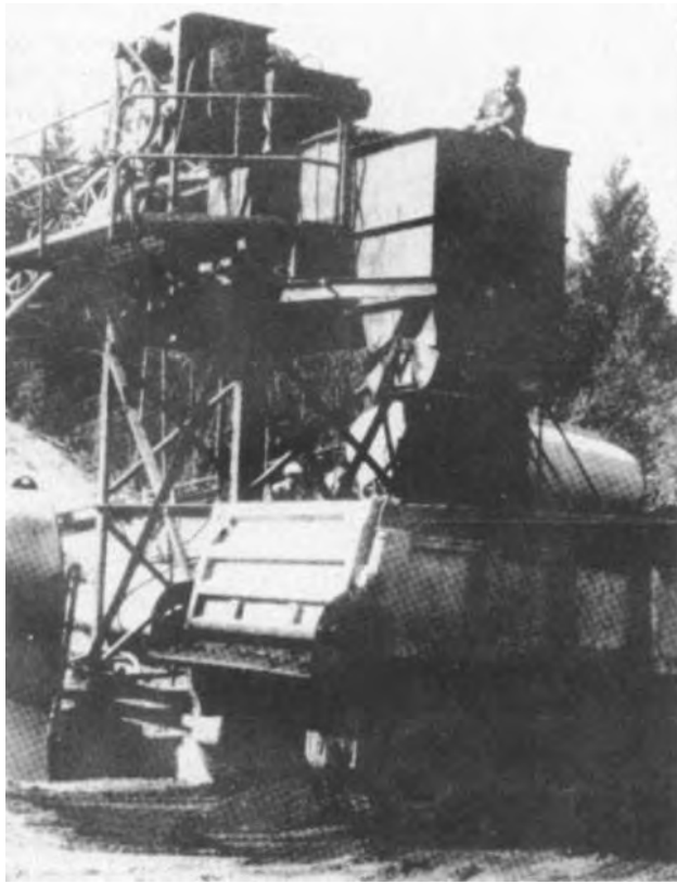
Figure 4-53. Stationary cold-mix plant.
