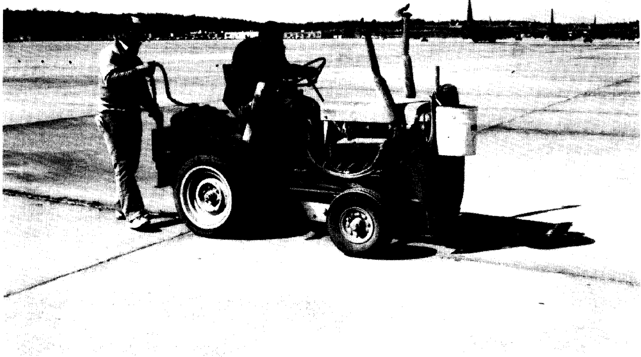
Figure 4-3. Joint Plow Removing Old Sealant.
