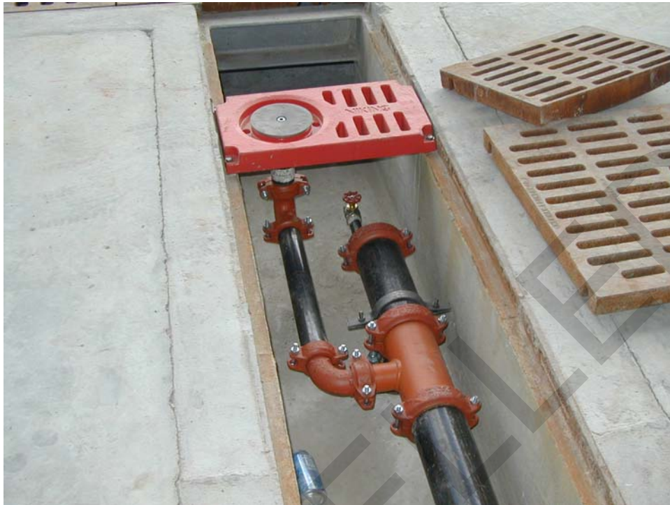
Figure 5-4 Trench Drain Detail
