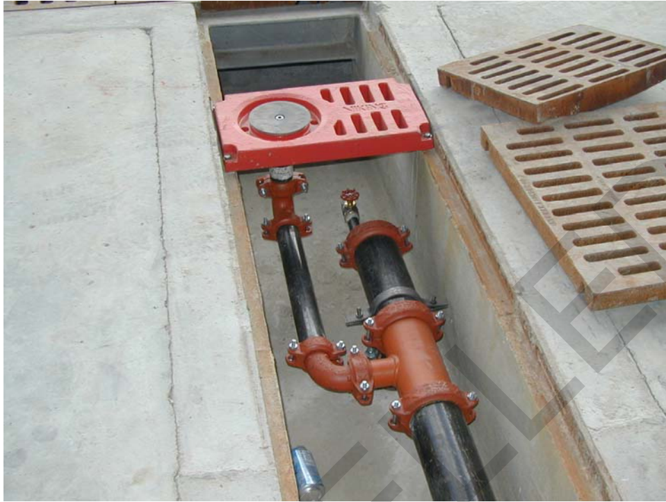
Figure 5-4 Trench Drain Detail
