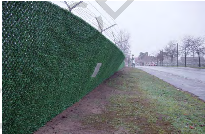
Figure 4-3. Chain Link Fence with Obscuration Material Added
