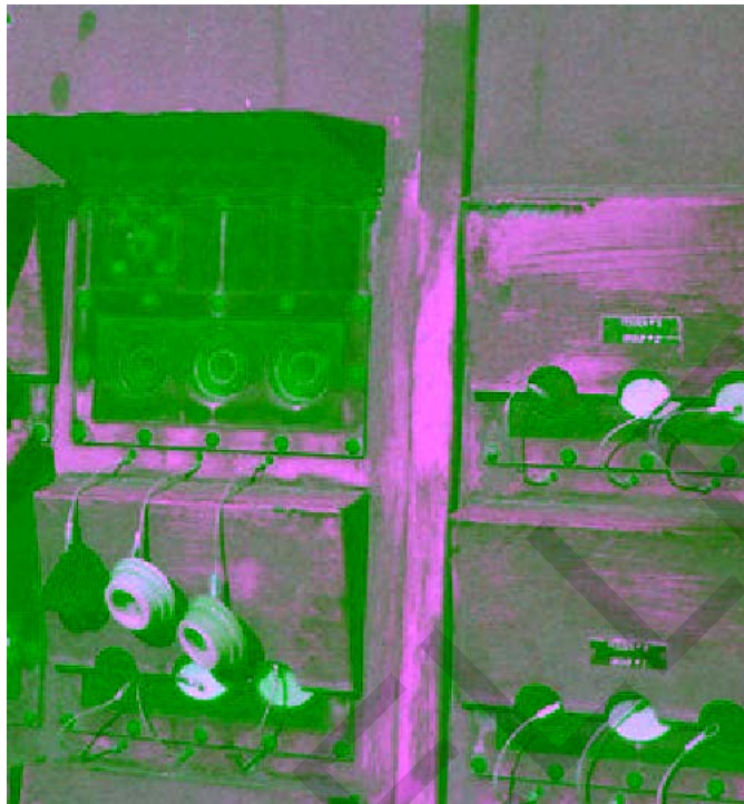
Figure 13-6. Newer Double-Deck Pier Switchgear
