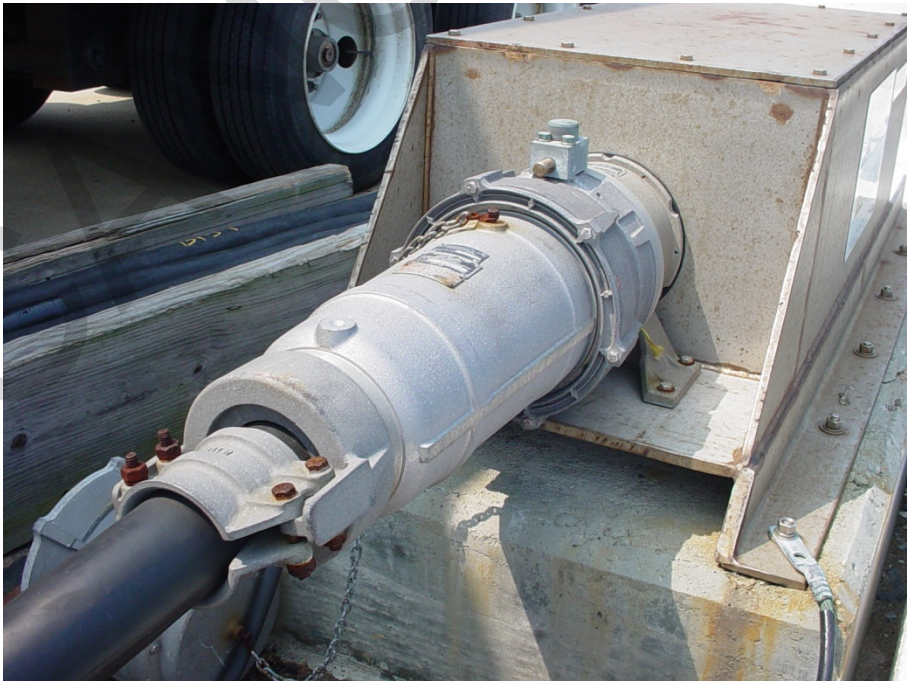
Figure 13-2. Close-Up of Electrical Connection Outlet Assembly
