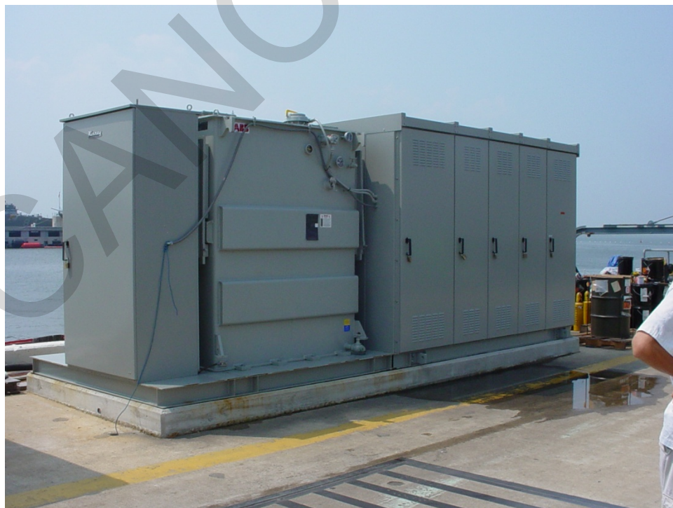
Figure 13-4. Skid-Mounted Substation
