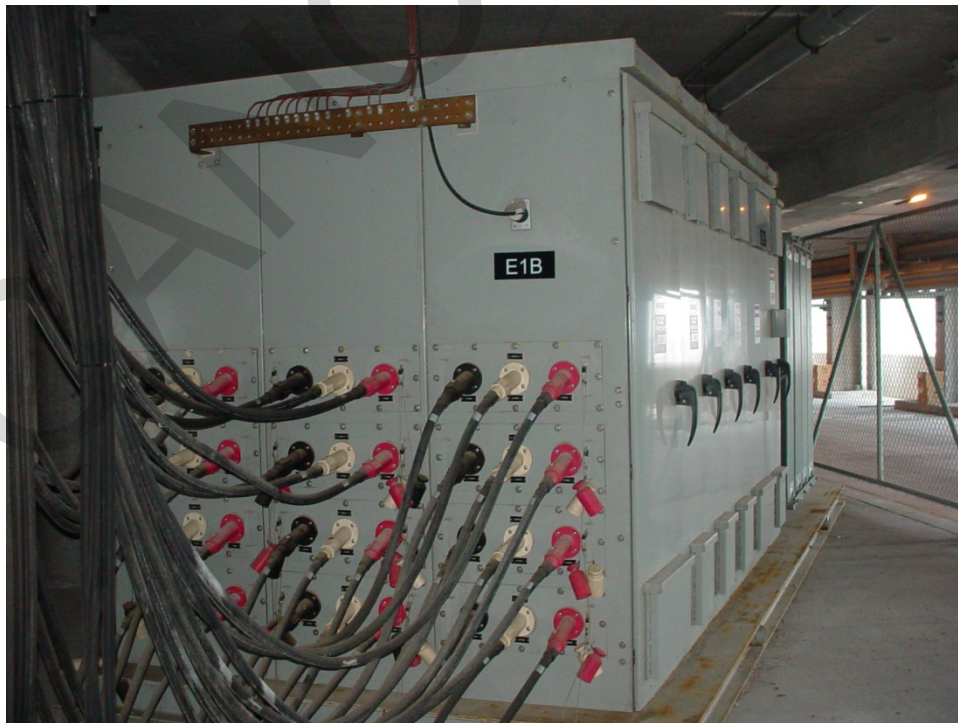
Figure 13-6. Newer Double-Deck Pier Switchgear
