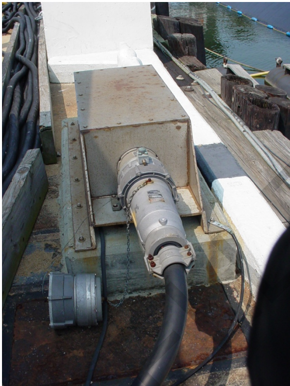
Figure 13-2. Close-Up of Electrical Connection Outlet Assembly
