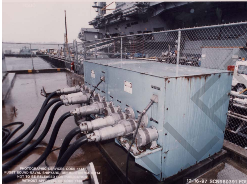
\2\ Figure 13-9. 4.16 kV Pier Electrical Outlet Assembly and Outlets – Newer Designs
