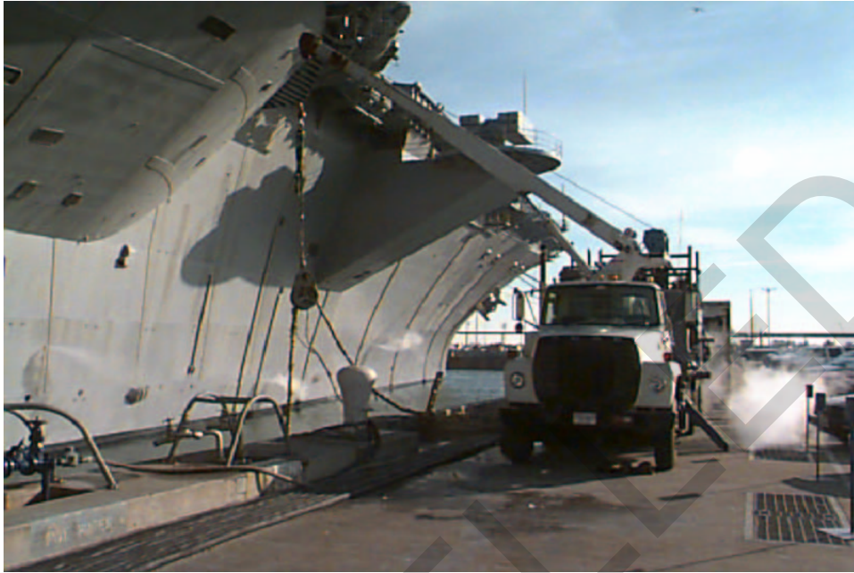
Figure 13-17. Cable Being Reeled by a Boom Truck.
