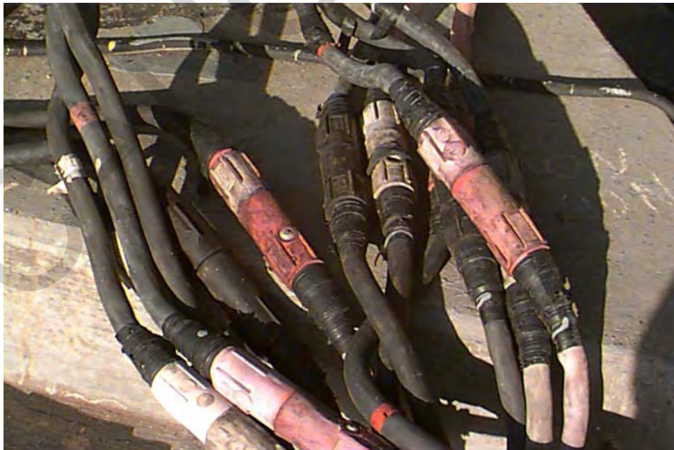
Figure 13-11. 480 Volt Shore-Cable to Ship-Cable with Single-Pole Connection
