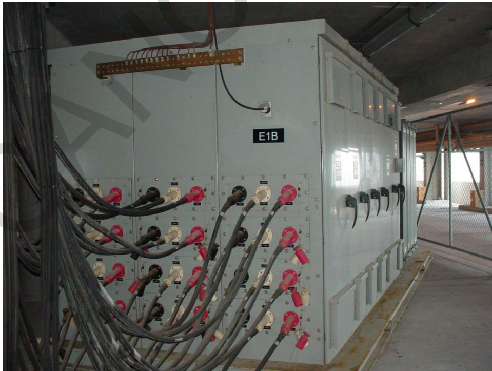
Figure 13-6. Newer Double-Deck Pier Switchgear
