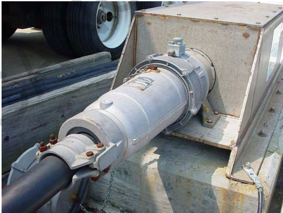
Figure 13-2. Close-Up of Electrical Connection Outlet Assembly
