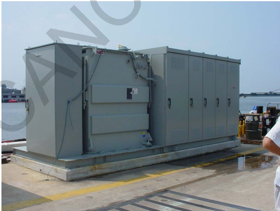
Figure 13-4. Skid-Mounted Substation
