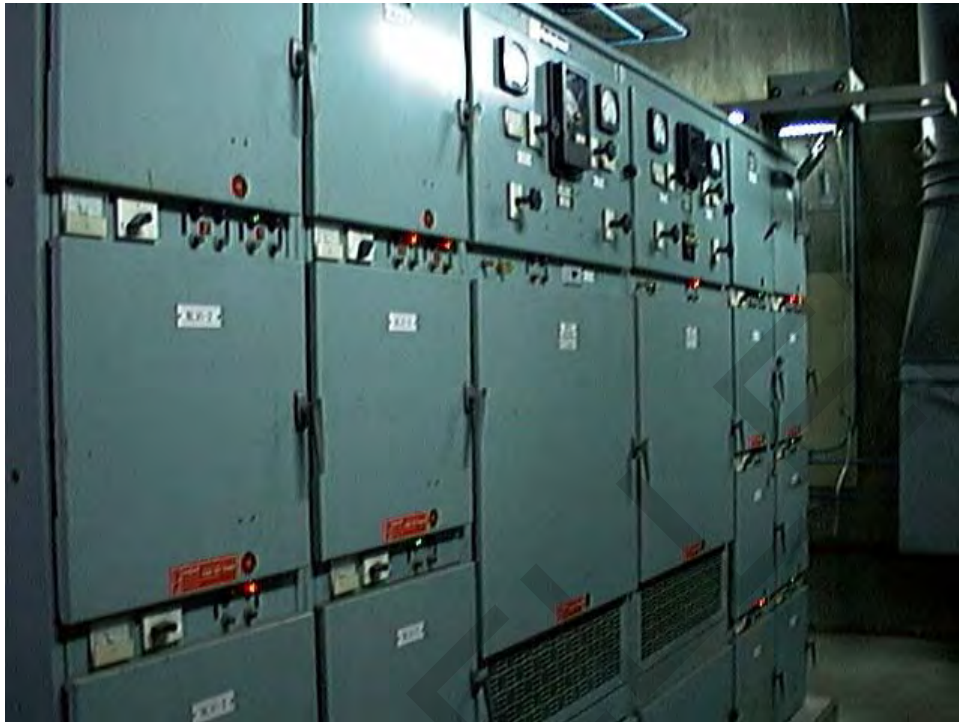
Figure 13-4. Skid-Mounted Substation
