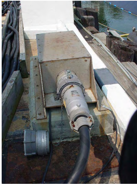
Figure 13-2. Close-Up of Electrical Connection Outlet Assembly
