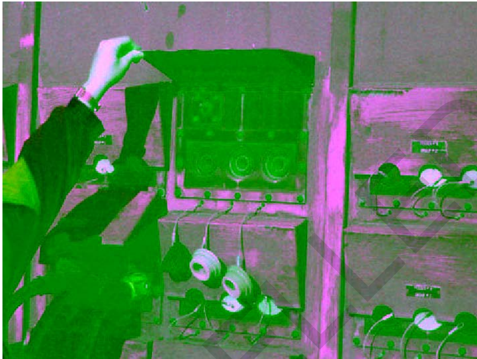
Figure 13-6. Newer Double-Deck Pier Switchgear
