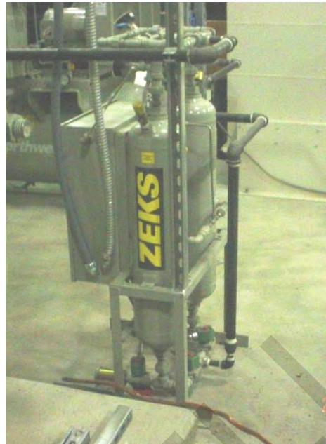
Figure 3.7. Desiccant Air Dryer Assembly
