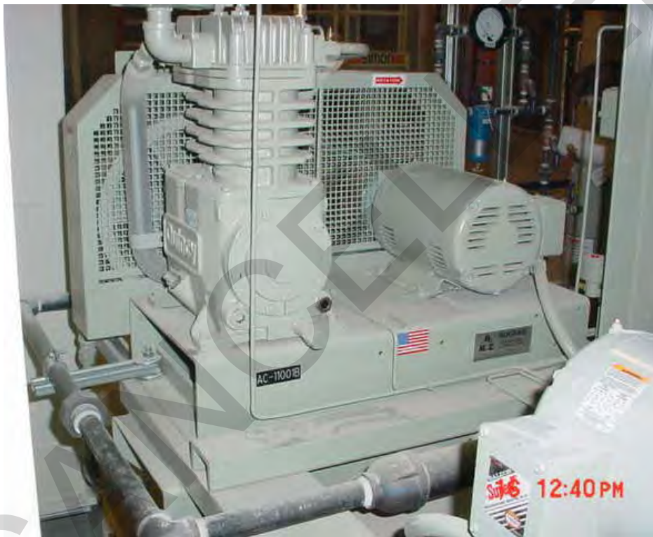
Figure 3-4. One of Two Motor Driven Reciprocating Compressors
