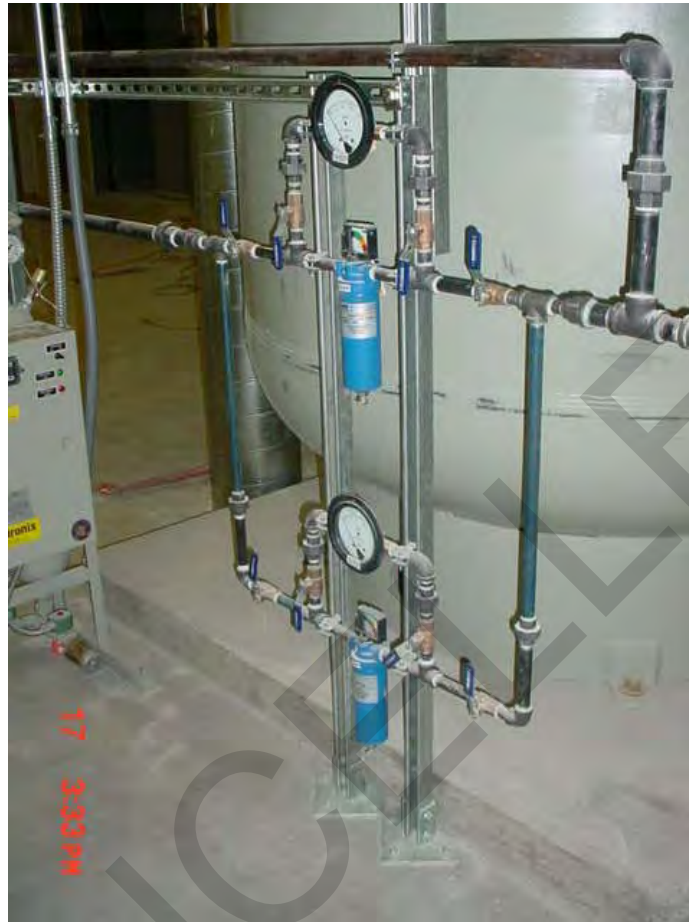
Figure 3.8. Coalescing Air Filters are Line-Mounted
