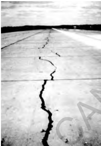
Figure 5.3. Low-severity longitudinal crack
