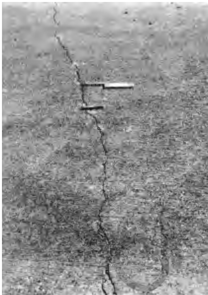
Figure 5.7. Medium-severity transverse crack
