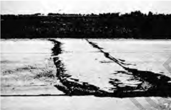
Figure 3.3. Medium-severity blowup
