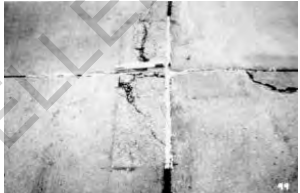
Figure 8.6. High-severity small patch
