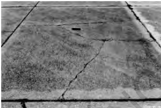
Figure 14.5. Medium-severity intersecting cracks
