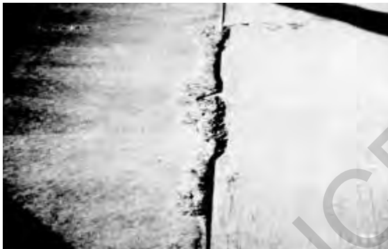
Figure 16.7. High-severity joint spall
