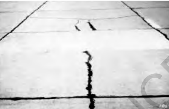
Figure 9.3. Low-severity patch
