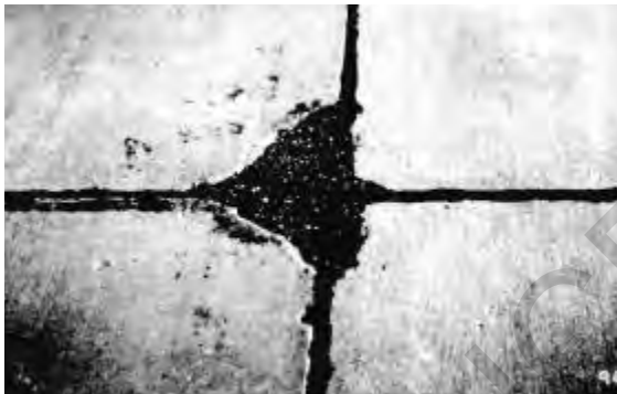
Figure 8.3. Low-severity small patch
