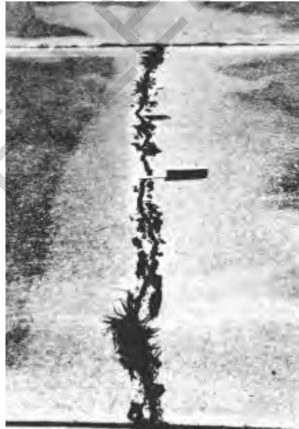
Figure 5.10. High-severity crack
