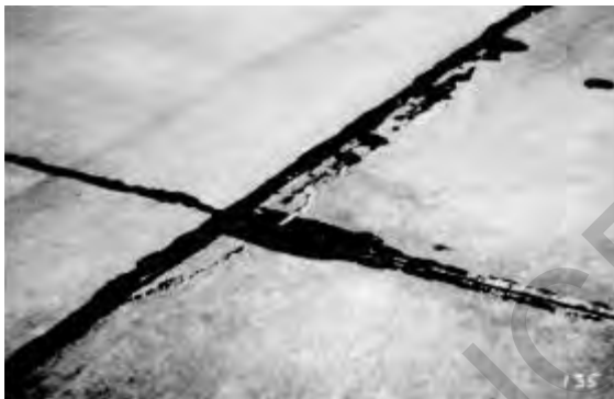
Figure 17.3. Low-severity corner spall
