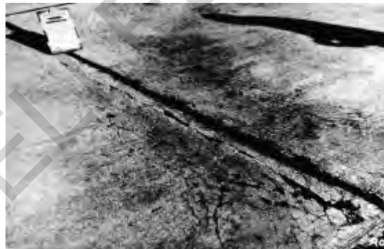
Figure 6.6. High-severity “D” cracking (the “D” cracking occurs over more than one joint with some disintegration)
