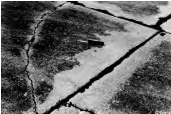
Figure 4.5. Medium-severity corner break
