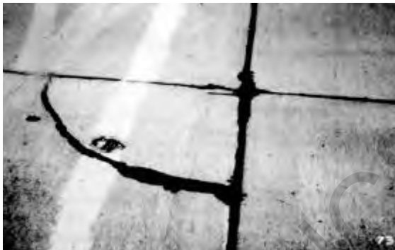
Figure 4.3. Low-severity corner break
