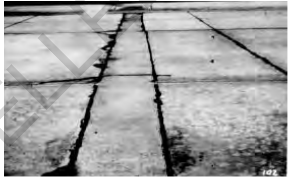
Figure 9.4. Low-severity utility cut
