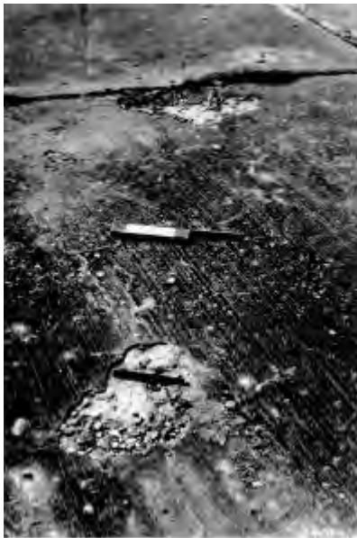
Figure 12.5. Close-up of high-severity scaling
