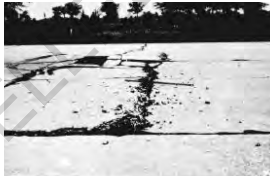
Figure 3.2. Low-severity blowup (note that this would only be considered low severity if the shattering in the foreground were the only part existing and the foreign material were removed)
