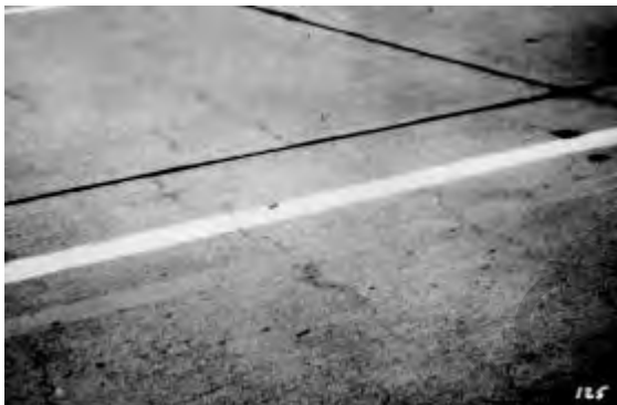
Figure 15.3. Shrinkage cracks
