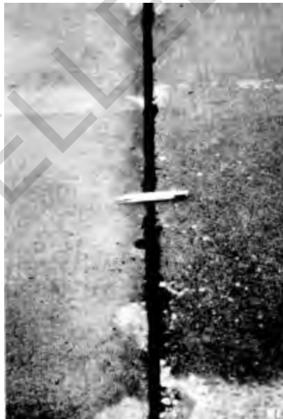
Figure 7.2. Low-severity joint seal damage
