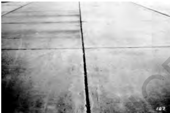
Figure 11.3. Pumping (note stains on pavement)
