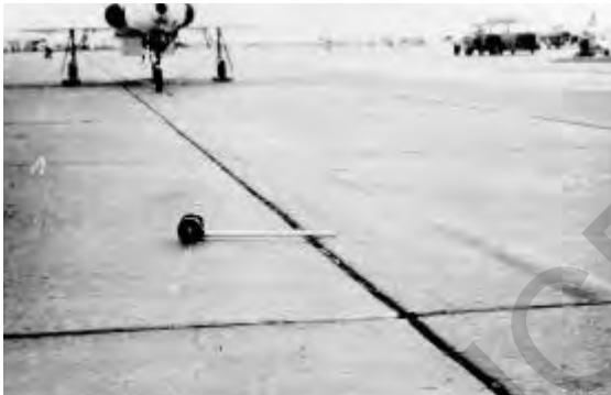
Figure 13.3. Low-severity settlement on apron
