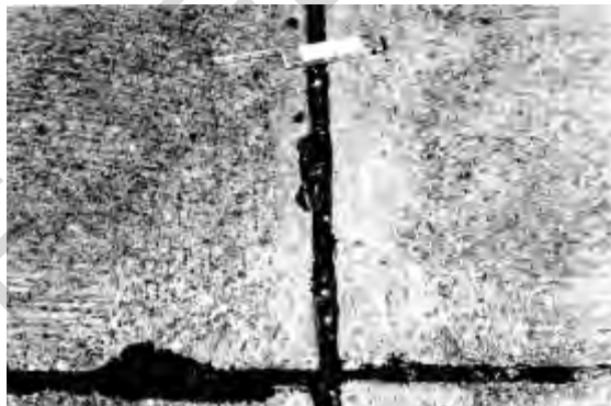
Figure 7.4. High-severity joint seal damage (complete loss of sealant; joint is filled with incompressible material)
