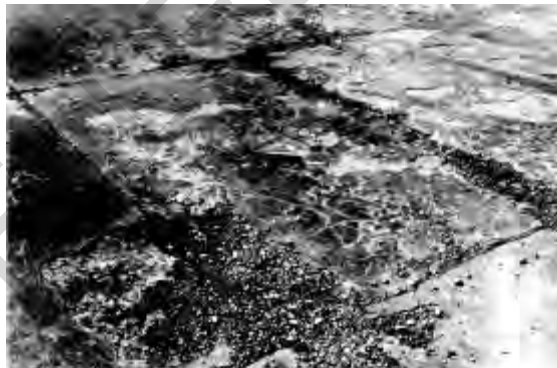
Figure 12.4. High-severity scaling
