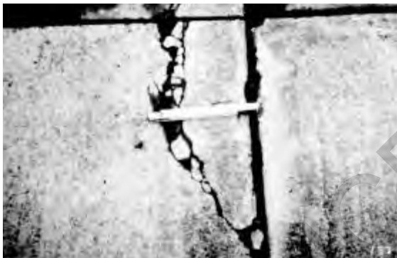
Figure 17.5. Medium-severity corner spall
