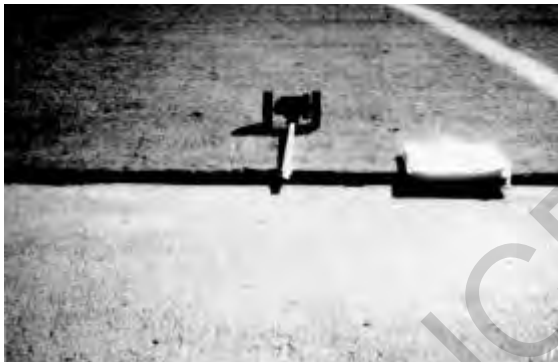
Figure 13.5. High-severity settlement on taxiway/runway, 3/4 in. (19.1 mm)
