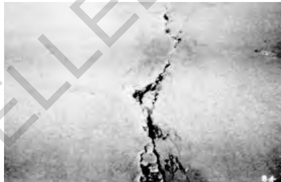
Figure 5.8. High-severity crack
