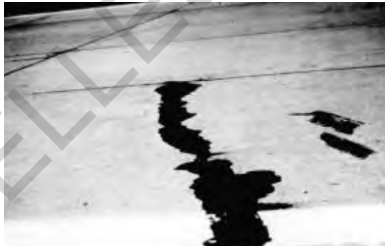
Figure 5.6. Medium-severity transverse crack
