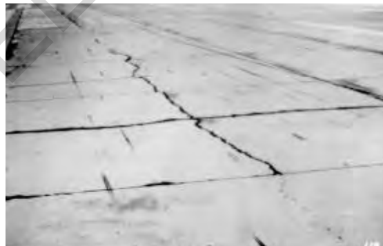
Figure 14.2. Low-severity intersecting cracks
