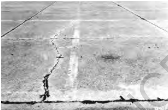
Figure 5.5. Medium-severity longitudinal crack
