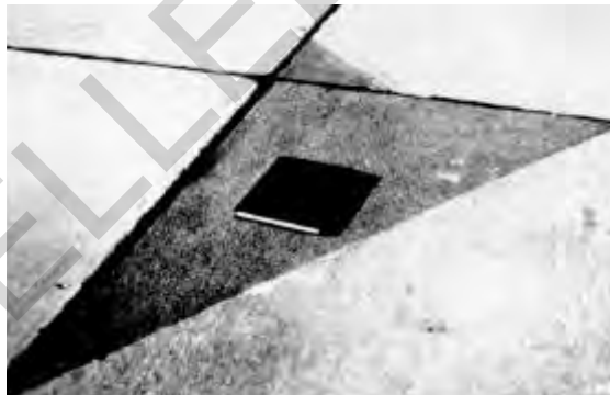
Figure 9.2. Low-severity patch
