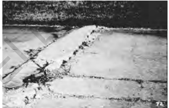
Figure 3.4. High-severity blowup
