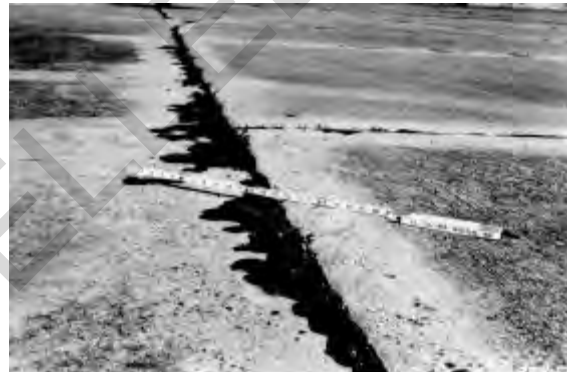
Figure 13.4. Medium-severity settlement on apron >1/2 in. (>12.7 mm)
