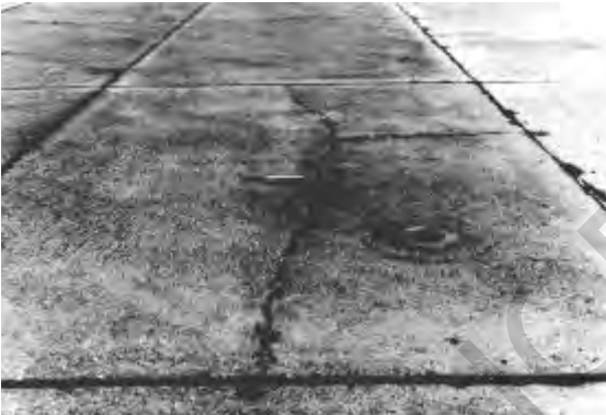
Figure 5.9. High-severity longitudinal cracks
