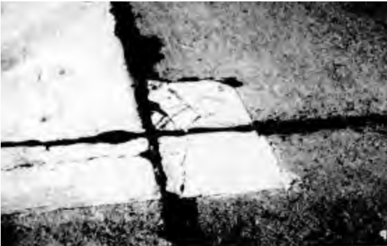
Figure 8.5. Medium-severity small patch
