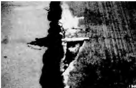
Figure 16.5. Medium-severity joint spall
