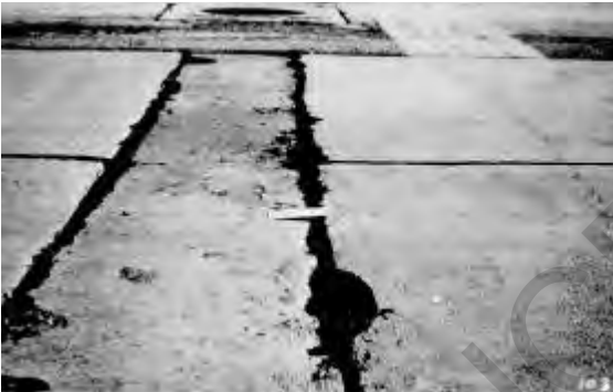
Figure 9.5. Medium-severity utility cut
