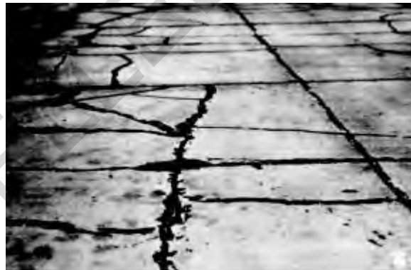
Figure 14.6. Shattered slab
