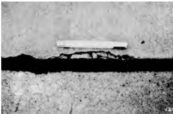
Figure 16.3. Low-severity joint spall
