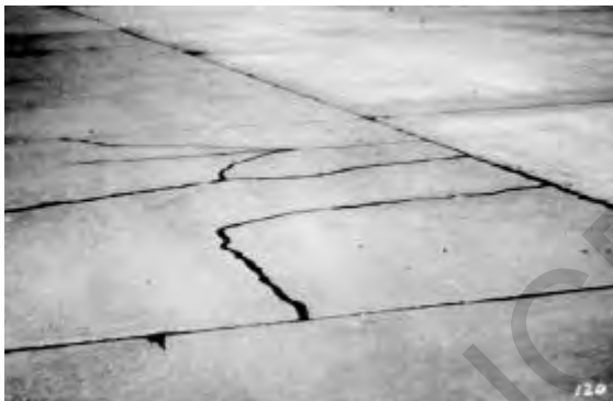
Figure 14.3. Low-severity intersecting cracks
