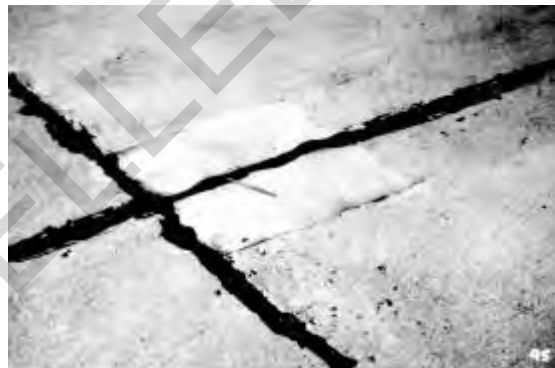
Figure 8.2. Low-severity small patch
