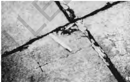
Figure 8.4. Medium-severity small patch
