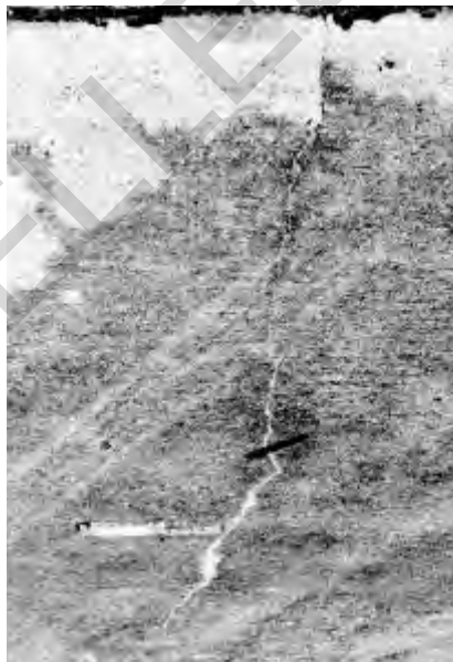
Figure 5.2. Low-severity longitudinal crack
