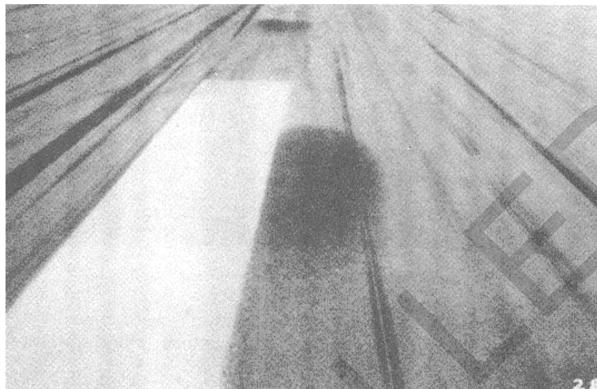
Figure A-21. Jet blast erosion, case 1.
