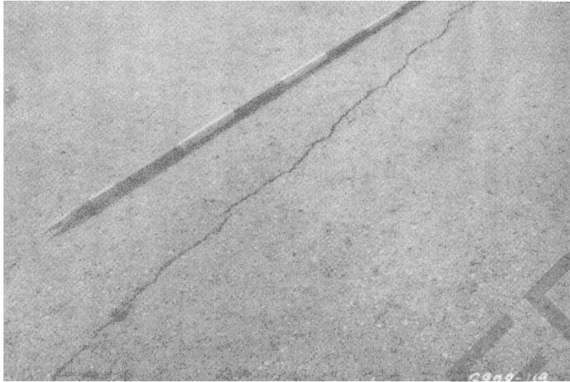
Figure A-31. Medium severity longitudinal crack, case 2.
