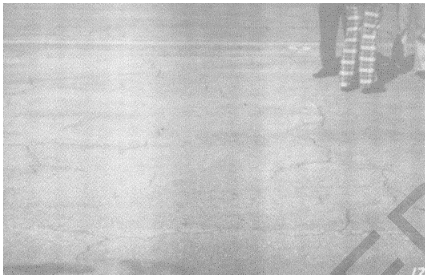
Figure A-10. Low severity block cracking, case 3.
