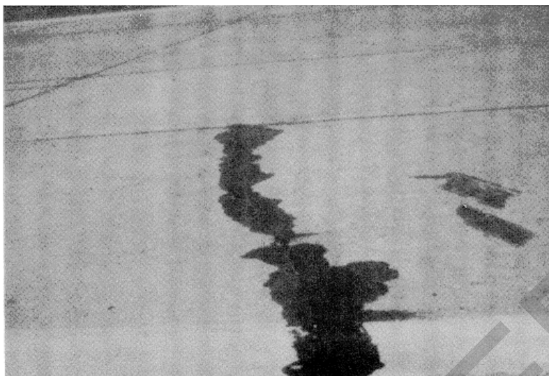
Figure A-79. Medium severity transverse crack, case 2.
