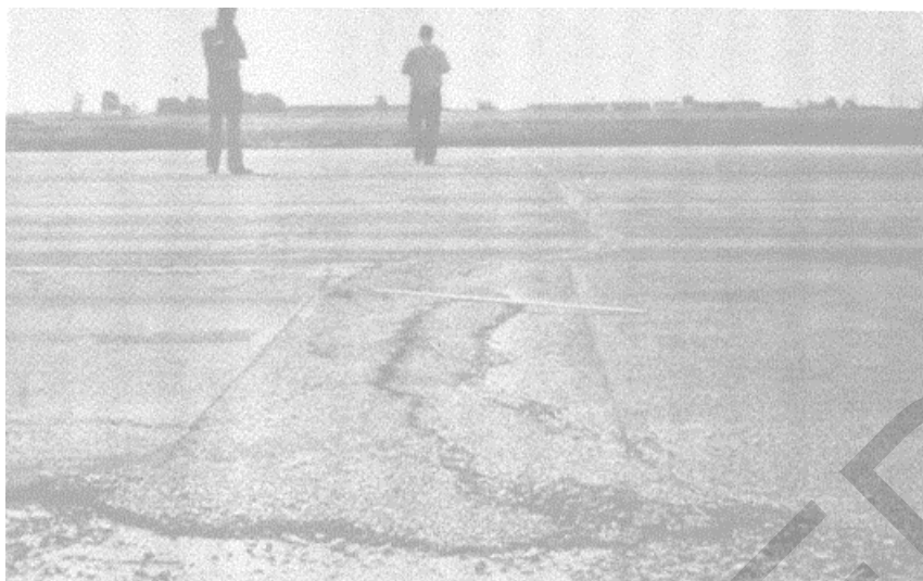
Figure A-65. High severity swell.
