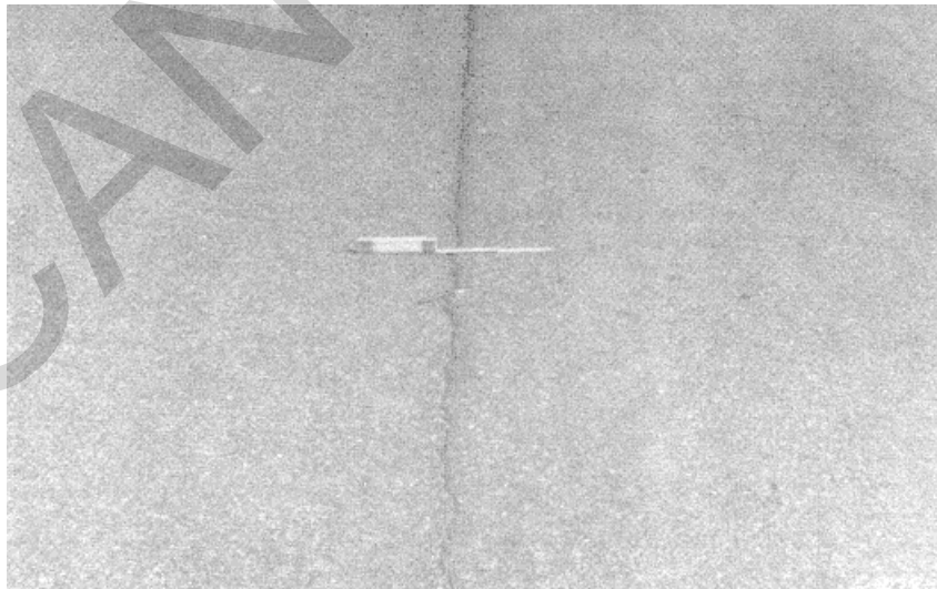
Figure A-30. Medium severity longitudinal construction joint crack, case 1.
