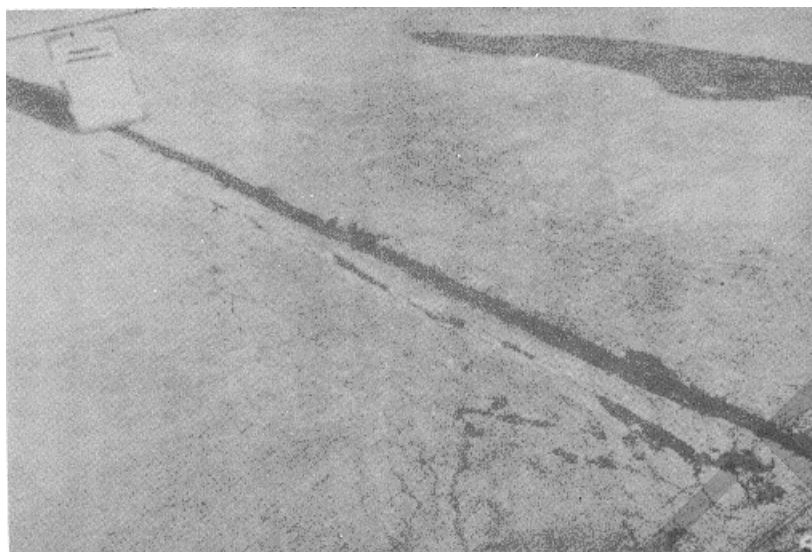
Figure A-86. High severity D cracking.
