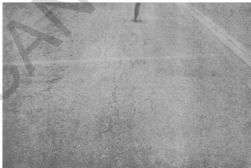
Figure A-2. Low severity alligator cracking, case 2.
