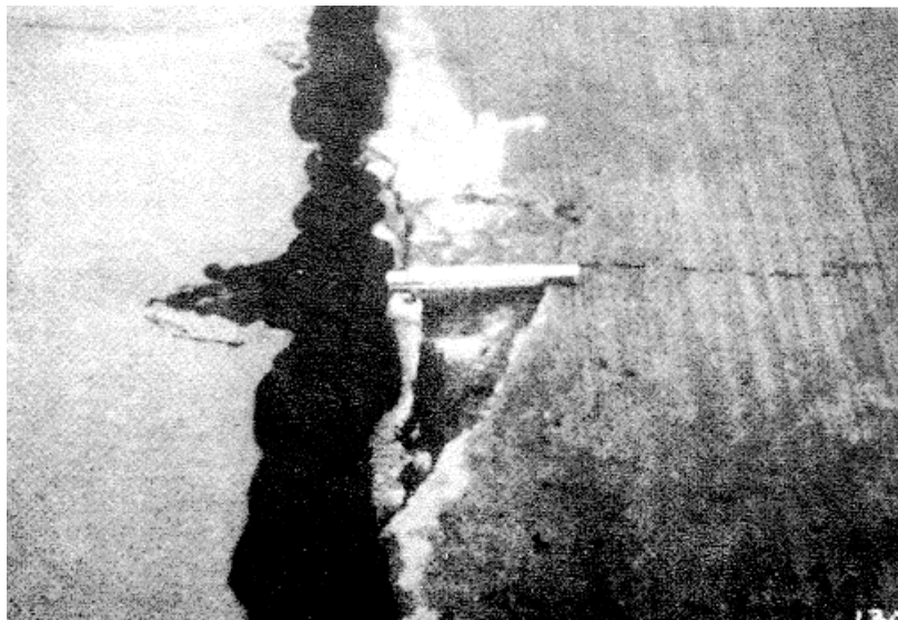
Figure A-126. Medium severity joint spay case 1.
