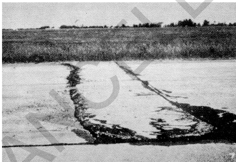
Figure A-67. Medium severity blowup
