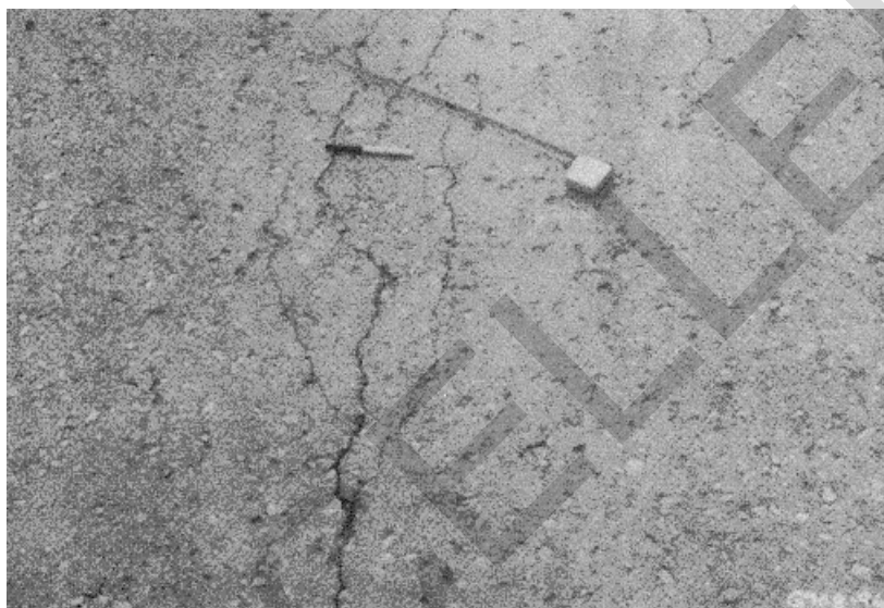
Figure A-1. Low severity alligator cracking, case 1.
