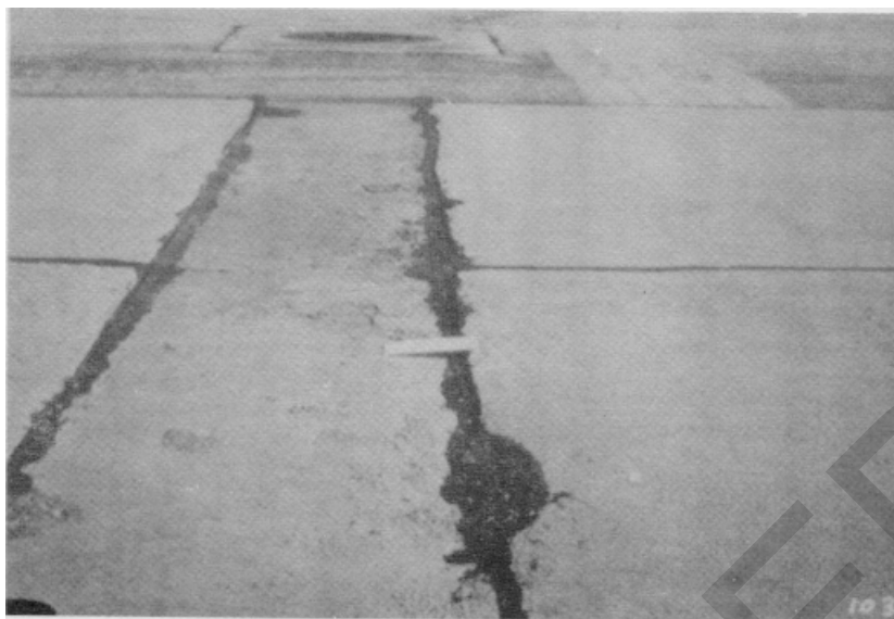
Figure A-99. Medium severity utility cut.
