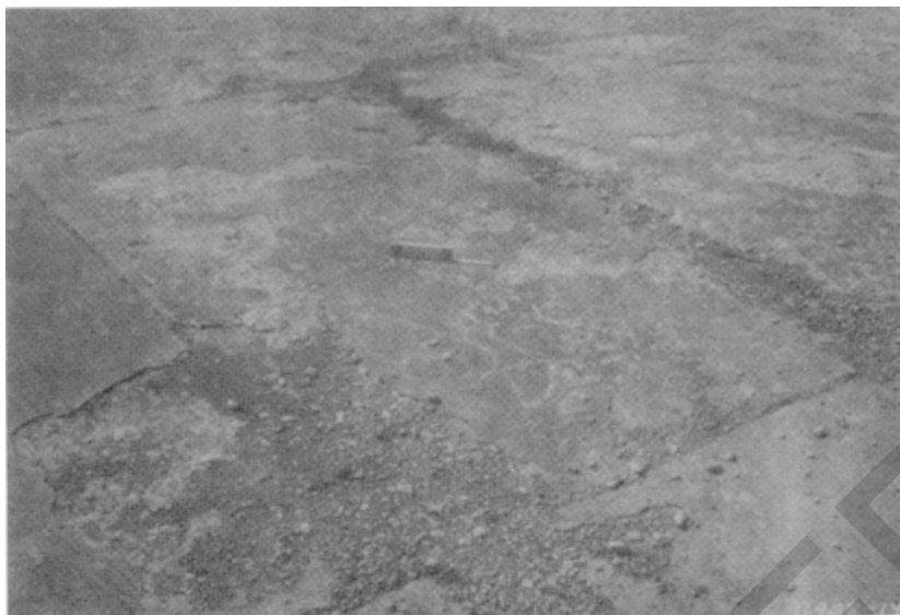
Figure A-109. High severity scaling.
