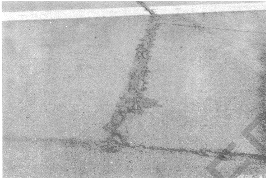
Figure A-26. High severity joint reflection cracking.
