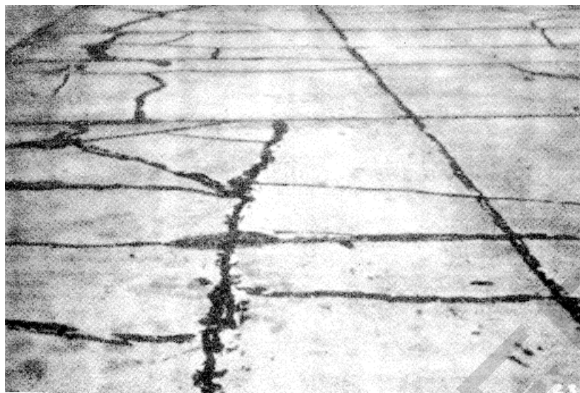
Figure A-121. Shattered slab.
