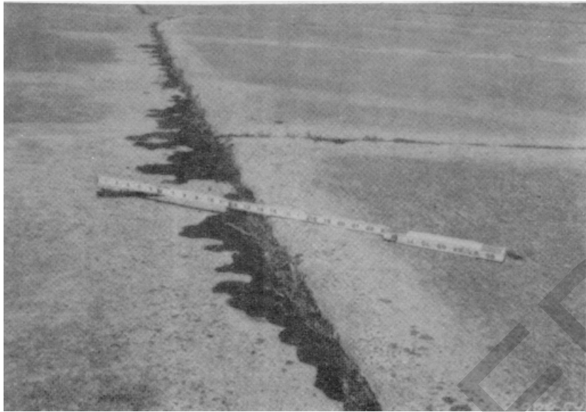
Figure A-113. Medium severity settlement on apron.
