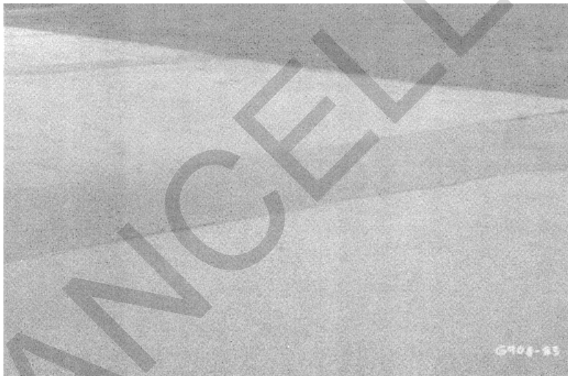
Figure A-38. Low severity patch, case 2.
