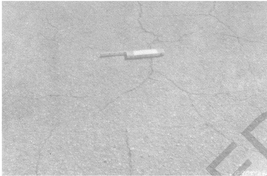
Figure A-8. Low severity block cracking, case 1.
