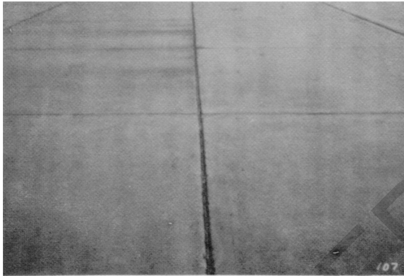
Figure A-103. Pumping (note stained pavement).
