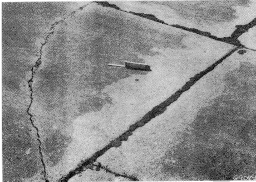
Figure A-72. Medium severity corner break, case 2.
