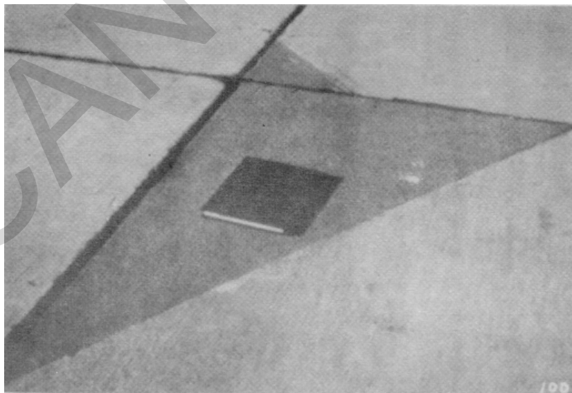
Figure A-96. Low severity patch, case 1.
