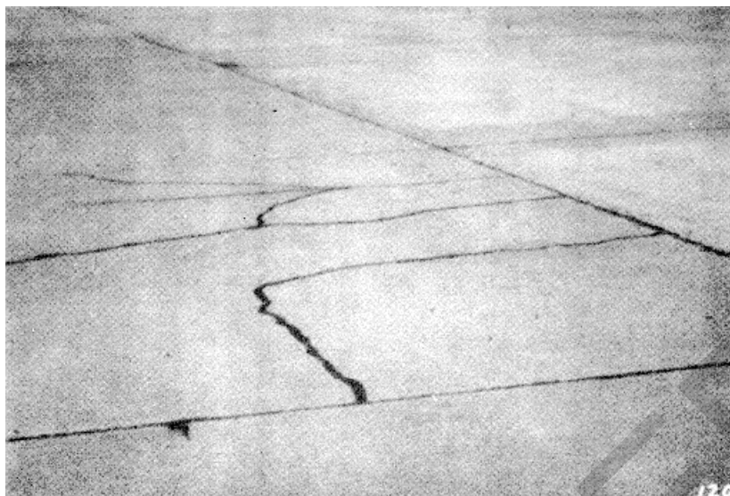
Figure A-117. Low severity intersecting cracks, case 1.
