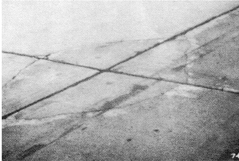
Figure A-70. Low severity corner break, case 2.
