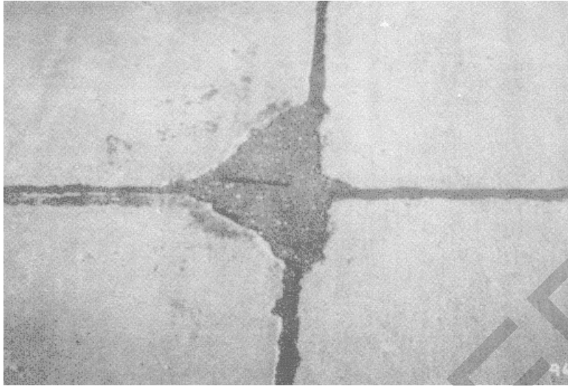
Figure A-91. Low severity small patch, case 1.
