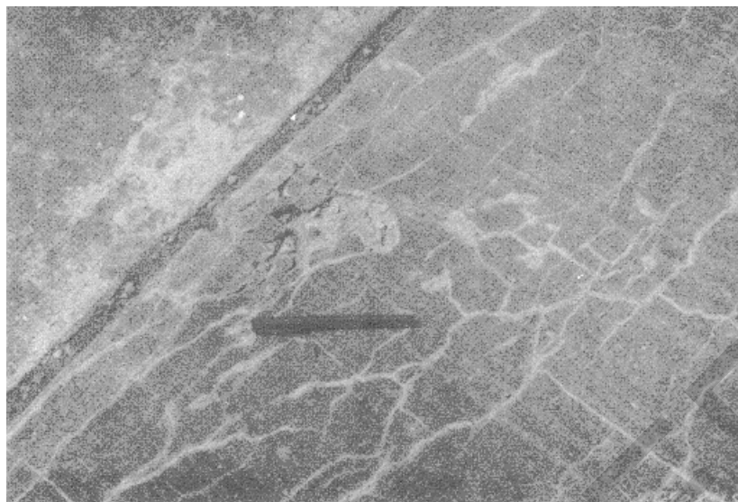
Figure A-84. Medium severity D cracking case 1.
