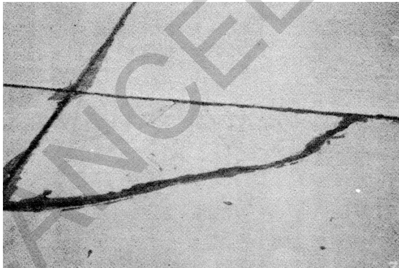
Figure A-71. Medium severity corner break, case 1.
