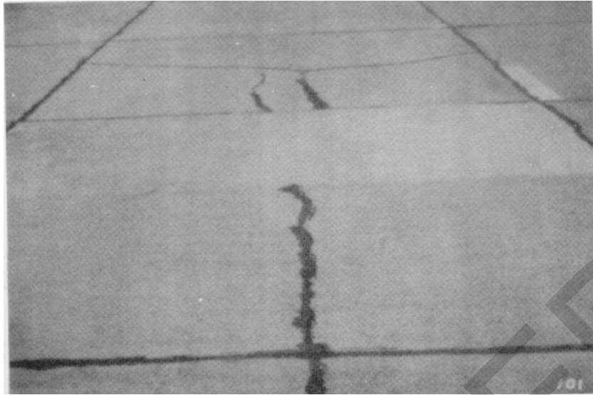
Figure A-97. Low severity patch, case 2.
