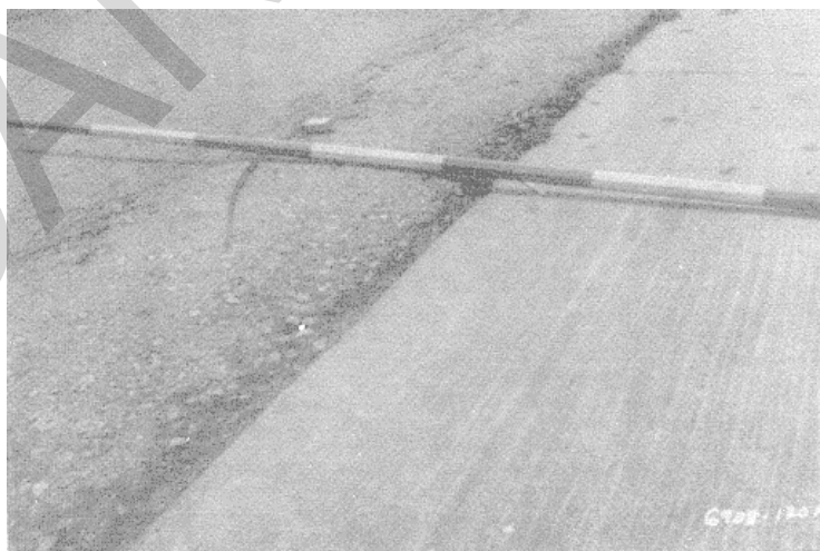
Figure A-59. High severity shoving.
