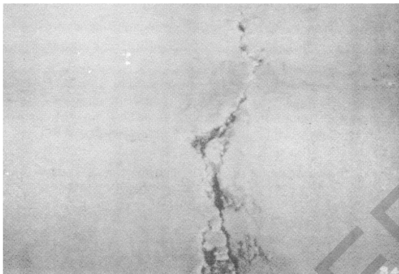
Figure A-81. High severity longitudinal crack, case 1.
