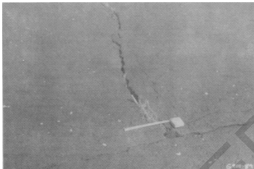
Figure A-33. High severity longitudinal crack.
