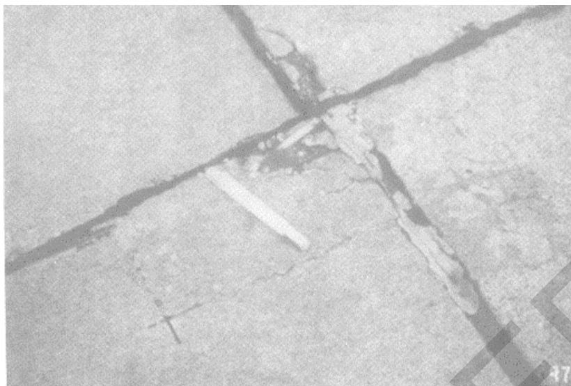
Figure A-93. Medium severity small patch case 1.
