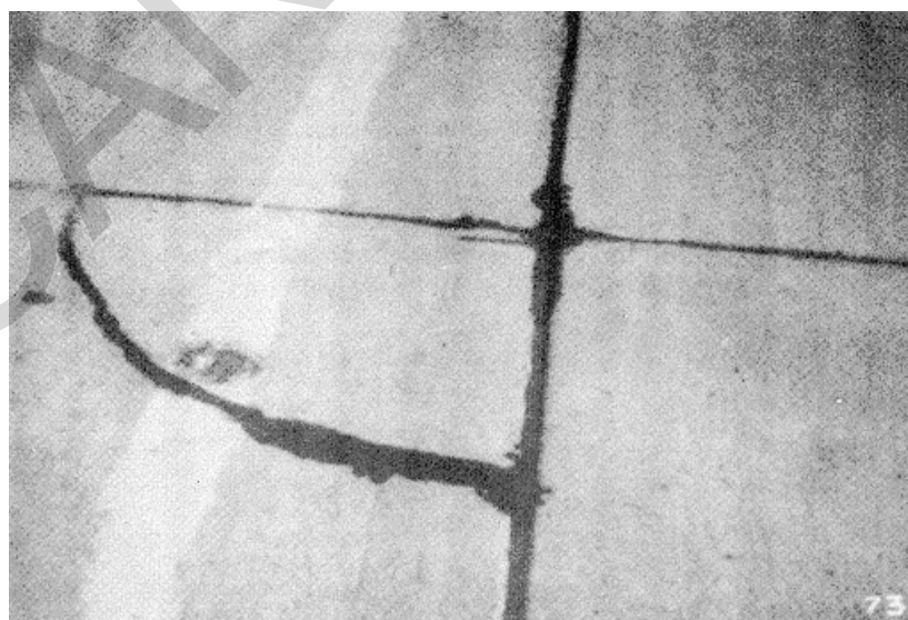
Figure A-69. Low severity corner break, case 1.
