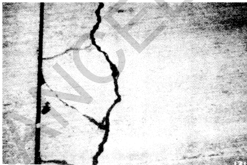
Figure A-127. Medium severity joint spay case 2
