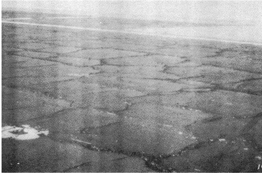
Figure A-14. High severity block cracking case 2.
