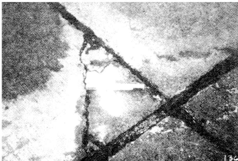
Figure A-132. Medium severity corner spay case 1
