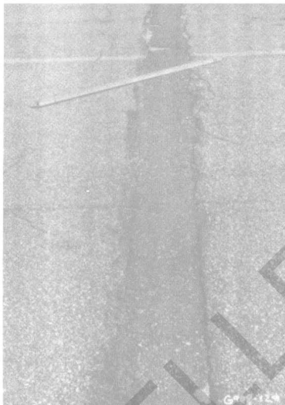
Figure A-39. Medium severity patch.
