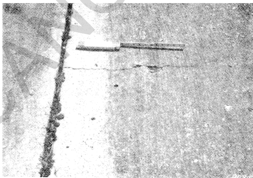
Figure A-122. Shrinkage crack, case 1
