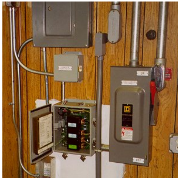
Figure 9 Less-Than-Optimal Installation by Including Safety Switch
