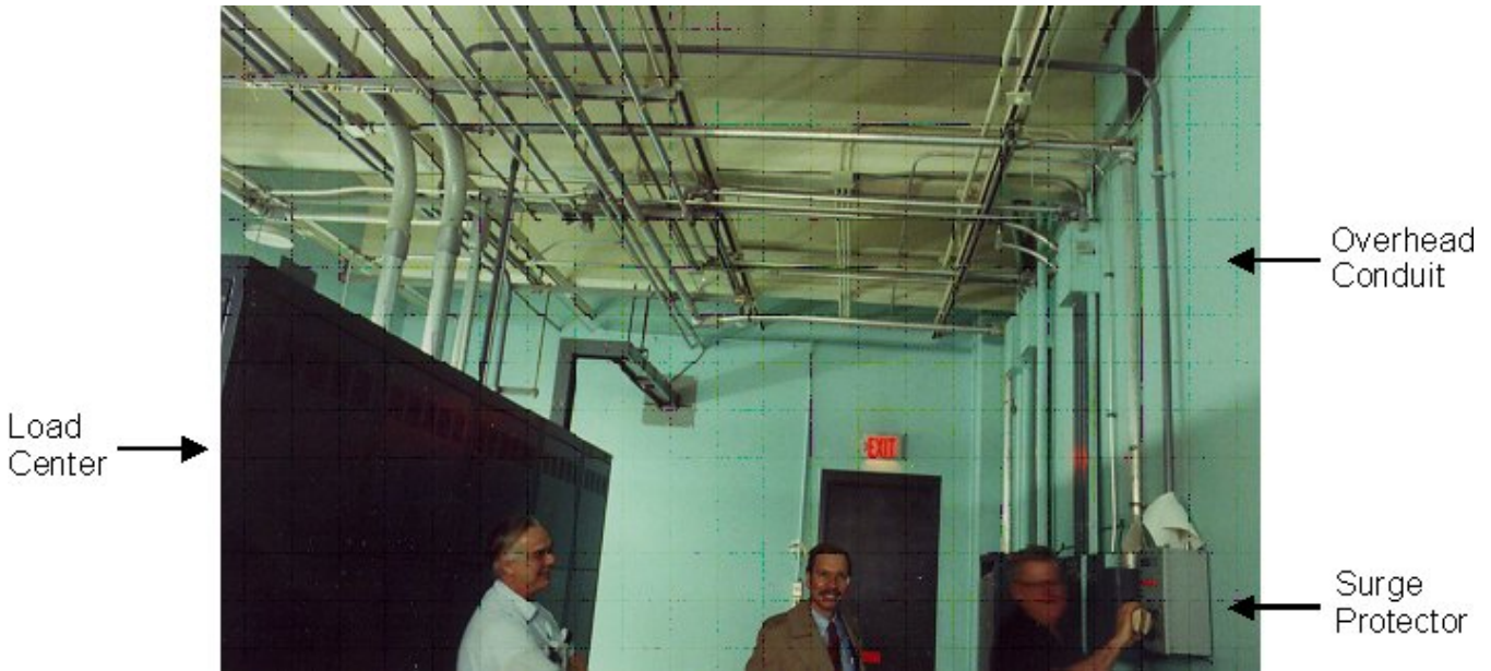
Figure 9 Less-Than-Optimal Installation by Including Safety Switch
