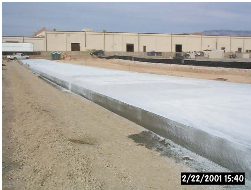
Figure 4-116 Poor Application of Curing Compound Vertical Joint
