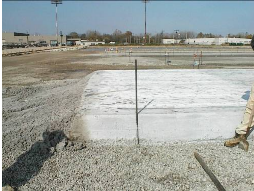
Figure 4-128 Paving Through and Sawing Off End
