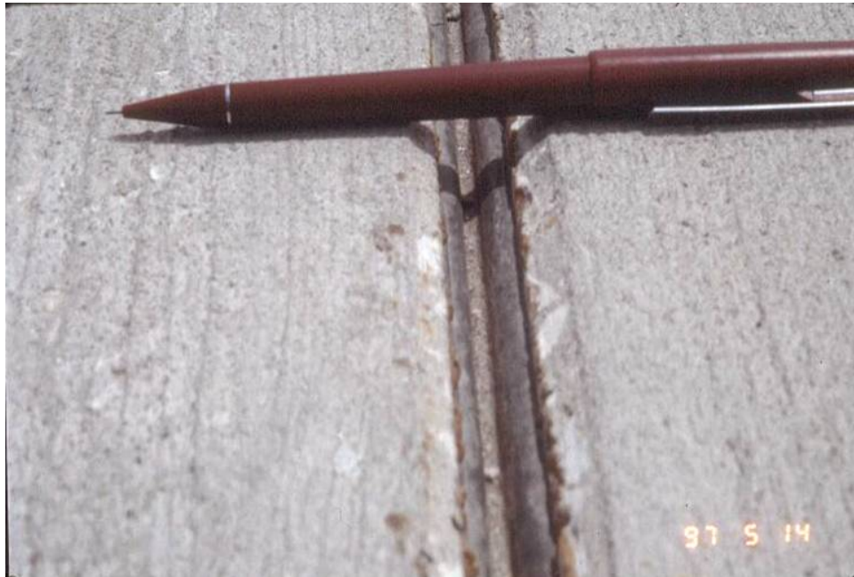
Figure 4-149 Chamfered and Sealed Joint
