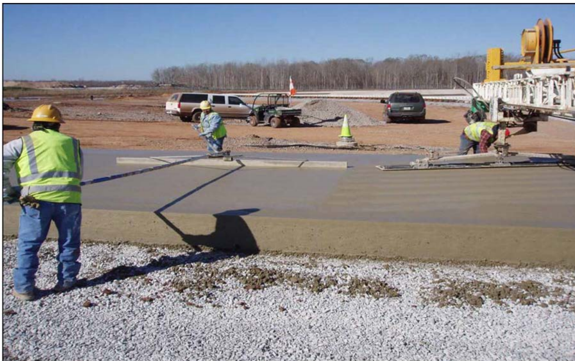
Figure 4-106 Cutting Straightedge
