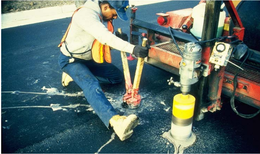
Figure 3-48 Cutting Cores for Density Testing
