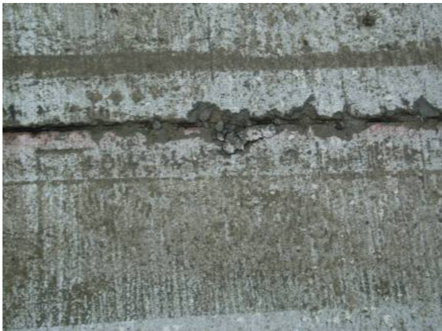
Figure 4-138 Spalling from Premature Saw Cutting
