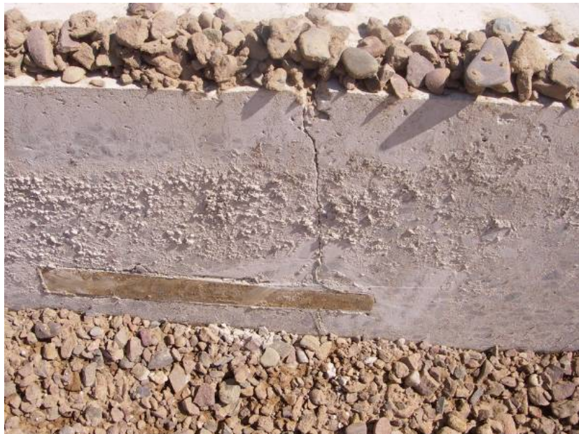
Figure 4-50 Misaligned Contract Joint Dowels
