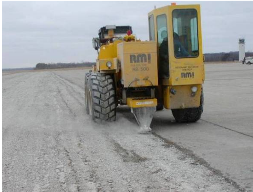
Figure 4-32 Resonant Pavement Demolition
