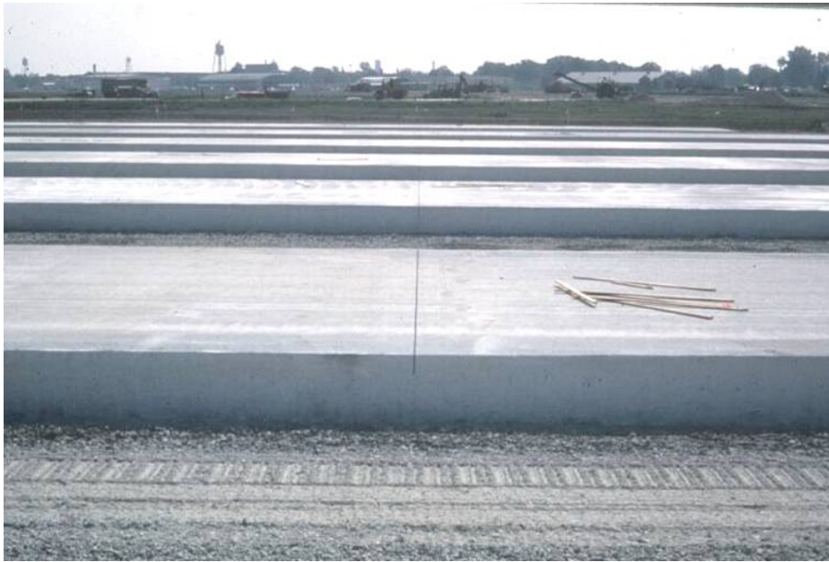
Figure 4-136 Lined Up Transverse Joints Across Pilot Lanes
