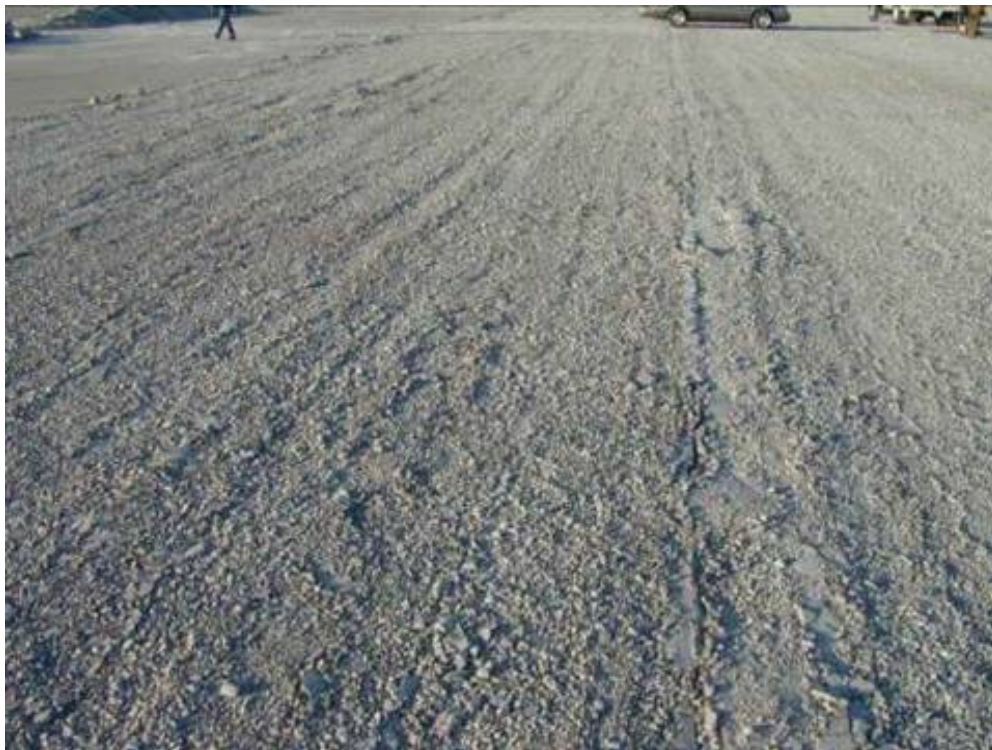
Figure 4-33 Rubblized Surface With The Resonant Rubblizing Technique
