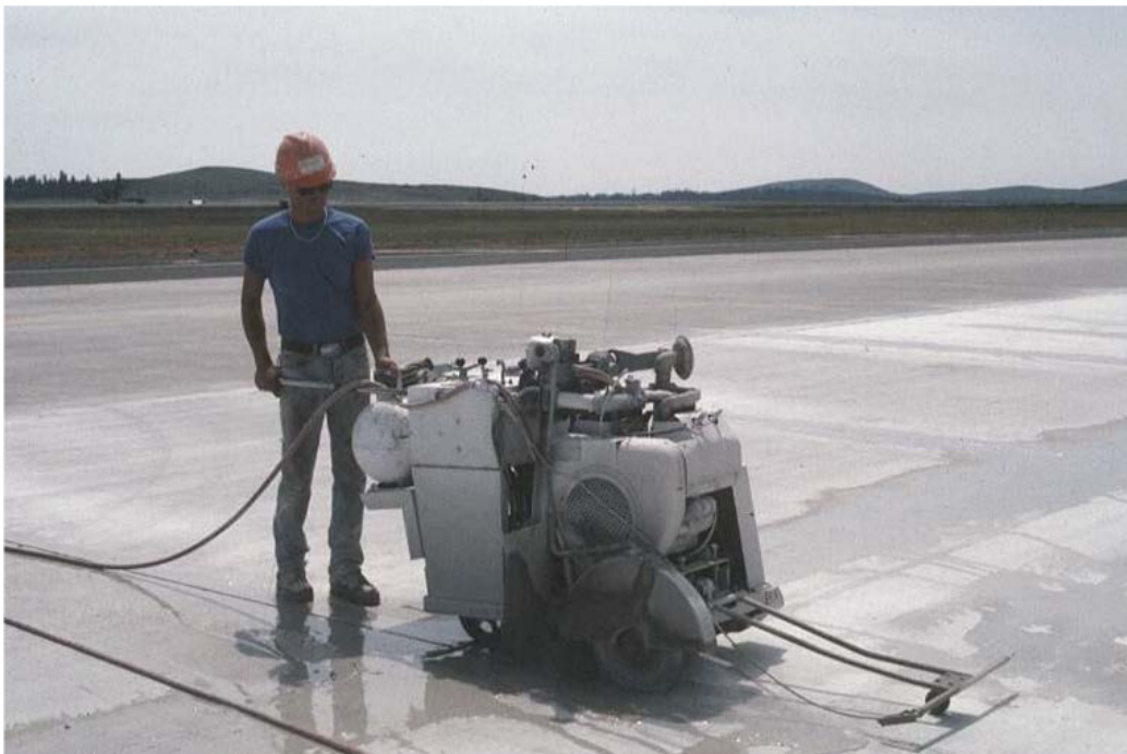
Figure 4-139 Early Entry Saw
