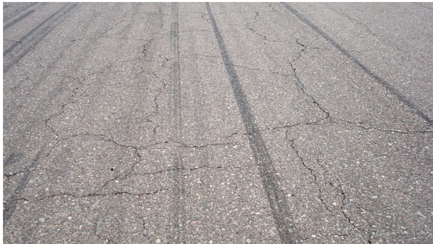
Figure 3-61 Block Cracking
