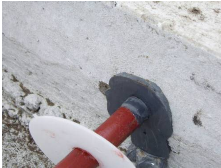
Figure 4-63 Dowel with Retention Ring
