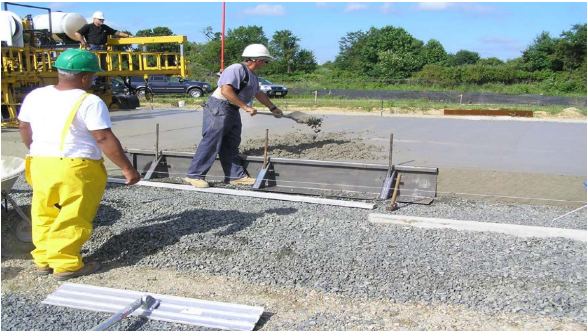
Figure 4-85 Acceptable Repair of Edge Slump
