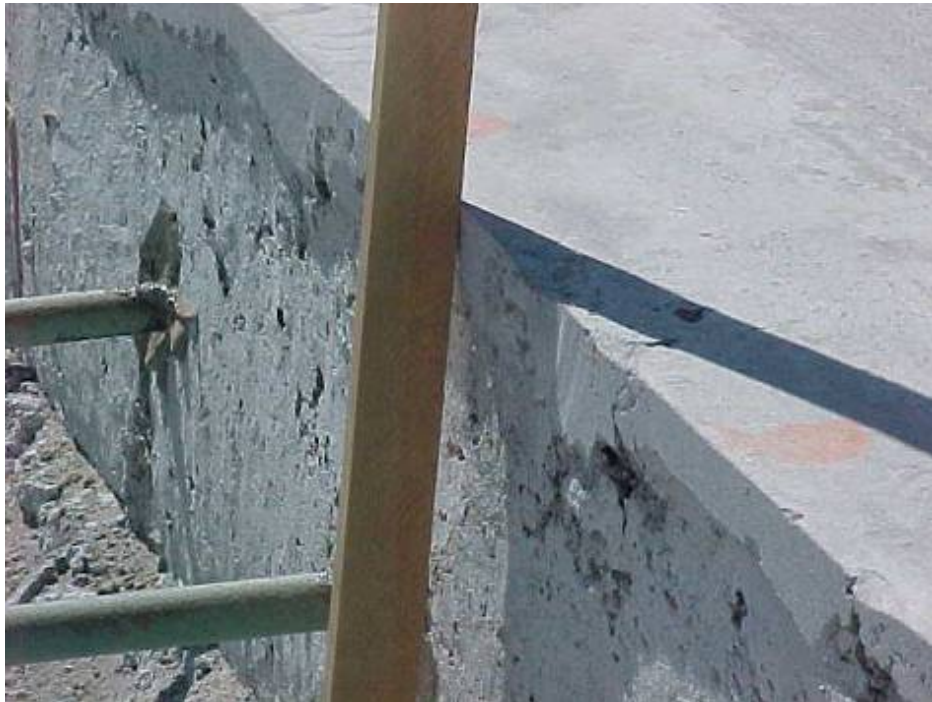
Figure 4-131 Out of Tolerance Joint Construction –Vertical Edge
