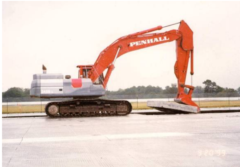
Figure 4-30 Removal of Saw-Cut Pavement Pieces
