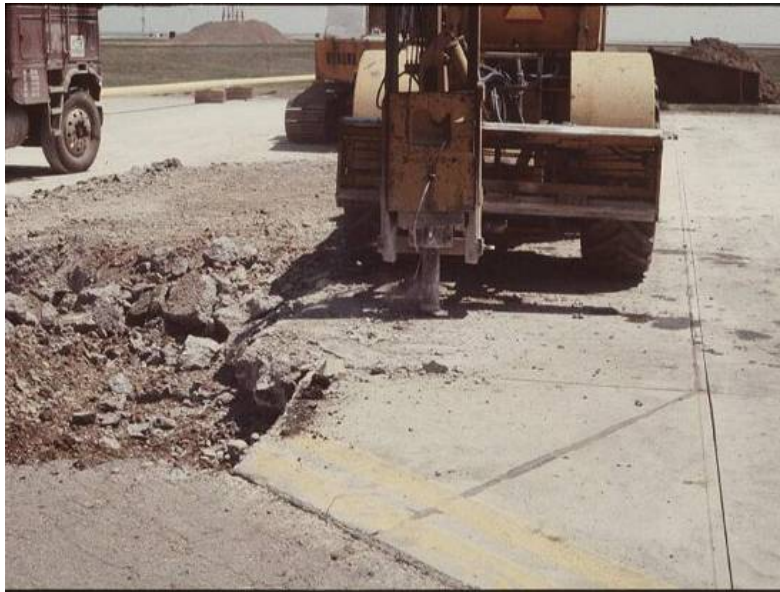
Figure 4-27 Under-breaking from Incorrect Removal Techniques
