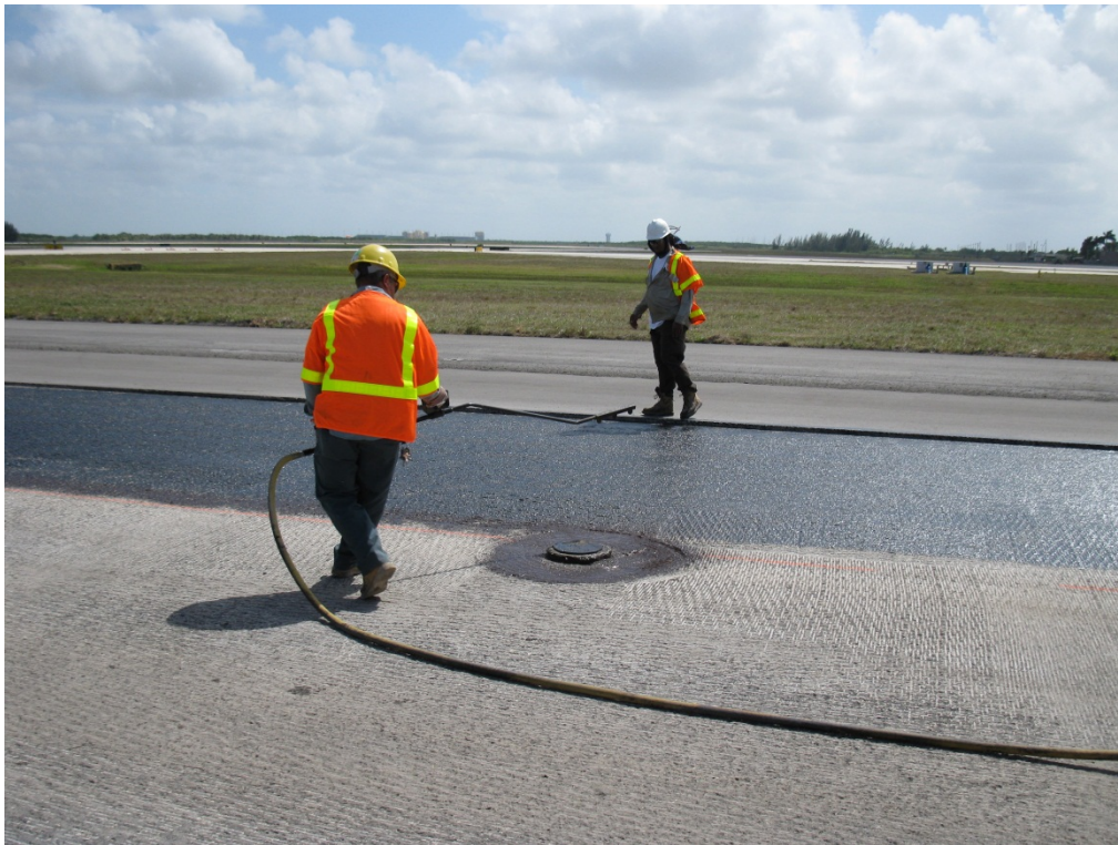
Figure 3-24 Application of Tack Coat with Hand Sprayer
