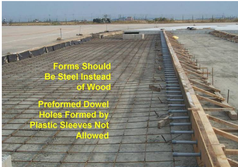
Figure 4-52 Plastic Sleeves on Wood Forms
