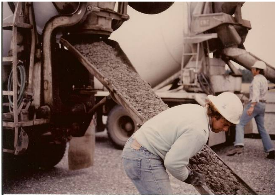
Figure 4-69 Difficulty in Discharging low Slump Concrete From Truck Mixer
