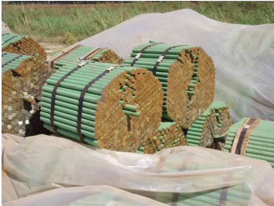
Figure 4-44 Dowels at Contraction Joints
