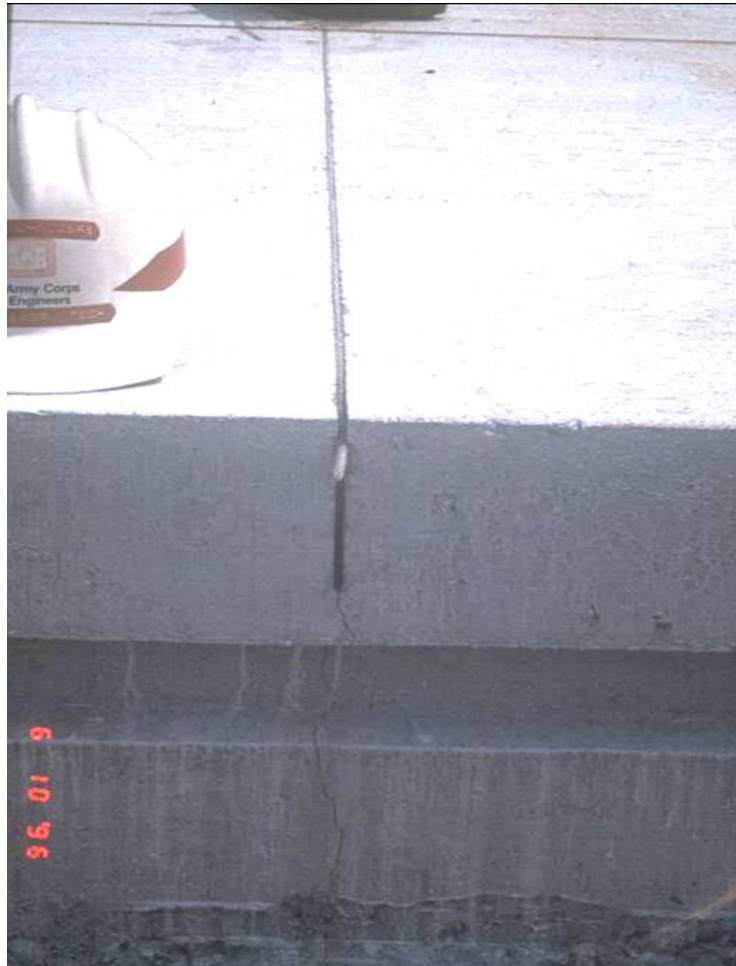
Figure 4-143 Saw Cut With Temporary Foam Rope
