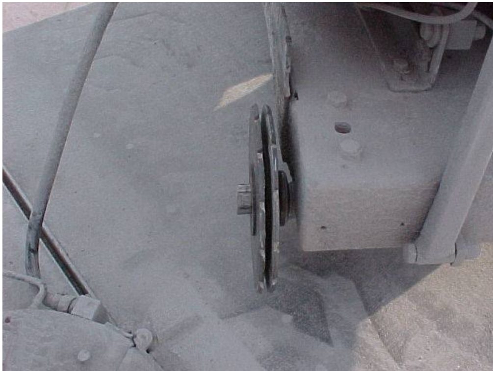
Figure 4-148 Blades used to Chamfer Joint Reservoirs
