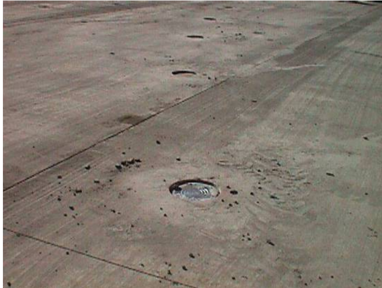
Figure 4-133 Light Cans Properly Located With the Joints
