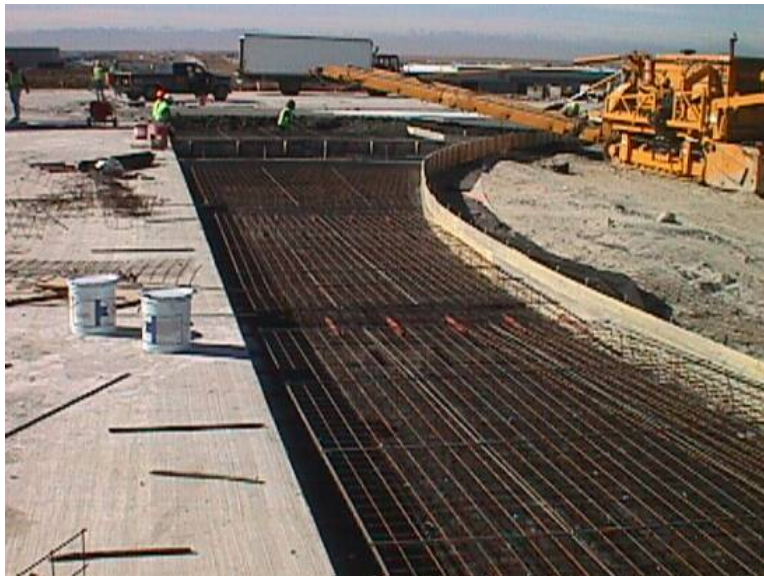
Figure 4-36 Reinforcement Steel for Odd (or Irregular)-Shaped Panels
