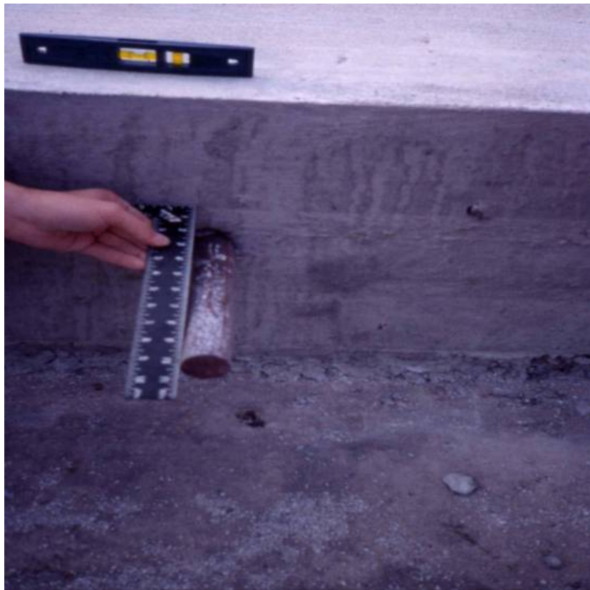
Photo 4-66 Checking Dowel for Horizontal Alignment
