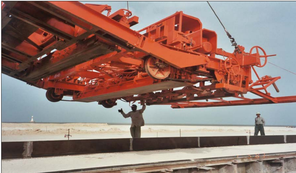
Figure 4-89 British Form-Riding Paver. Note Rail Section on Top of Forms
