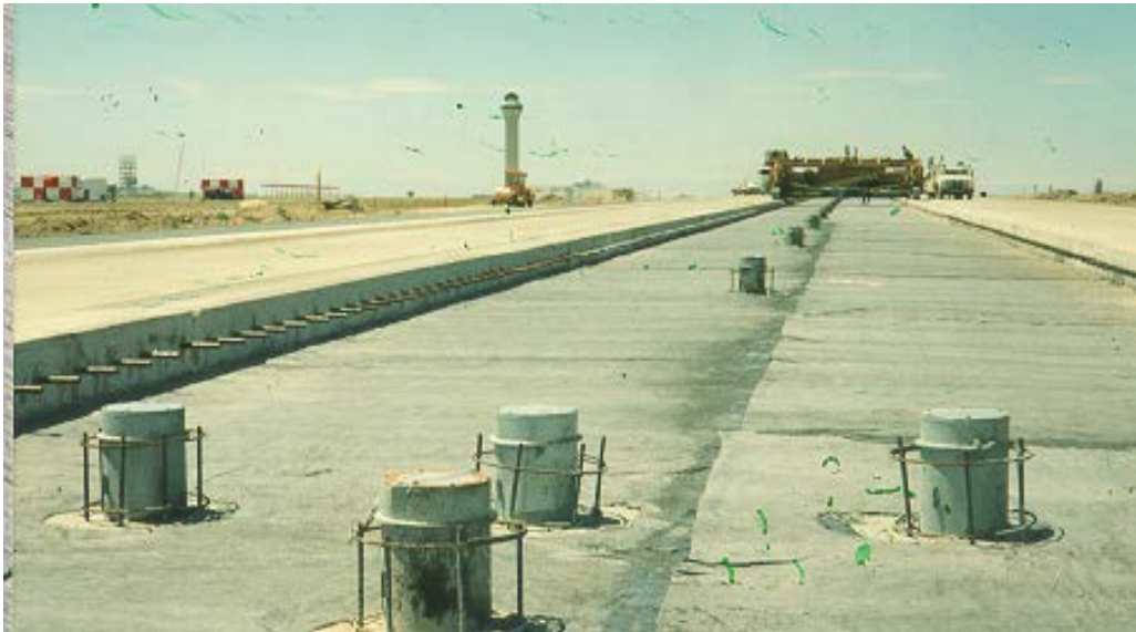
Figure 4-72 Light Cans in Paving Lane
