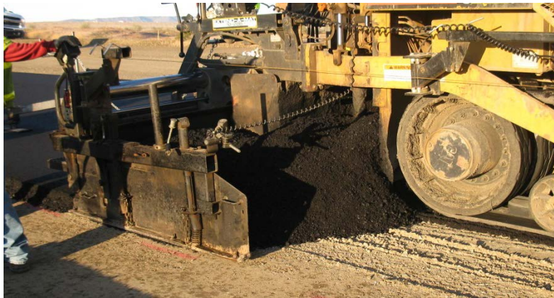
Figure 3-37. Excessive Distance between Auger and Side Plate
