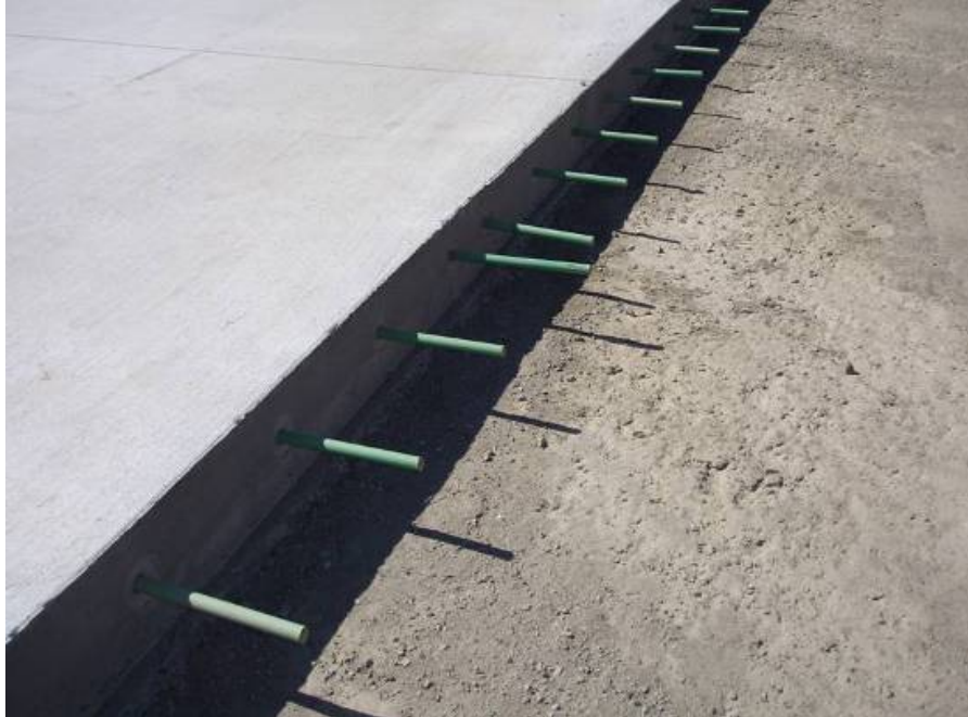
Photo 4-65 Misaligned Dowels
