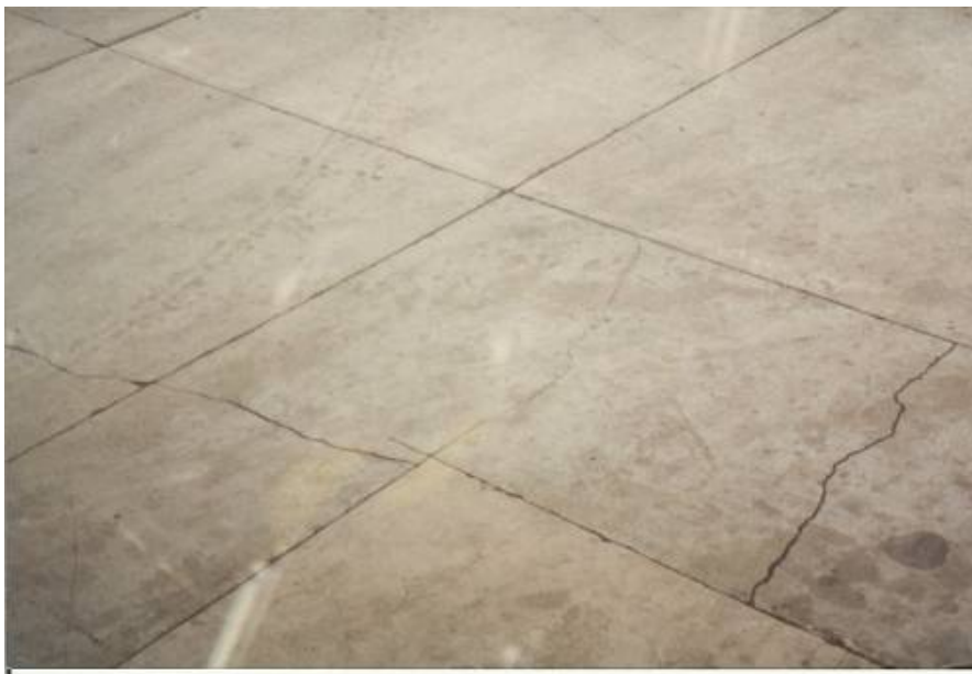
Figure 4-132 Cracks Induced by Partial Panel Replacement
