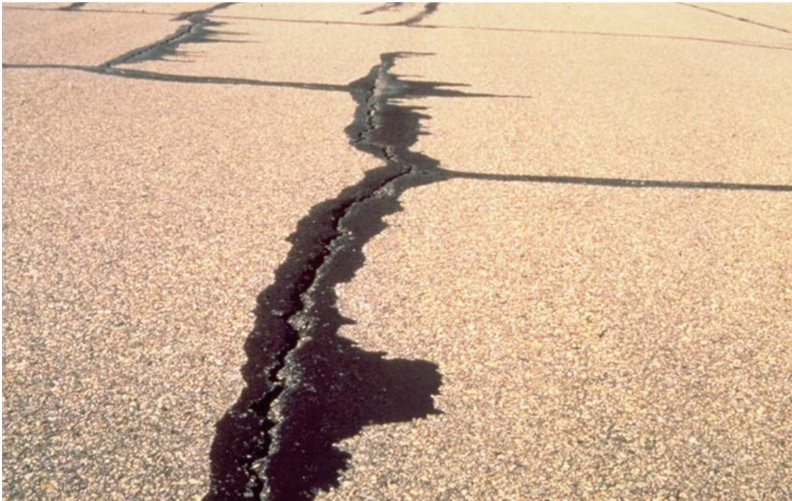
Figure 3-19 Excess Sealant
