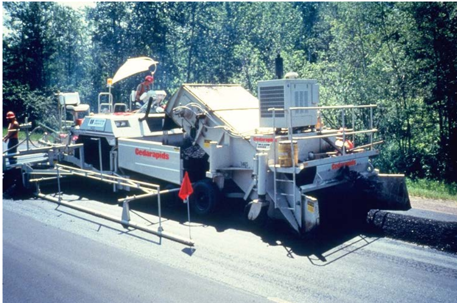
Figure 3-28 Dumping Directly into Paver
