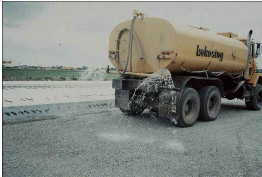
Figure 4-19 Dampening the Base Course
