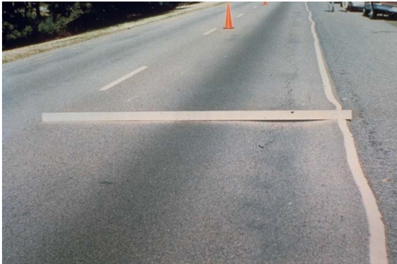
Figure 3-61 Block Cracking
