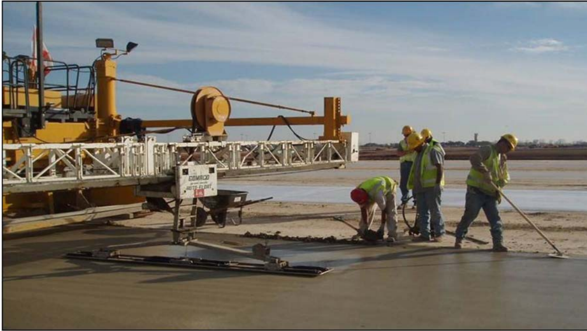
Figure 4-102 Longitudinal Float Behind Slipform Paver
