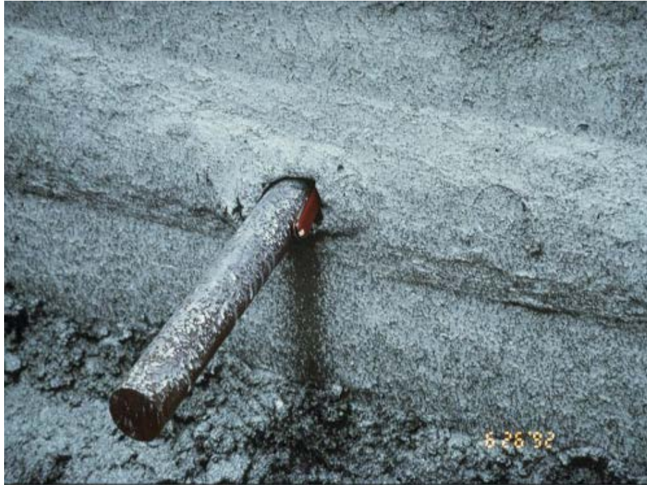
Figure 4-54 Voids around an Inserted Dowel
