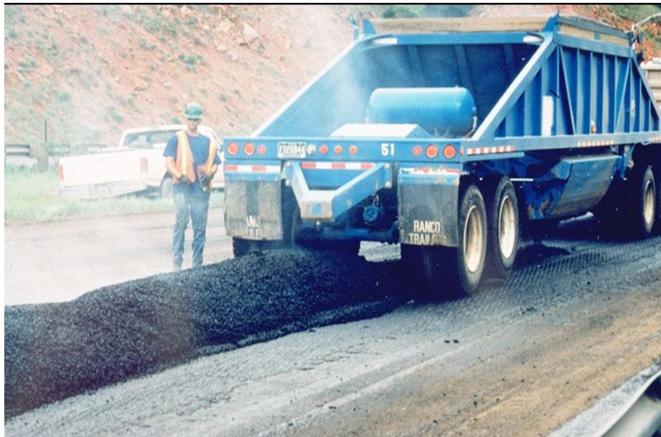
Figure 3-26 Placing of Windrow
