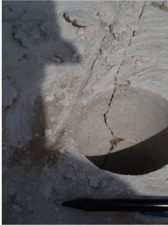
Figure 4-40 Cracked Panels from Misplaced Reinforcement Steel
