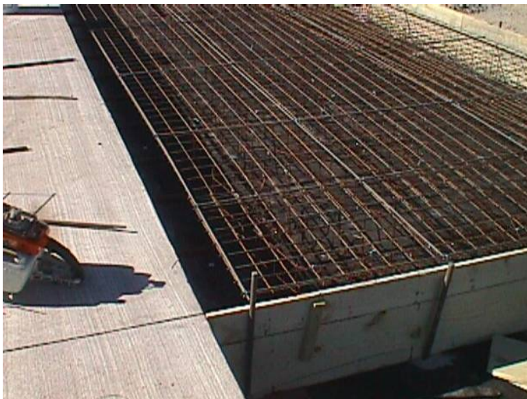
Figure 4-36 Reinforcement Steel for Odd (or Irregular)-Shaped Panels
