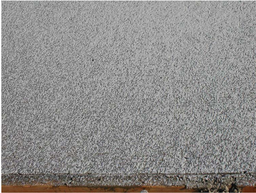
Figure 4-119 Excessive Rain Damage
