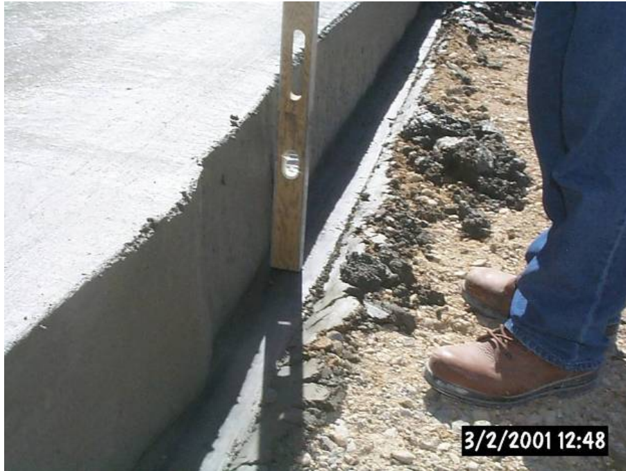
Figure 4-129 Poor Quality Construction Joint
