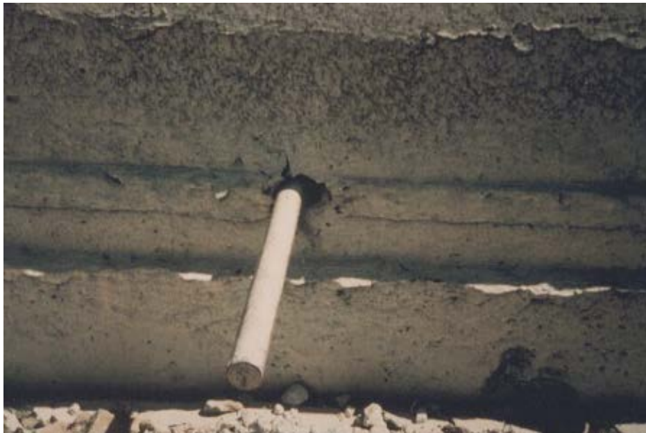
Figure 4-54 Voids around an Inserted Dowel
