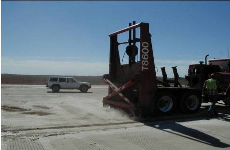
Figure 4-29 Demolition With No Protection of Adjacent Concrete
