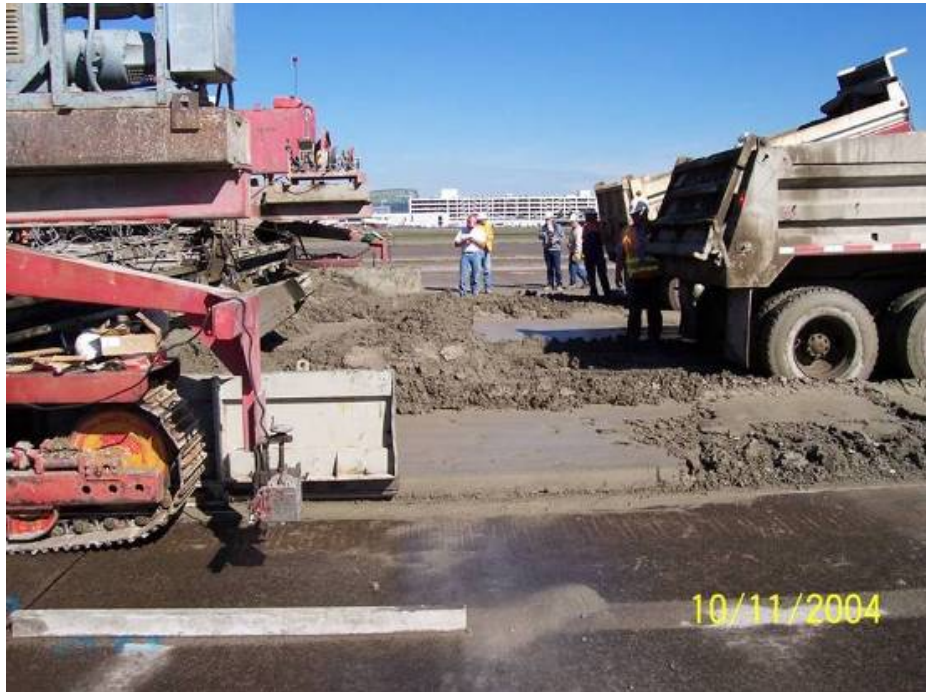
Figure 4-77 Backing Trucks Down Paving Lane
