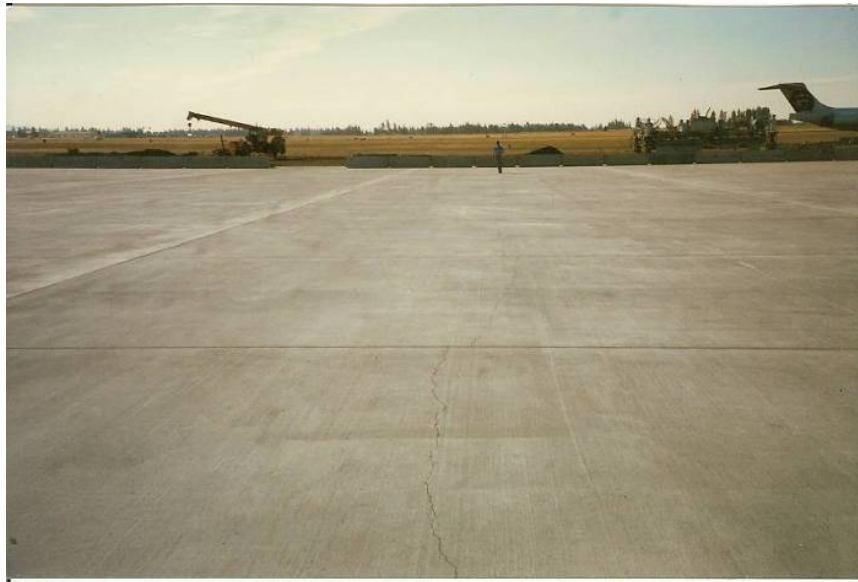
Figure 4-127 Mid-panel Cracking
