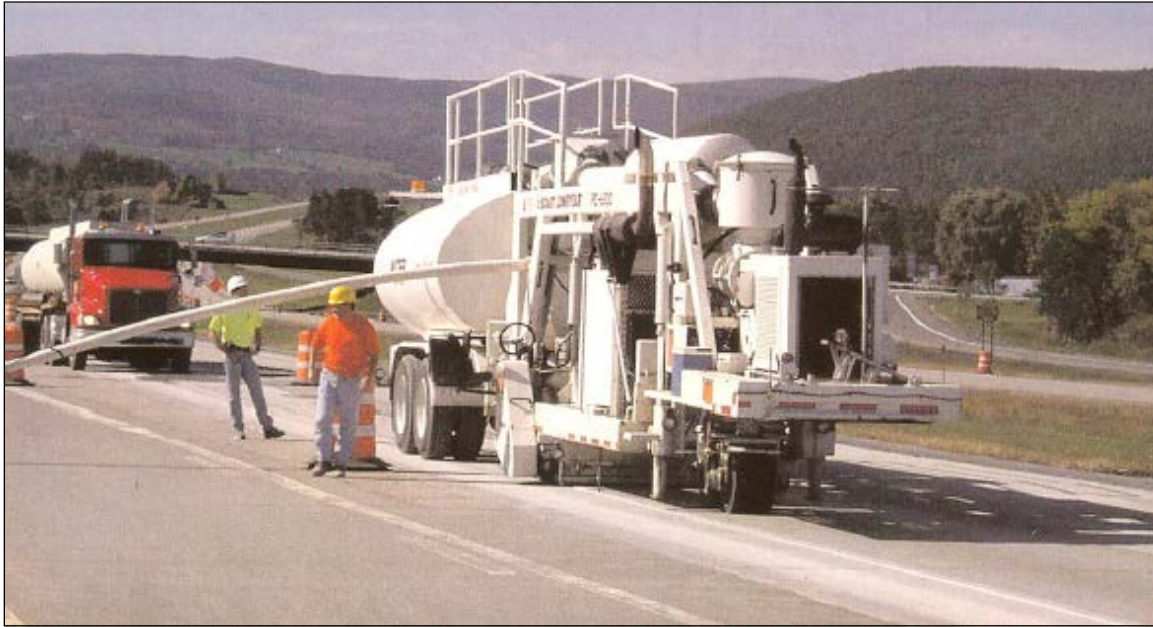
Figure 4-126 Diamond Grinding
