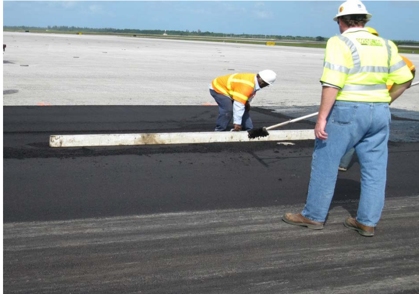
Figure 3-51 Using Straightedge to Check Smoothness
