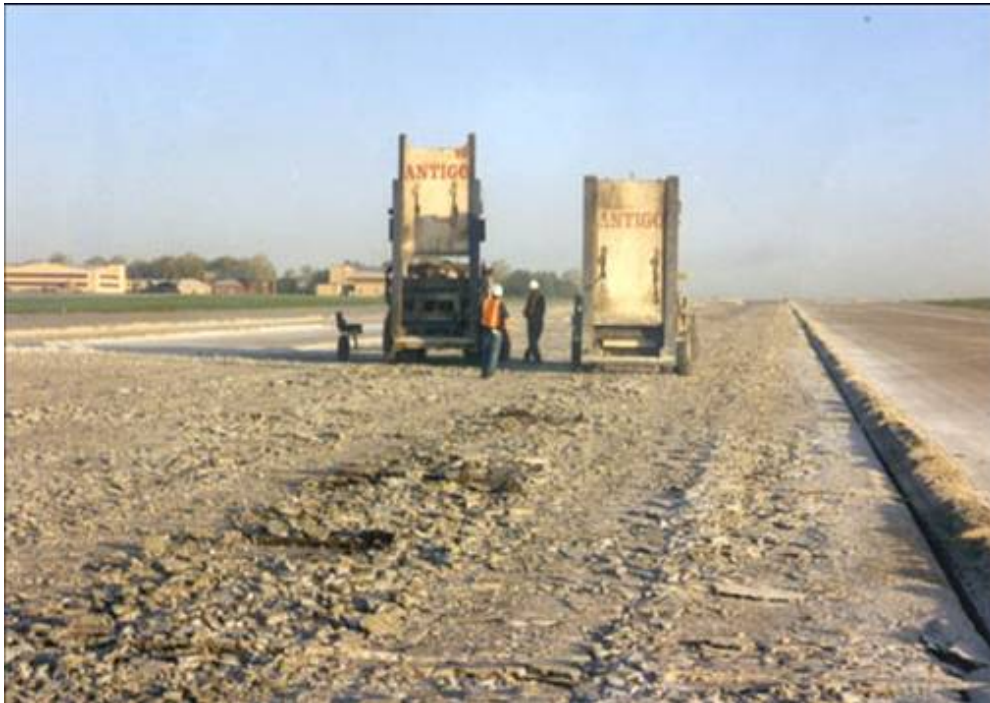
Figure 4-25 Improper removal Techniques - No Double Saw Cut
