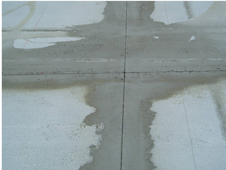
Figure 4-140 Cuttings Not Removed
