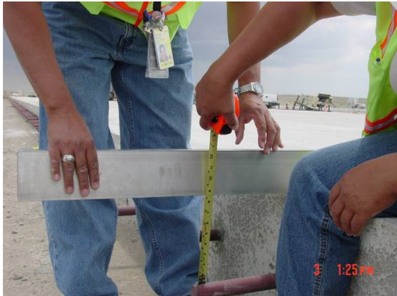
Figure 4-67 Checking Dowel for Vertical Alignment
