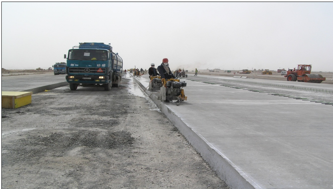
Figure 4-158 Saw Cutting Vertical Joint Face
