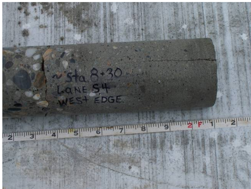
Figure 4-70 Segregated Concrete with no Coarse Aggregate on Right Side of Core
