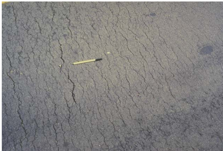
Figure 3-46 Checking Under Steel Wheel Rollers
