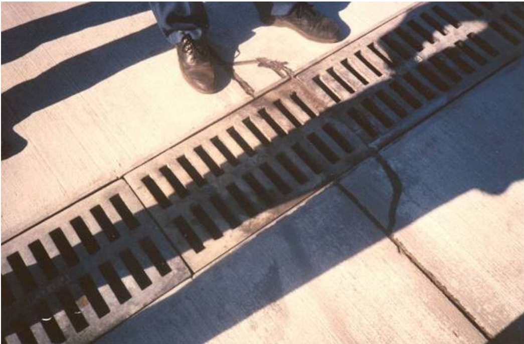
Figure 4-135 Drainage Structure – Joint Lines not matched and Random Cracking
