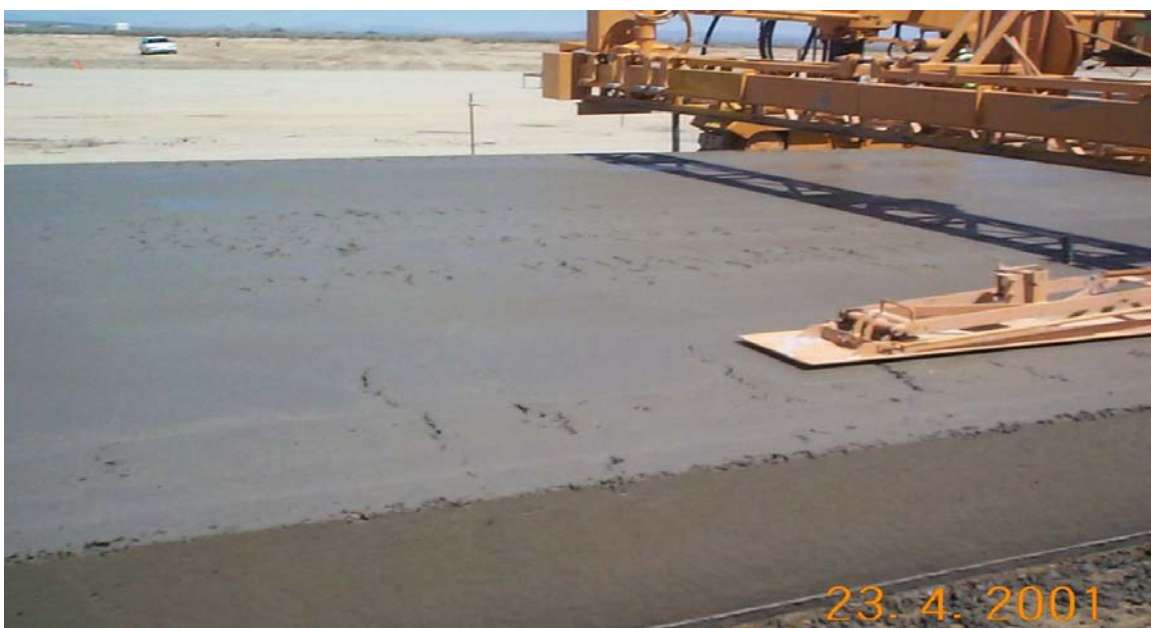
Figure 4-81 Poor Consolidation on Horizontal Surface of Slab
