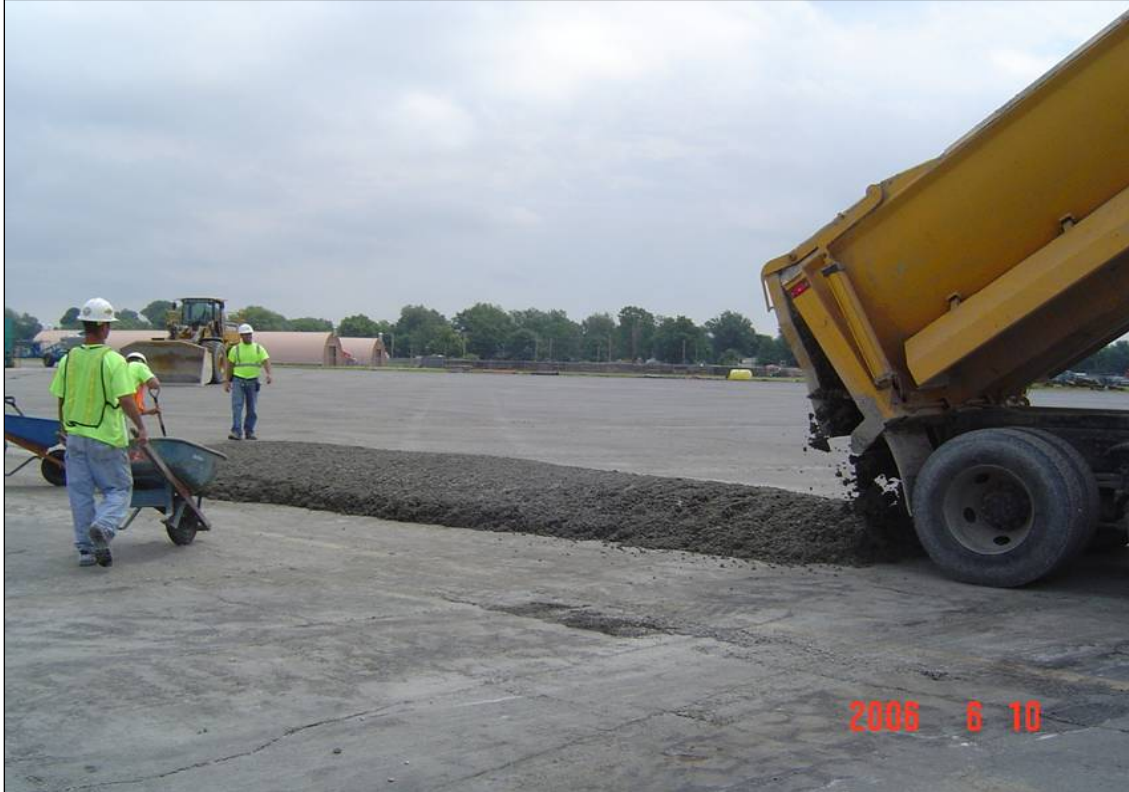
Figure 4-9 Spreading a Batch for Sampling
