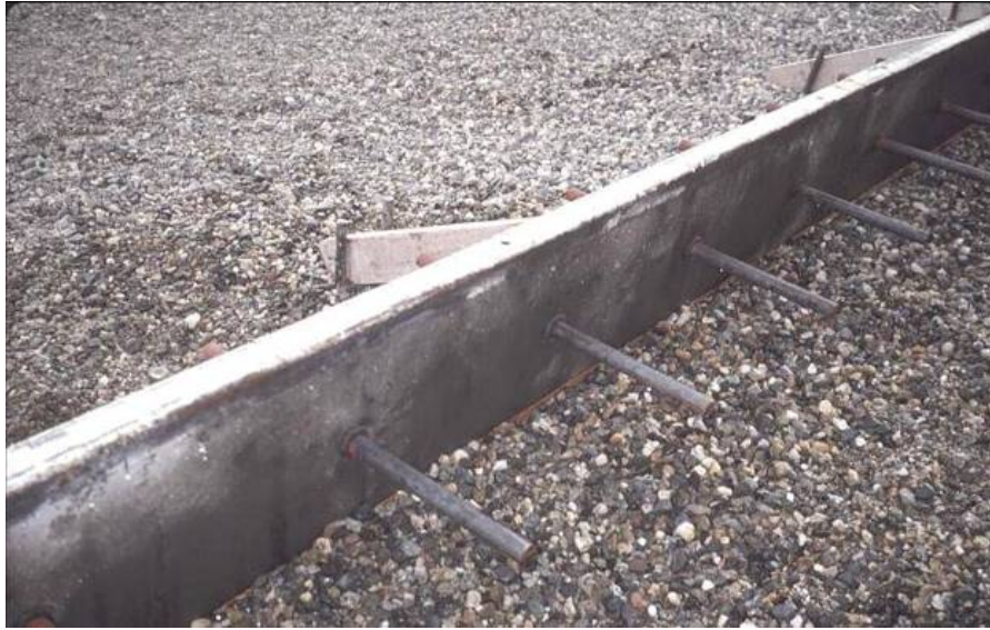
Figure 4-51 Dowels in Steel Forms
