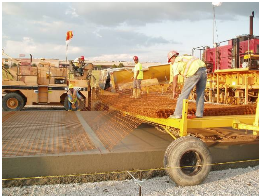
Figure 4-39 Gap in Reinforcing steel at Contraction Joint
