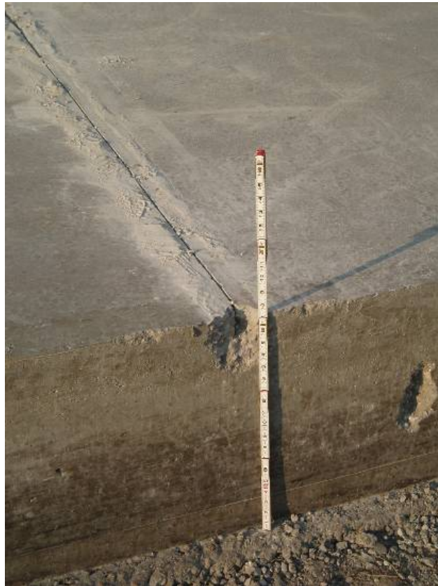
Figure 4-138 Spalling from Premature Saw Cutting
