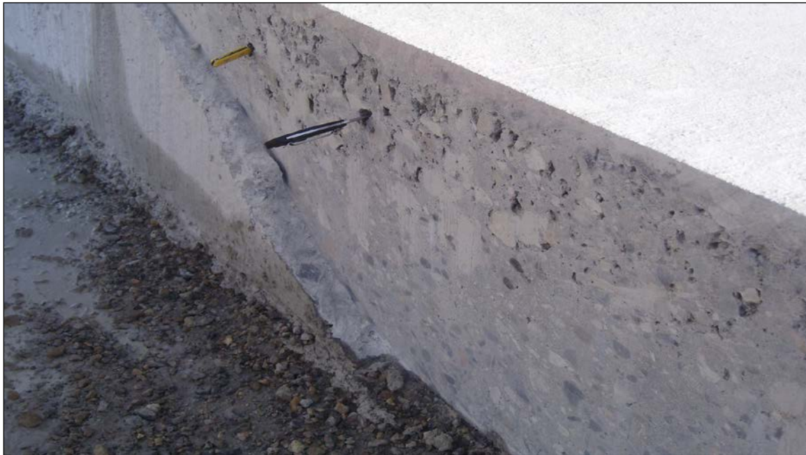
Figure 4-80 Poor Consolidation of Vertical Face of Slab
