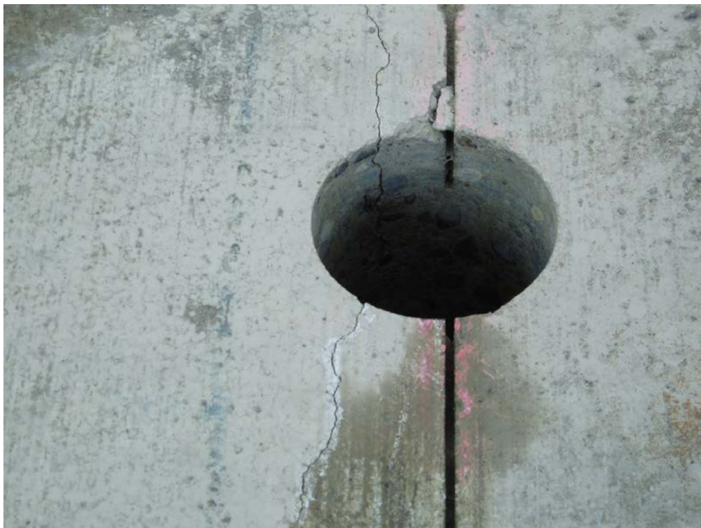
Figure 4-145 Core to Verify Depth of Crack
