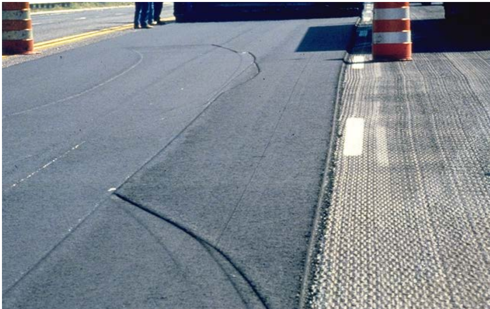
Figure 3-47 Excessive Roller Marks
