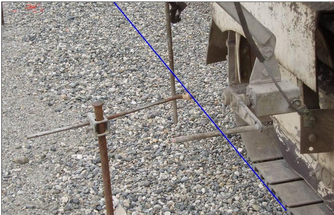
Figure 4-79 Typical String Line Alignment, Showing, Supports, Whisker Poles, and String Line
