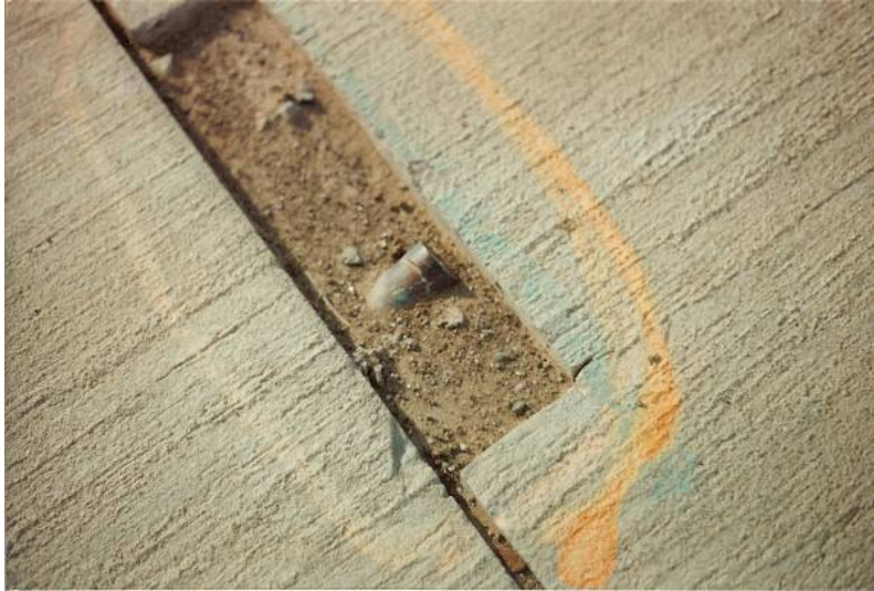
Figure 4-50 Misaligned Contract Joint Dowels
