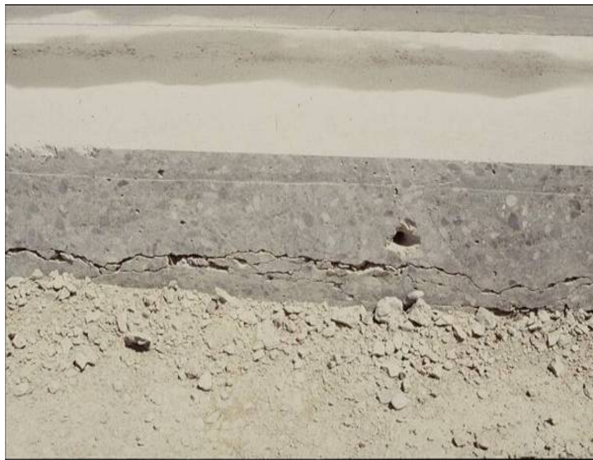
Figure 4-27 Under-breaking from Incorrect Removal Techniques
