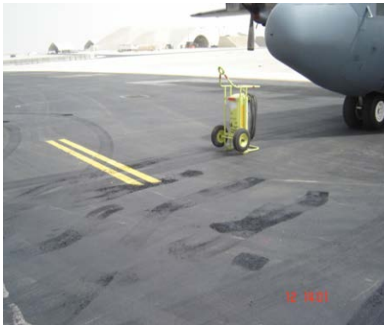
Figure 3-55 Surface Distortion
