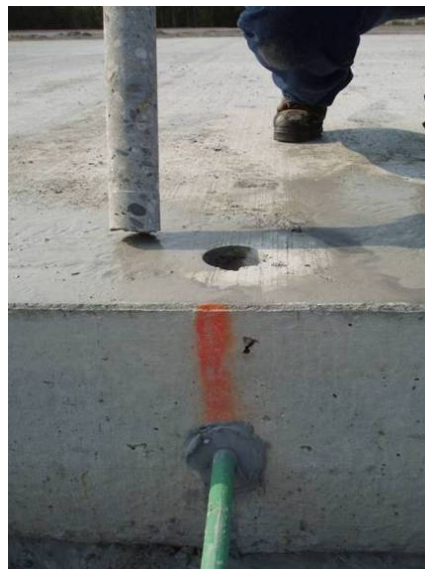
Figure 4-64 Cored Dowel to Verify the Grouting Technique
