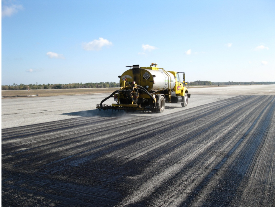
Figure 3-23 Excess amount of Tack Coat
