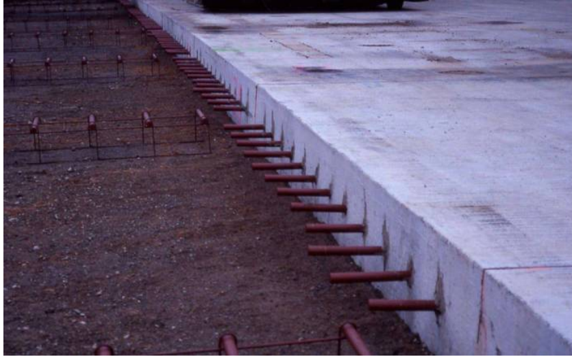
Figure 4-43 Dowel Ends not Epoxy Coated
