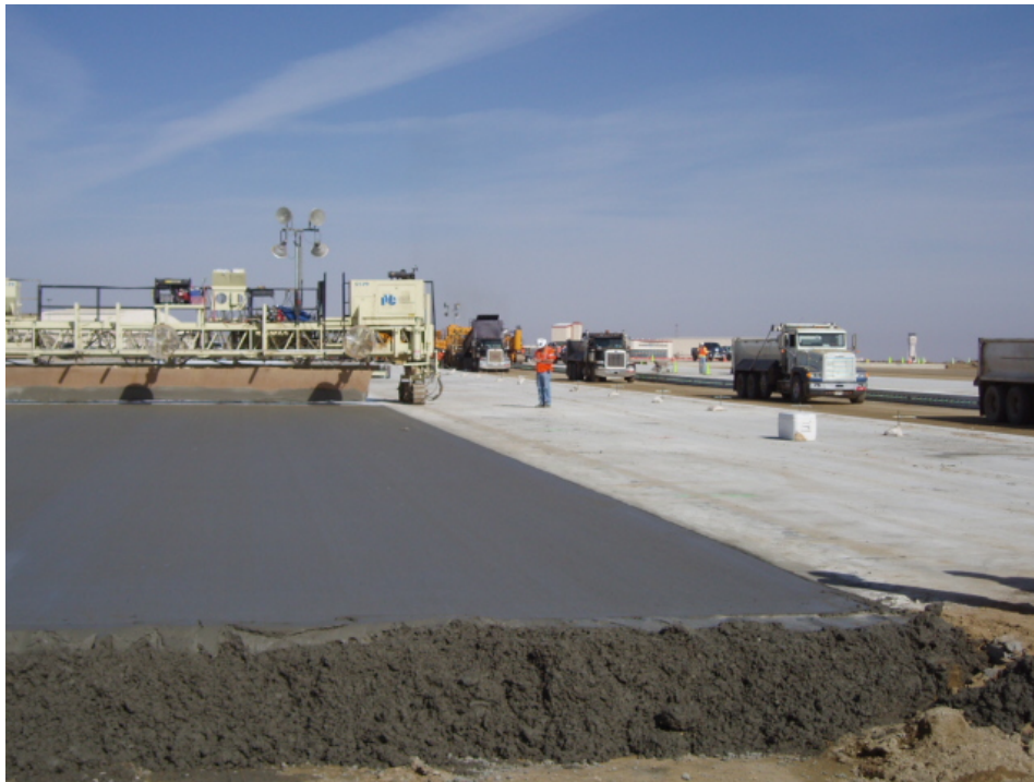
Figure 4-68 Backup of Trucks at Paving Site
