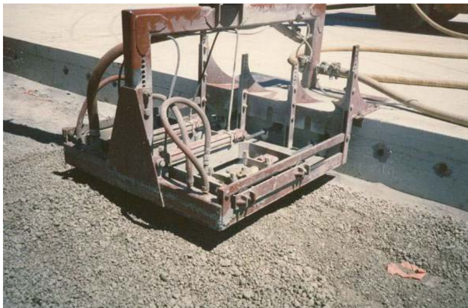
Figure 4-56 Drilling Construction Joint Dowel Holes
