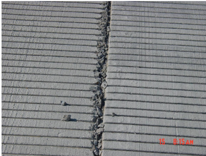
Figure 4-121 Spall Damage
