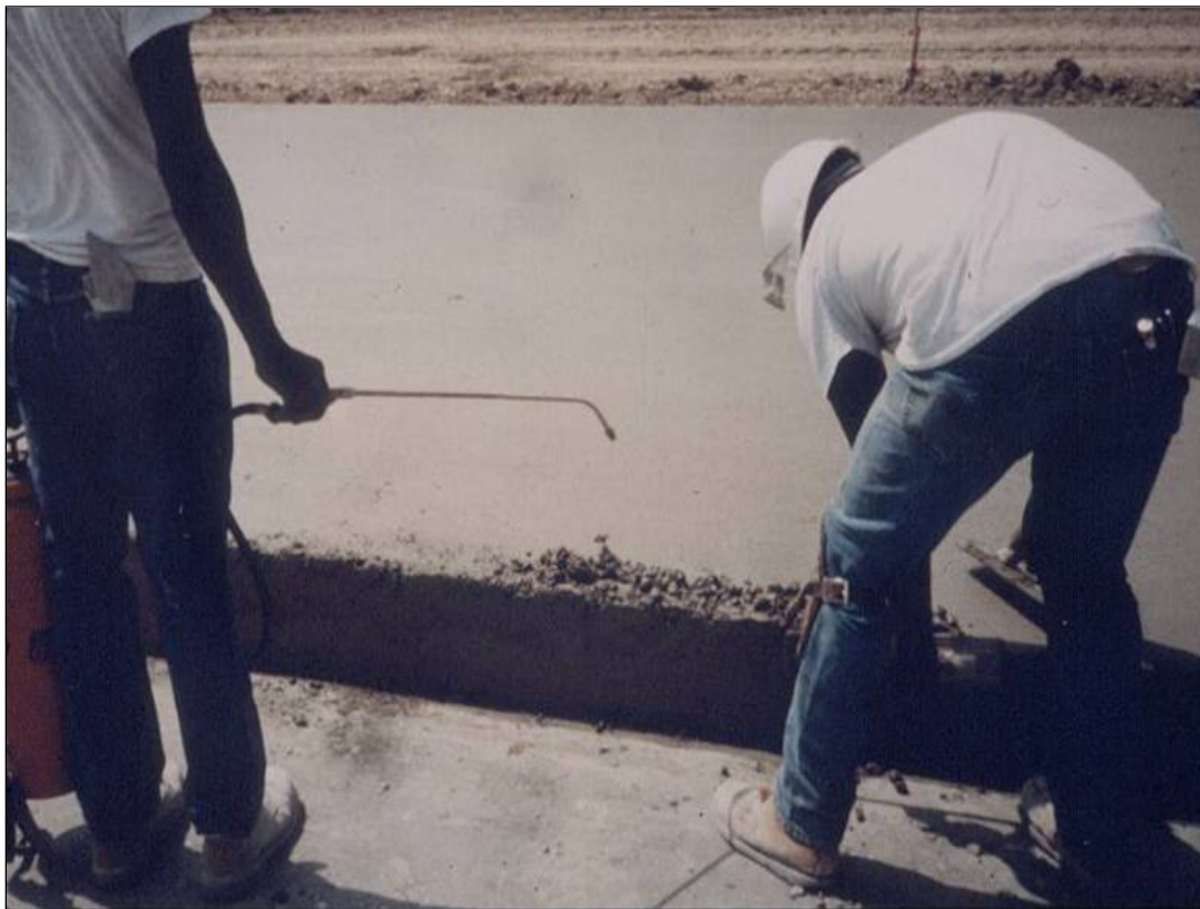
Figure 4-161 Over Finishing Edge of Pilot Lane
