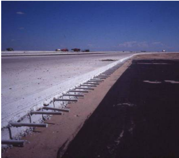
Figure 4-55 Alignments of Inserted Dowels
