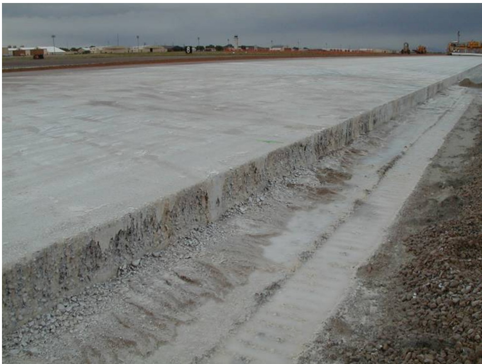
Figure 4-119 Excessive Rain Damage
