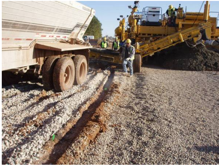
Figure 4-20 Disturbed Base Course from Equipment
