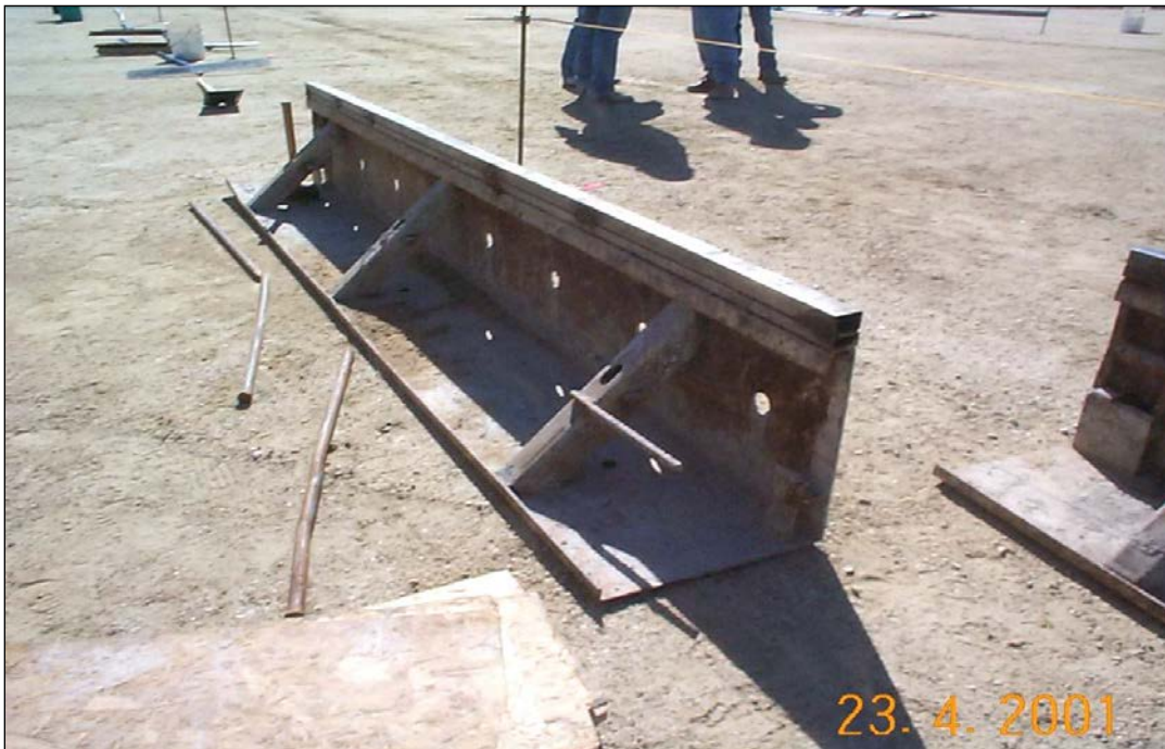
Figure 4-87 Fixed Form. Note Hole for Dowels in Middle of Form Face
