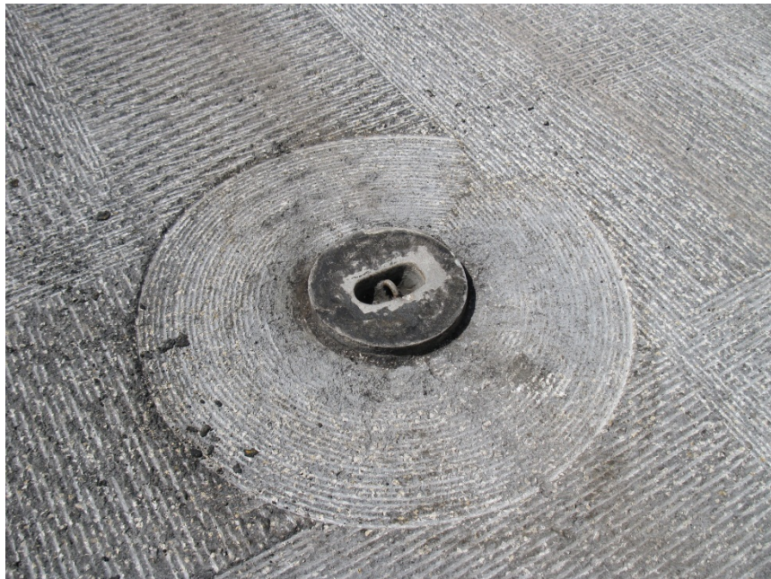
Figure 3-17 Surface Milled with Small Milling Machine Adjacent to Tie Down
