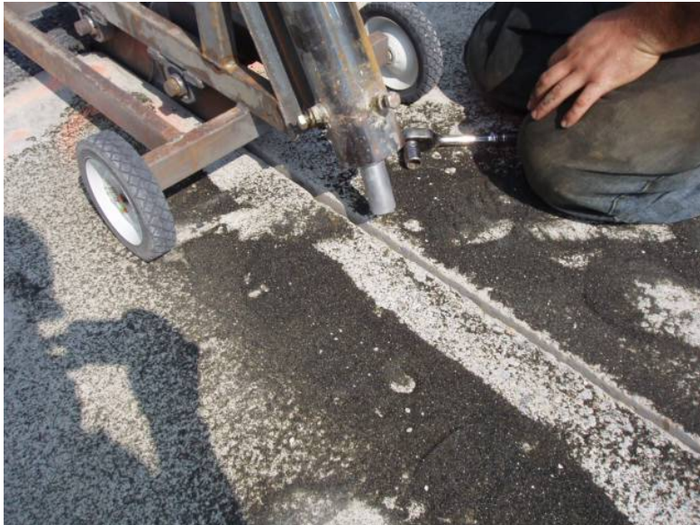
Figure 4-150 Sandblasting Joint
