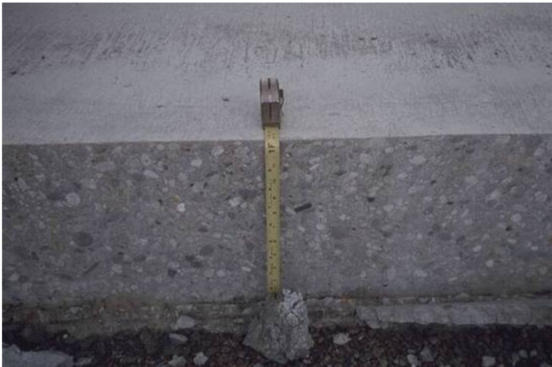
Figure 4-21 Full Depth Sawcut
