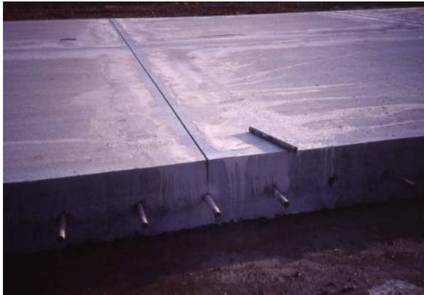
Figure 4-46 Dowel Located on a Contraction Joint.
