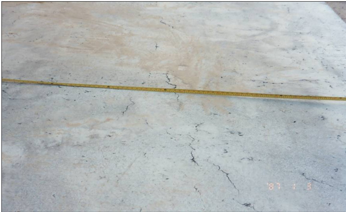
Figure 4-159 Plastic Shrinkage Cracking
