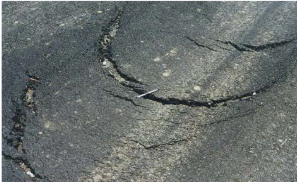
Figure 3-58 Slippage of Asphalt Mixture over Underlying Layer
