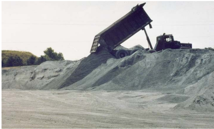
Figure 3-6 Improper Addition of Material to a Stockpile
