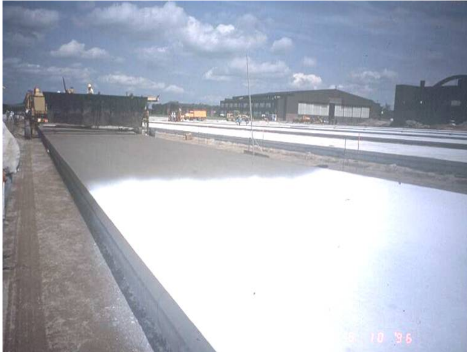
Figure 4-114 Good Application With Overlapping Spray and Windscreens
