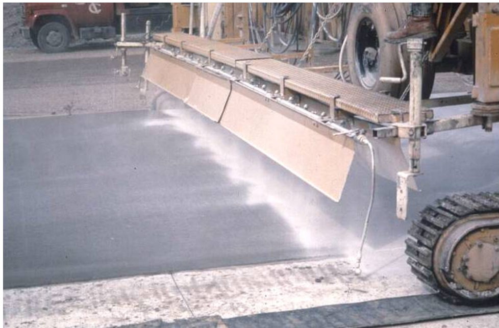
Figure 4-114 Good Application With Overlapping Spray and Windscreens
