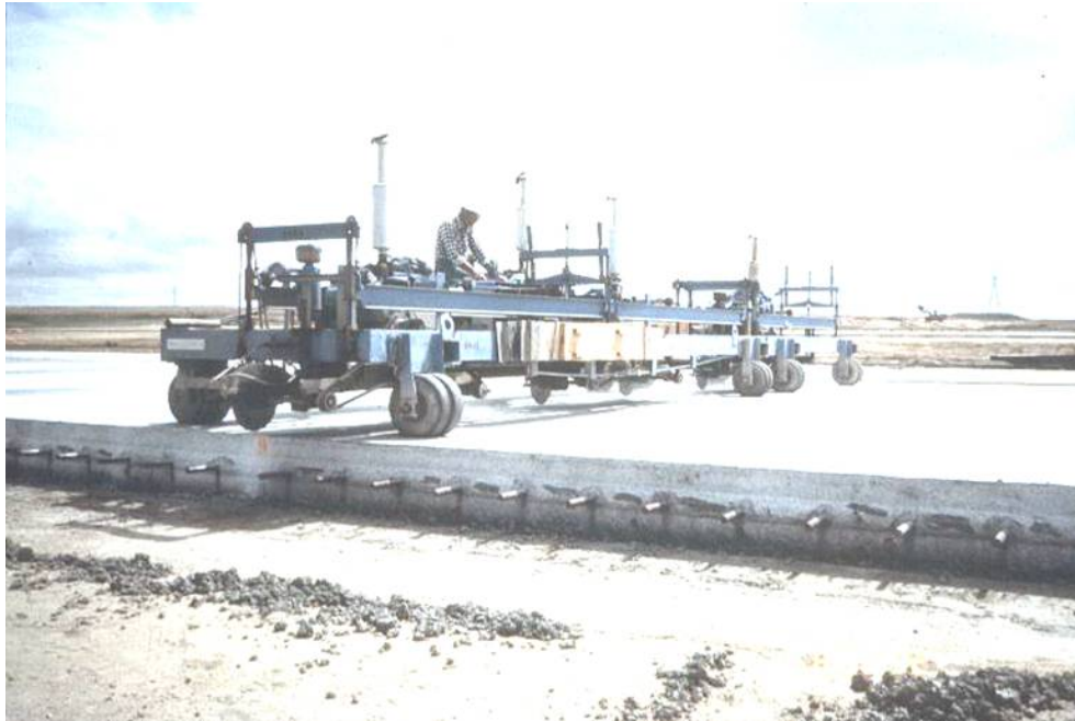
Figure 4-116 Poor Application of Curing Compound Vertical Joint
