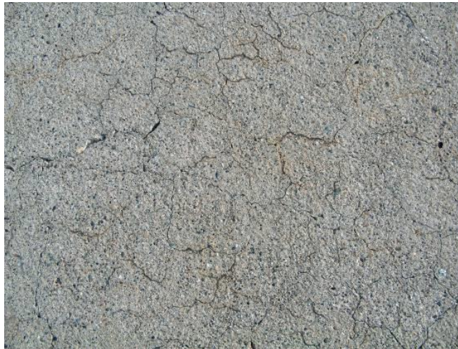
Figure 5-4 Example of Low Reactivity ASR at Travis AFB
