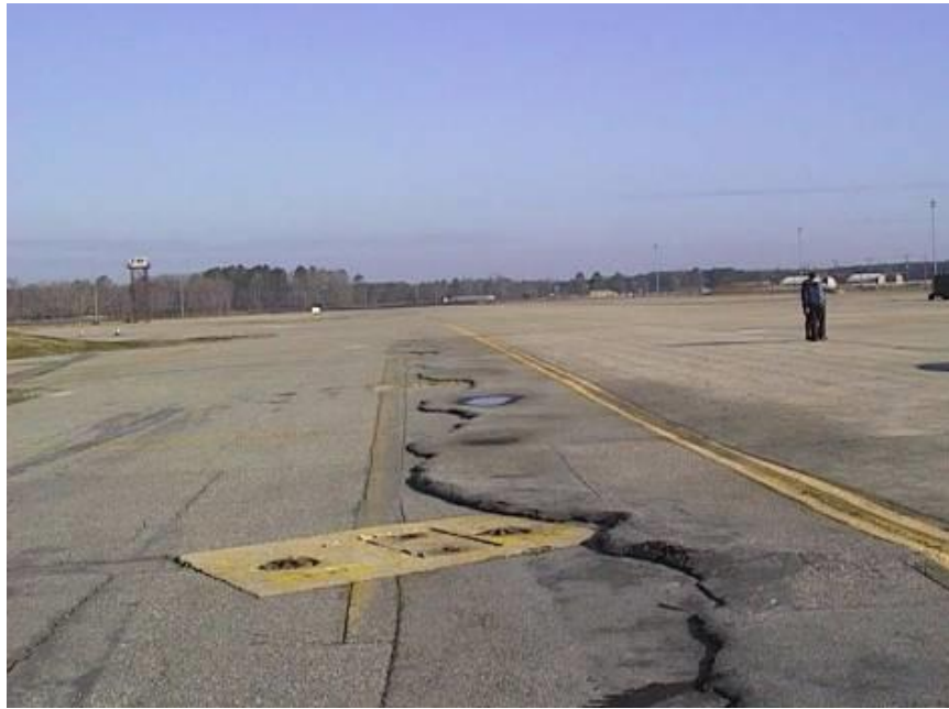
Figure 5-2 Examples of Damage to Adjacent Asphalt from ASR-Induced Expansion in Adjacent PCC Pavement
