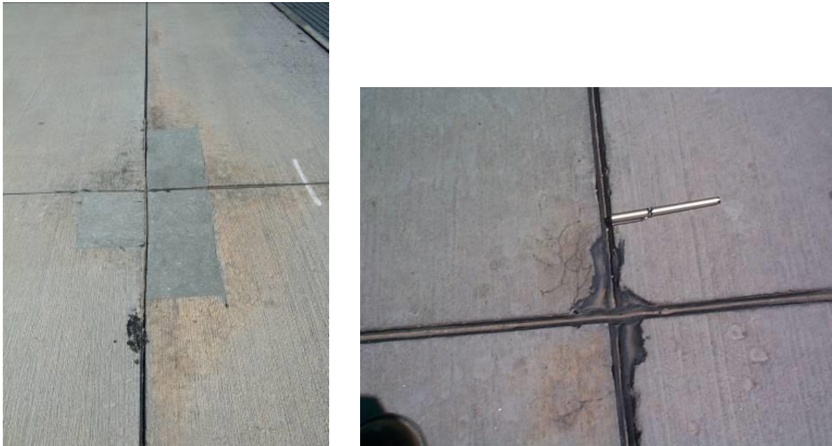
Figure 5-1 Minor ASR Cracking in 5-Year-Old Pavement (Left Photograph); Patching Needed 3-Years Later (Right Photograph)
