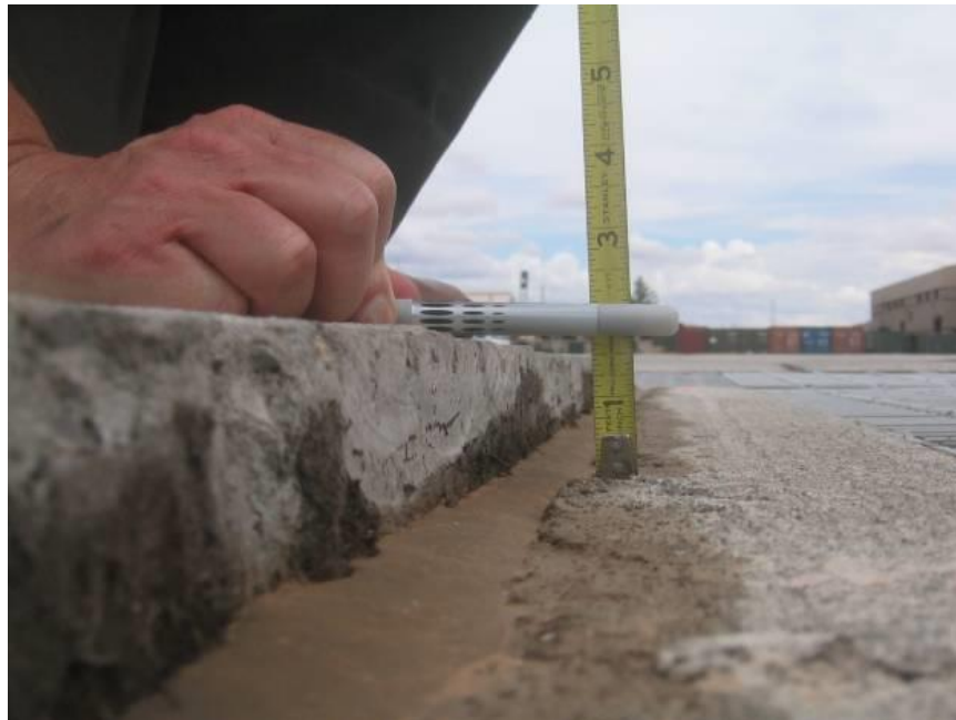
Figure 3-1 Example of Differential Heaving on a Rigid Pavement Caused by Volume Change in Underlying Base and Fill Layers
