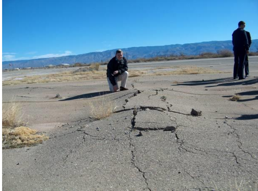
Figure 3-2 Example of Localized Heaving in a Flexible Pavement Caused by Volume Change in the Underlying Base Course
