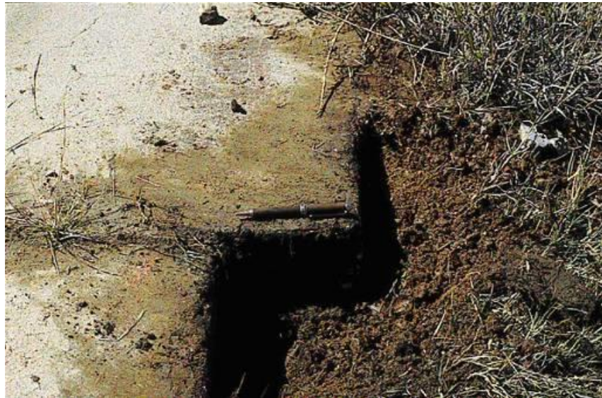
Figure 5-3 Examples of Large Volume Changes Suggesting Highly Reactive ASR Pavements
