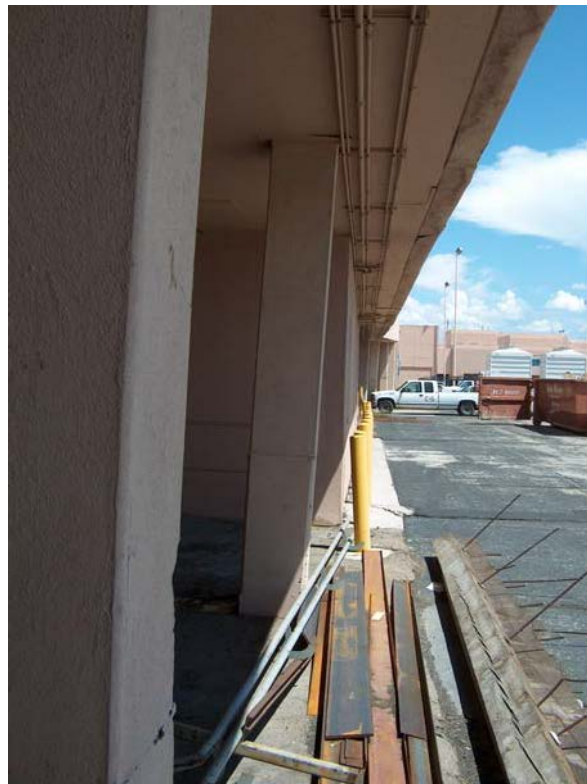
Figure 10 Building Column Pushed Out of Alignment by ASR Volume Expansion in Adjacent Concrete Pavement, Albuquerque, NM
