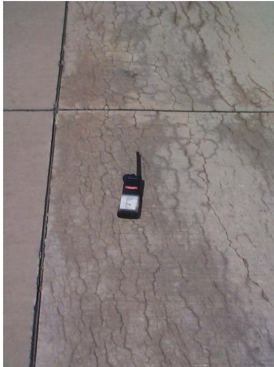
Figure 2 ASR-induced Cracking on Taxiway, Holloman AFB
