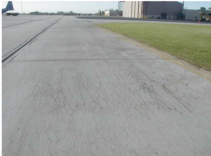
Figure 3 ASR-induced Cracking in Taxiway at Channel Island ANG Facility
