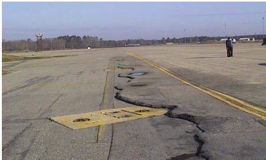
Figure 8 Asphalt Shoulder Heaving Caused by ASR Expansion in Adjacent Concrete at Seymour-Johnson AFB
