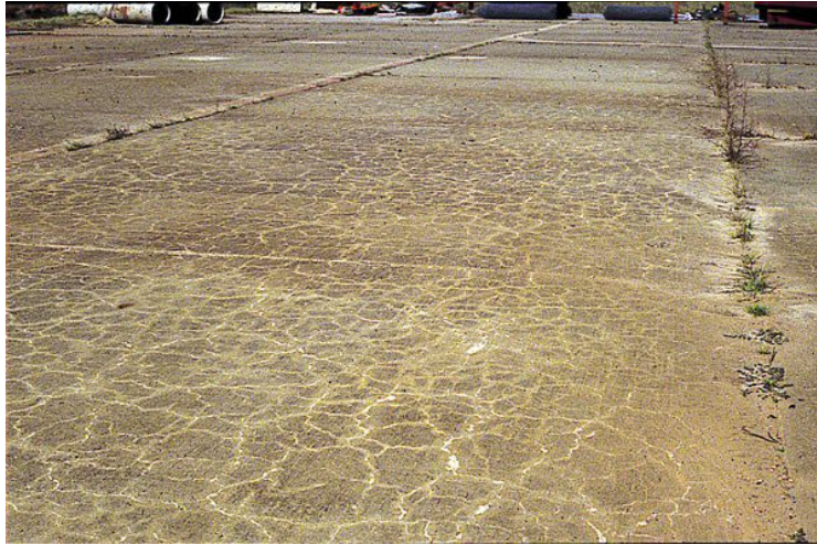
Figure 4 ASR-induced Cracking in Ramp at Tinker AFB
