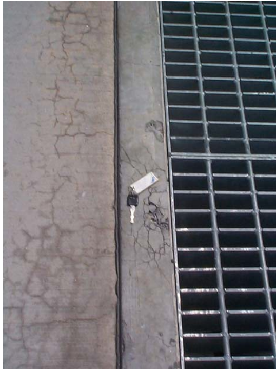
Figure 10 Building Column Pushed Out of Alignment by ASR Volume Expansion in Adjacent Concrete Pavement, Albuquerque, NM
