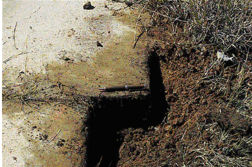
Figure 8 Asphalt Shoulder Heaving Caused by ASR Expansion in Adjacent Concrete at Seymour-Johnson AFB
