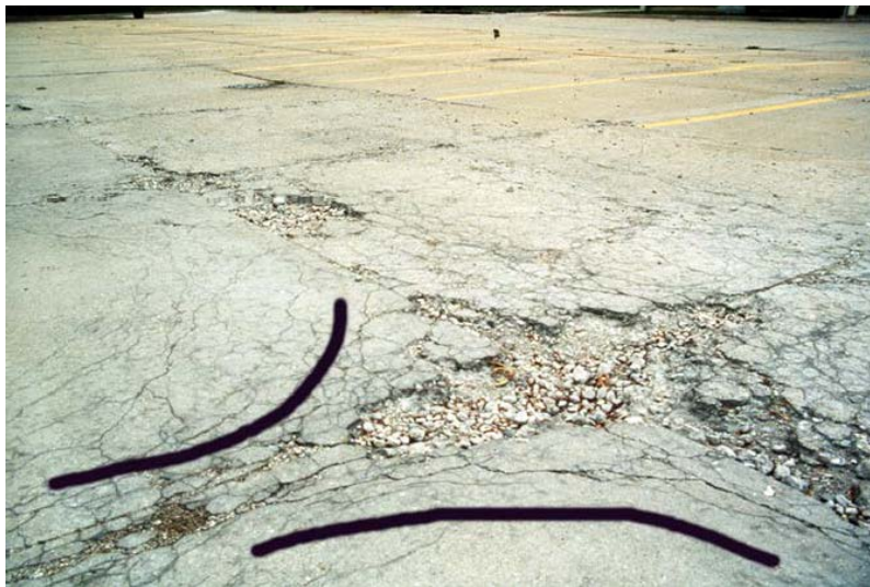
Figure 6 D-cracking at Grissom AFB
