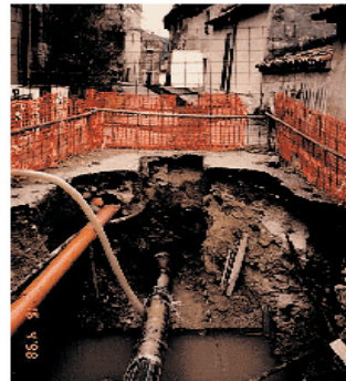
"Open cut", a well established technique.
