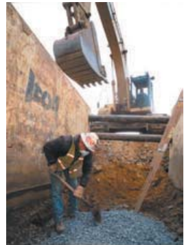
OSHA's excavation standard requires employers to provide sloping, benching, shoring, or shielding to protect workers in excavations five feet or deeper.
