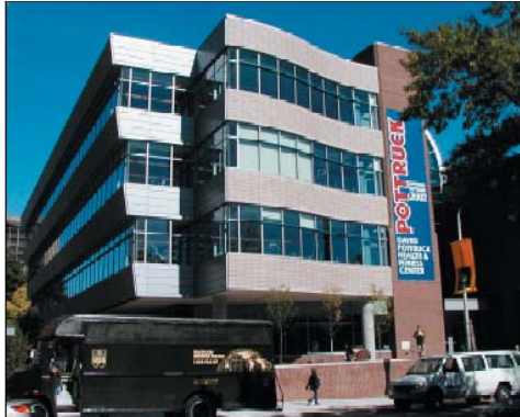
Five different façade materials were required in the enclosure of the David S. Pottruck Center, University of Pennsylvania
