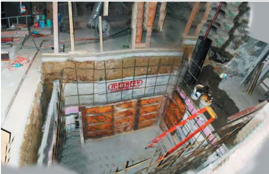
Construction of an elevator pit
