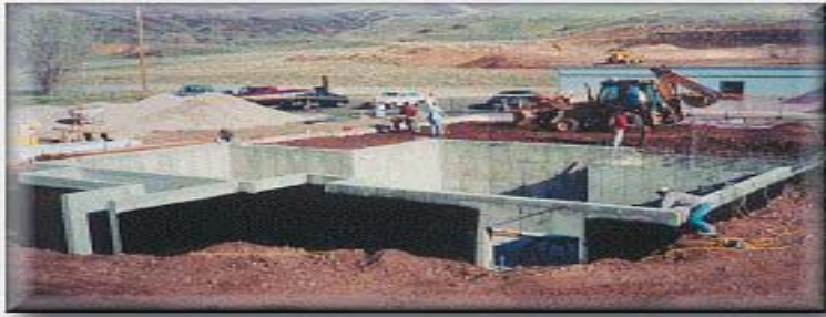
Foundation wall construction
