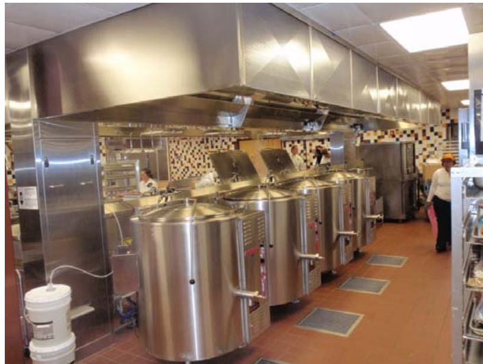
Building 18028 Main Kitchen – One Side of Hood 1.
