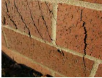
Improper Sealing (Source: http://cx.lbl.gov )
