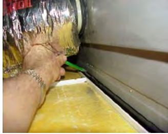
Duct Leakage (Source: http://cx.lbl.gov )
