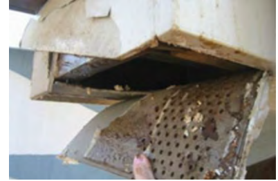
Building Envelope Moisture Entry (Source: http://cx.lbl.gov )
