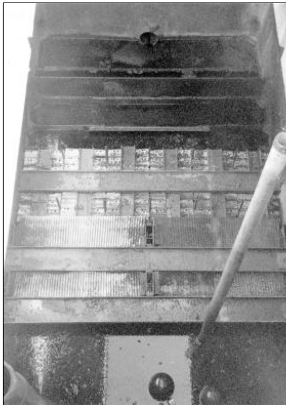
Figure 2. Oil/water separator at Building 3966, Fort Lewis.
