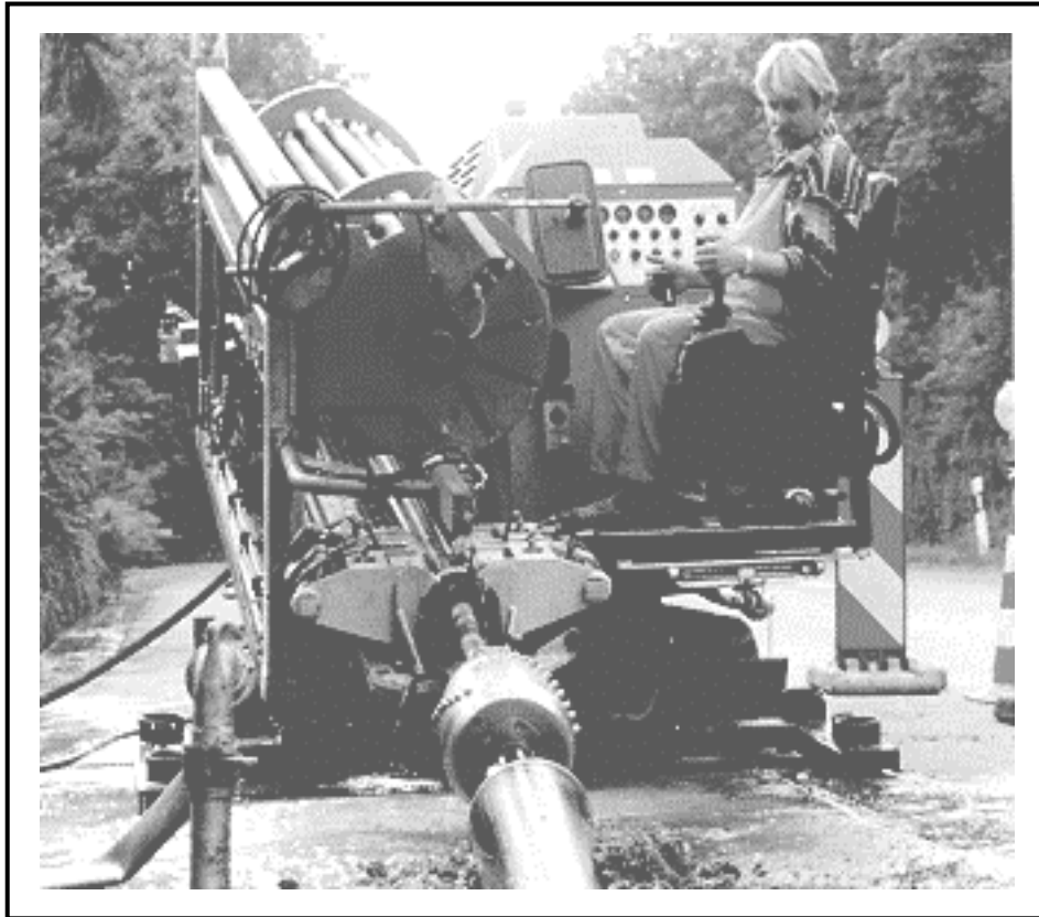
Figure 5. Directional Drill Rig.
