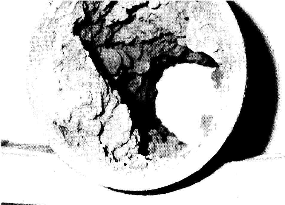
Figure 1. Heavily tuberculated unlined cast iron pipe.
