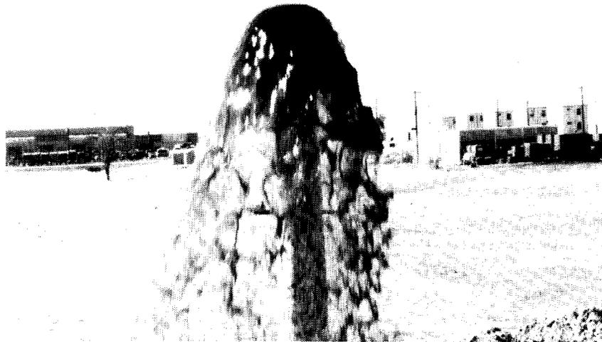
Figure 5. Discolored water as a result of pigging.
