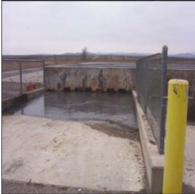
Figure A-1. Fort Sill waste receiving basin.
