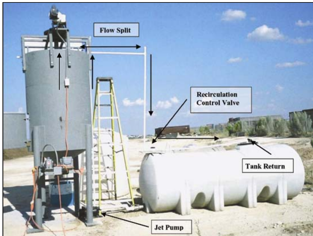
Figure A-6. Plumbing arrangement.
