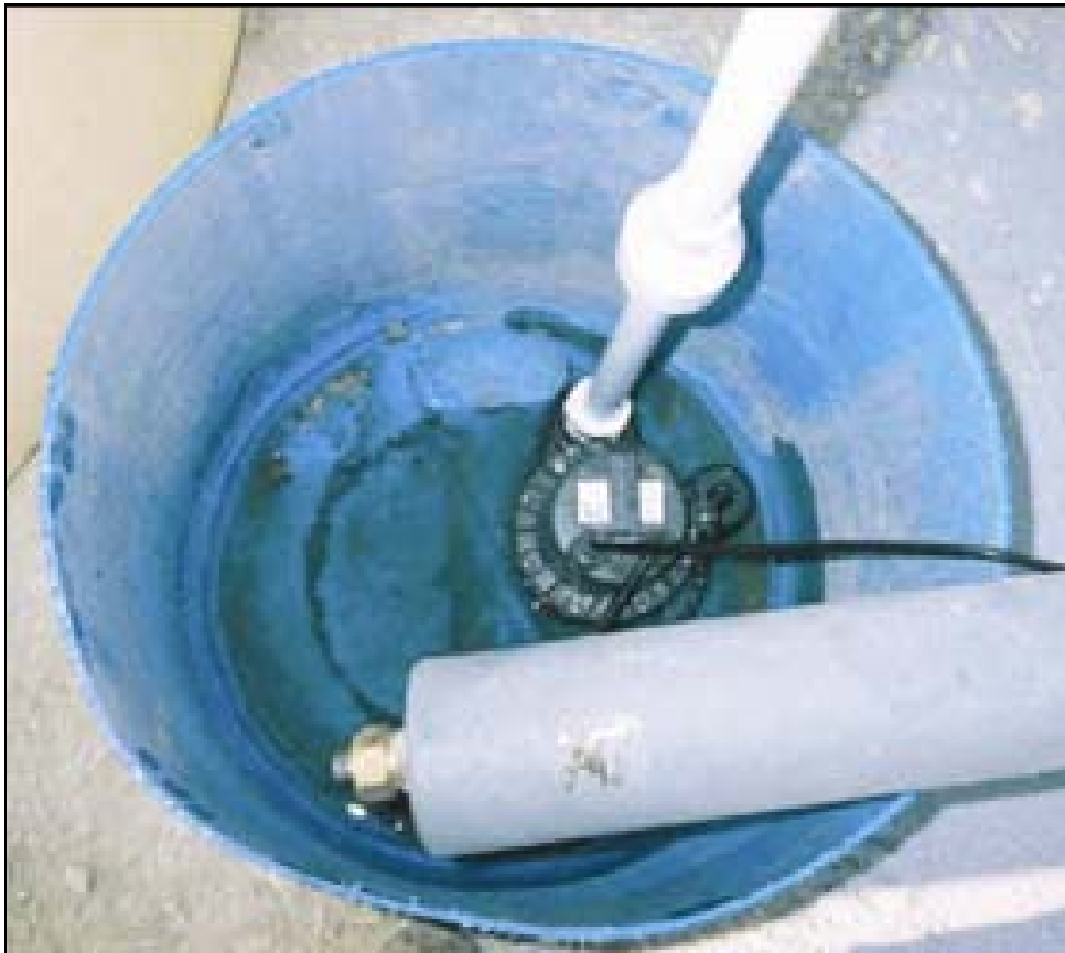
Figure A-17. Sump bucket arrangement.
