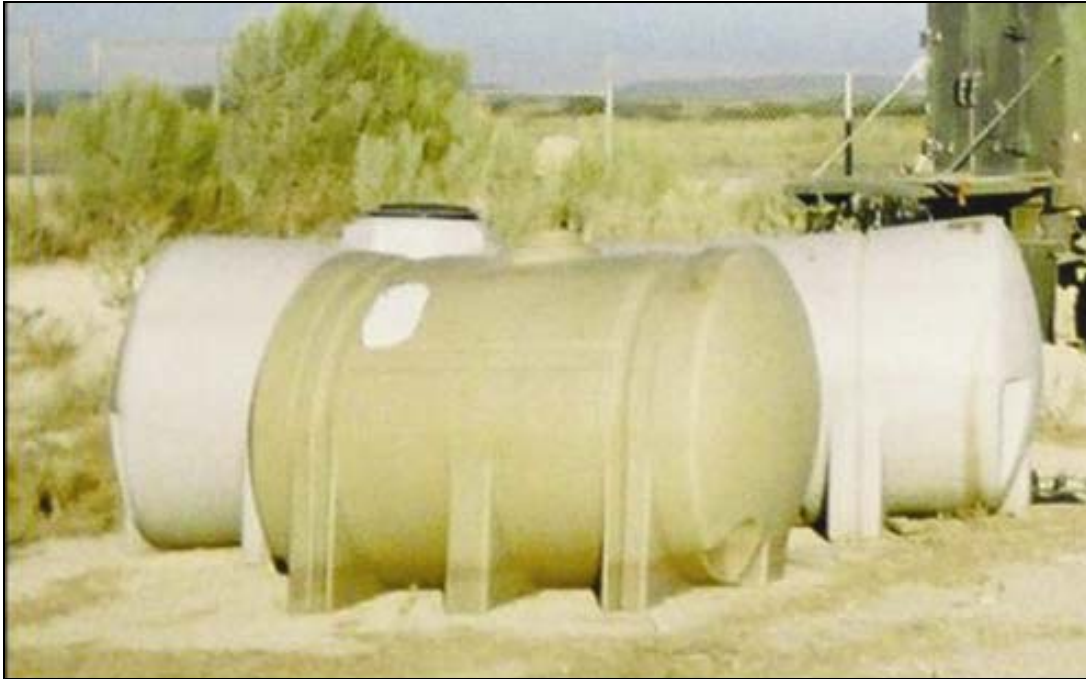
Figure A-4. Waste influent holding tanks from Fort Hood.
