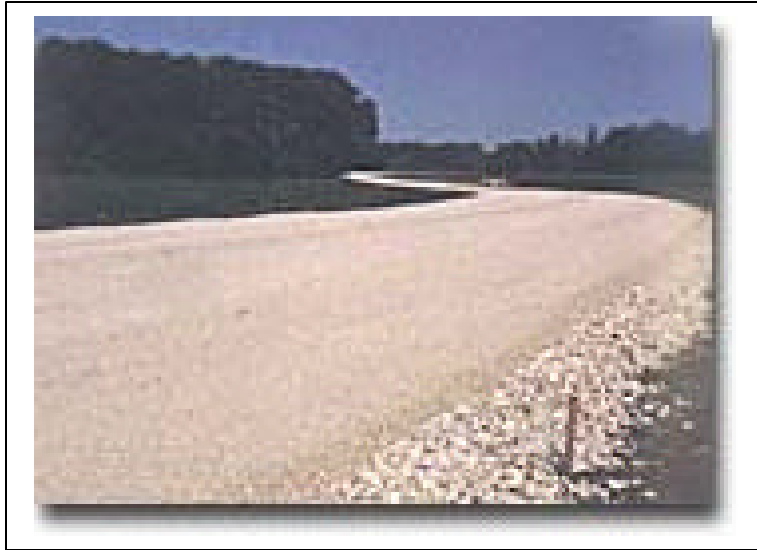
Figure 6. RCA Used for Granular Base.
