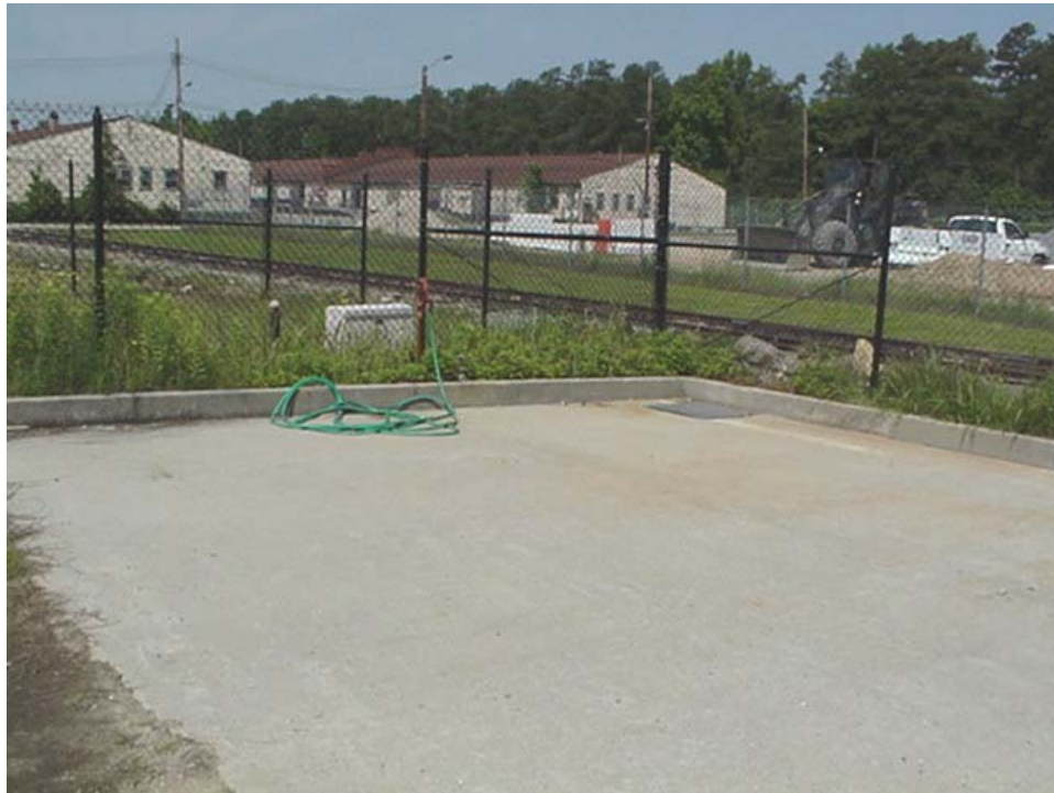
Figure 1 – Fort Lee, VA, washrack dedicated for use as a purging facility
