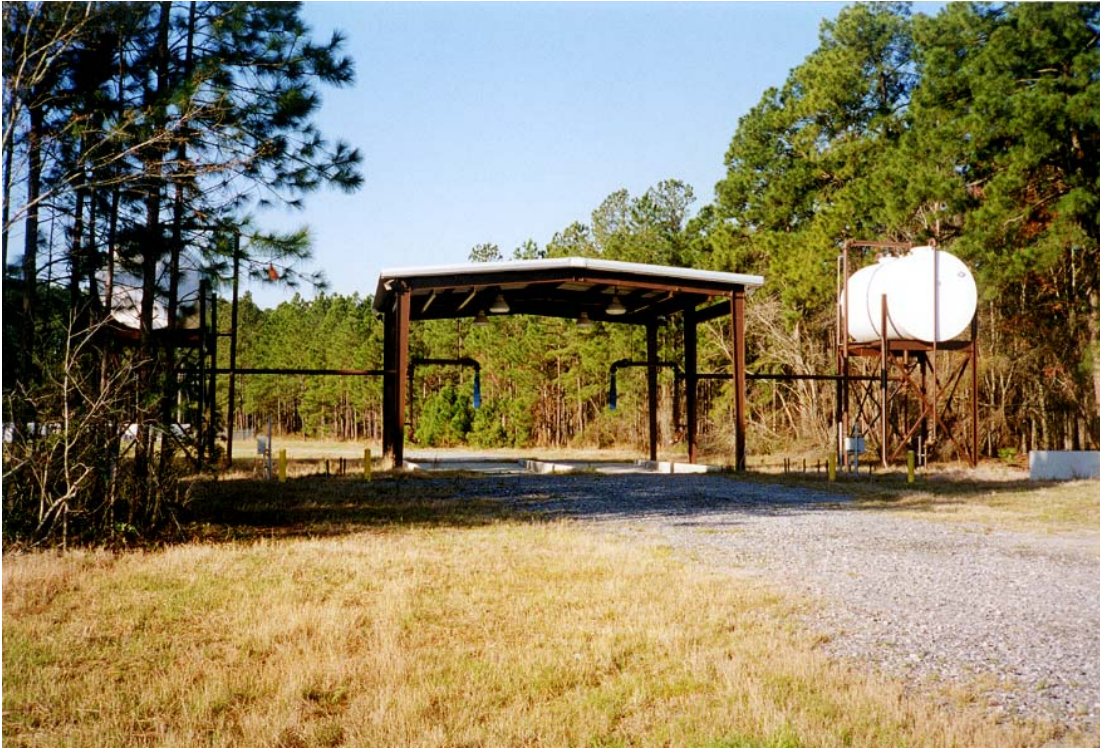
Figure 4 – Purging facility with recycle treatment and covered fill area
