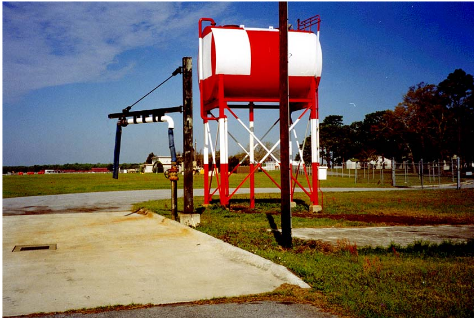
Figure 3 – Hunter Army Airfield purging facility
