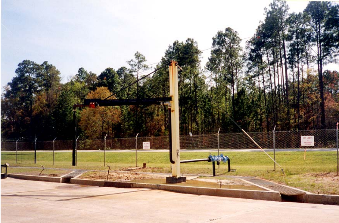
Figure 2 – Existing washrack modified to decrease fill times
