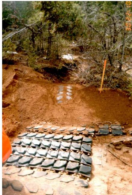
**Figure 6. Tank tracks lining a natural inlet.**
