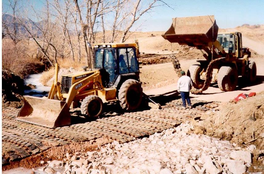
**Figure 16. Placing the tracks.**
