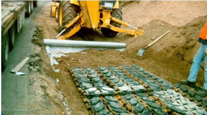
**Figure 3. A drainage channel lined with geotextile and tank tracks.**
