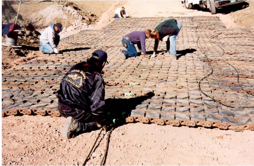
**Figure 18. Using cables to string the tracks together.**
