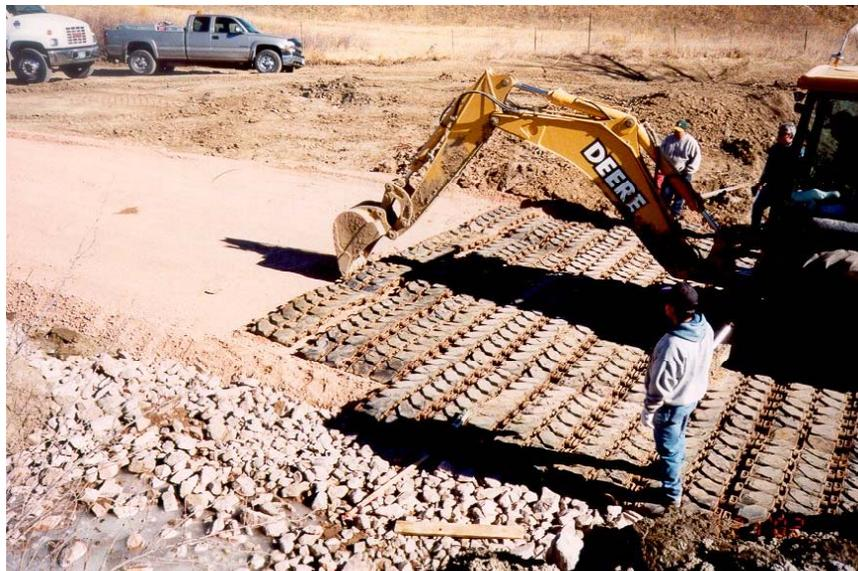
**Figure 17. Moving the tank tracks into final position.**
