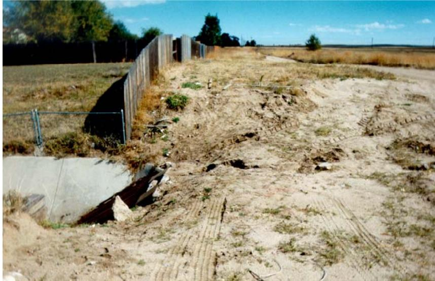
**Figure 1. Unstable culvert inlet.**
