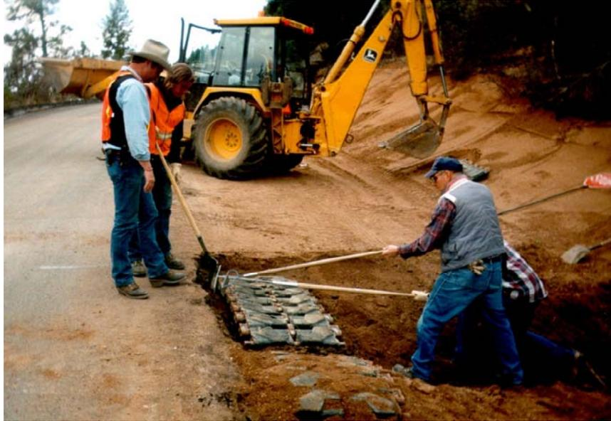
**Figure 7. Tracks toed into the soil profile under the waterflow line.**
