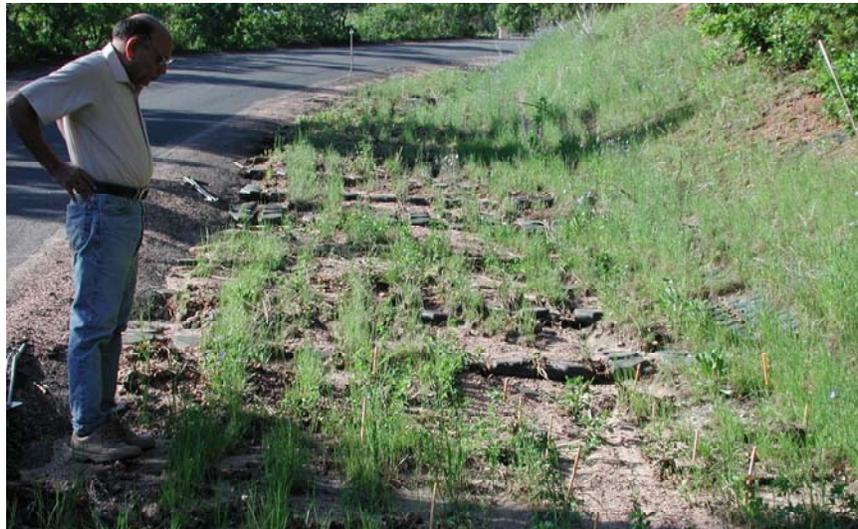
**Figure 10. The project area 2 years after tank tracks were placed.**
