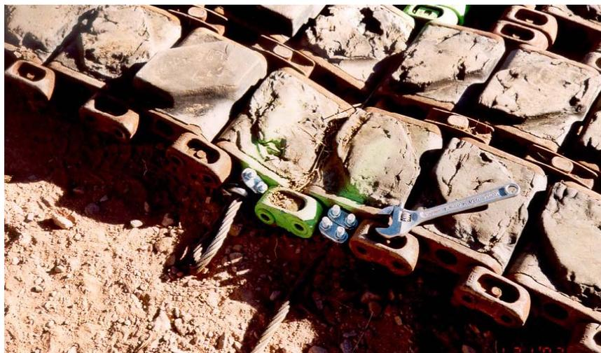
**Figure 19. Using clamps to secure the cables.**
