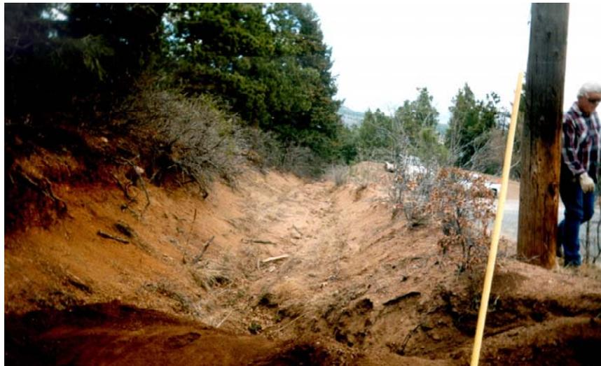
**Figure 8. Erosion and scouring downstream from the project site.**
