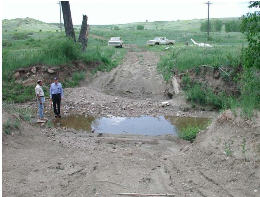
**Figure 11. Heavily trafficked tank trail crossing before hardening.**
