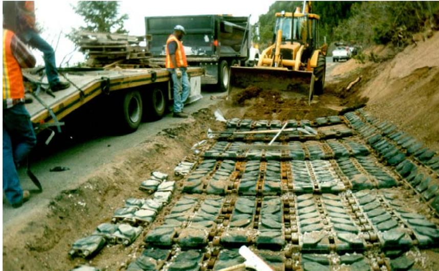
**Figure 5. Tracks toed under the adjacent roadway.**
