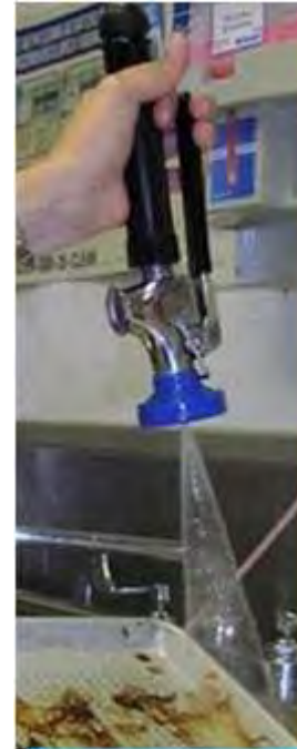
Figure A-18. High-efficiency pre-rinse spray valve (Scholze 2010).
