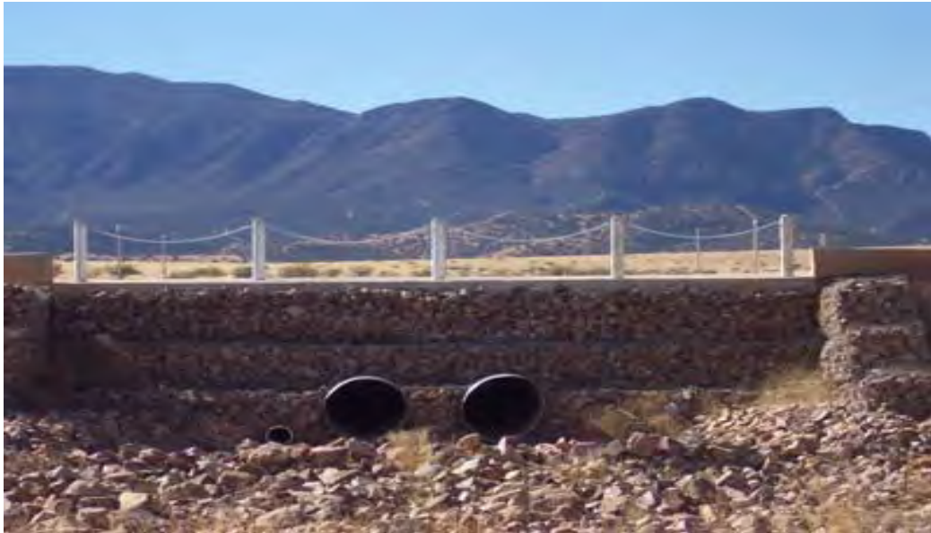
Figure A-22. Retention and infiltration to an aquifer at Fort Huachuca (Courtesy of Tom Runyon, Fort Huachuca).
