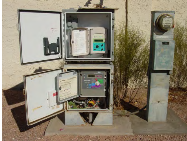
Figure A-7. A typical, newer style of irrigation control system that will conserve water (Scholze 2011a).
