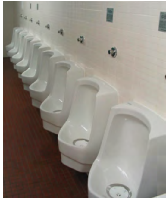
Figure A-12. Each waterless urinal can save tens of thousands of gallons of water per year (Scholze 2011a).
