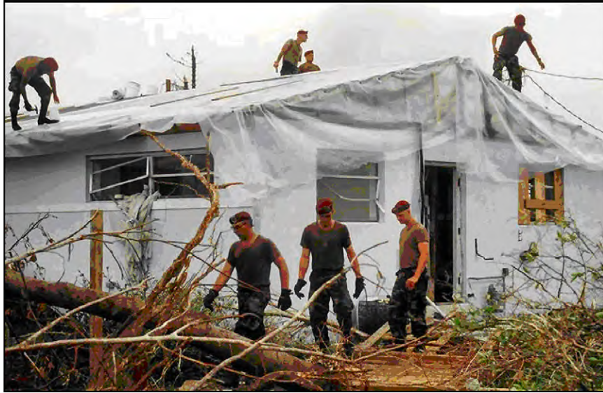
Figure 3.22. Using Plastic to Cover a Damaged Roof.
