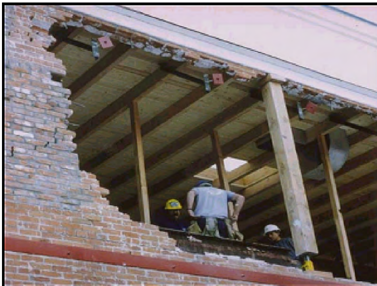
Figure 3.26. Damaged Brick Infill Wall.
