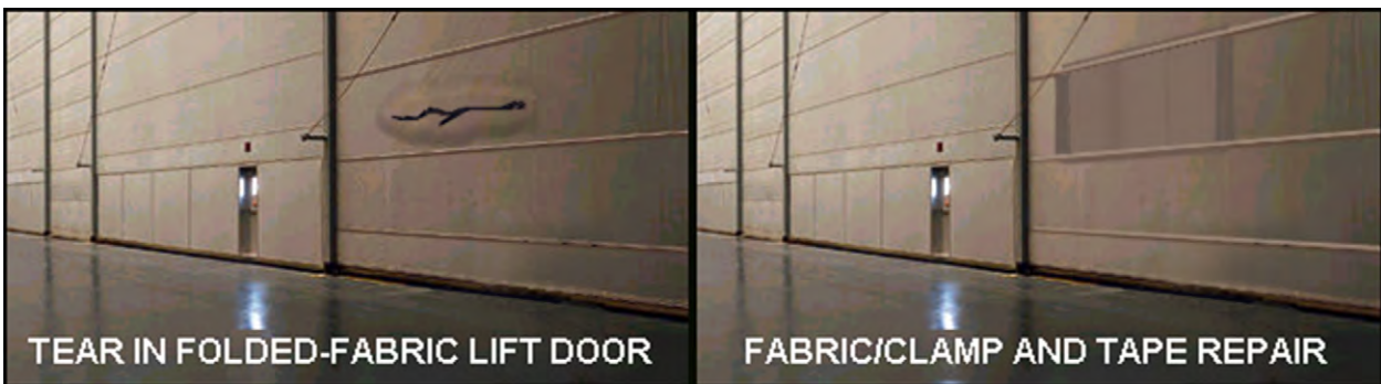
Figure 3.34. Typical Fabric Clamp Repair.
