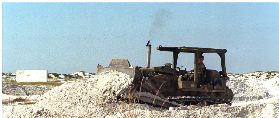
Figure 7.8. Cutting a Sand Dike for a Fuel Bladder.
