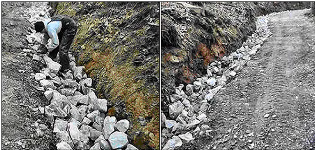
Figure 2.29. Riprap-Lined Drainage Ditches.
