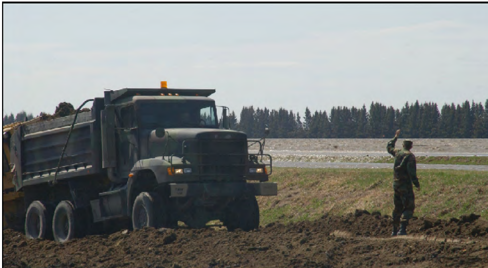
Figure 7.12. Earthen Dike Being Constructed to Control Flood Waters.
