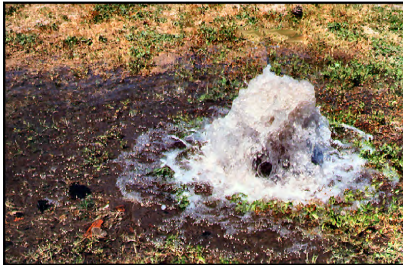
Figure 4.1. Obvious Water Line Break.
