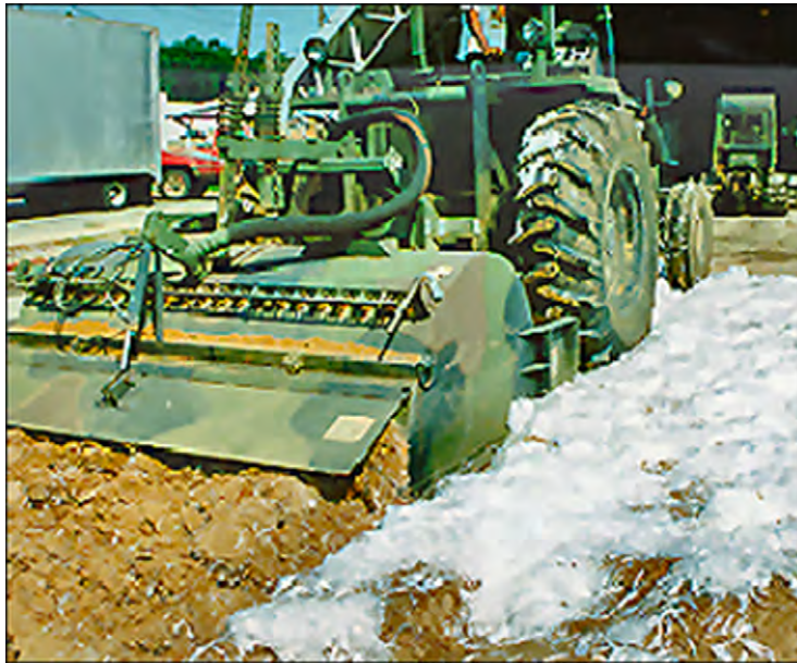
Figure 2.10. Blending Fibers With Soil.
