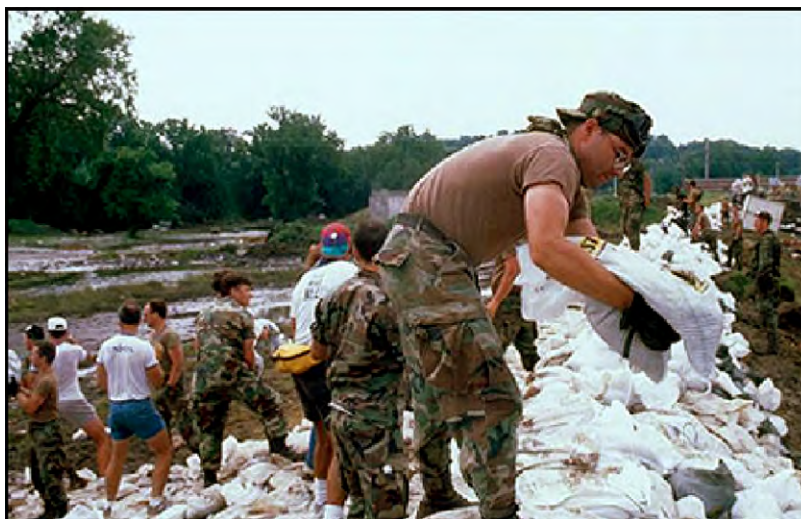
Figure 7.13. Personnel Constructing Sandbag Levee.
