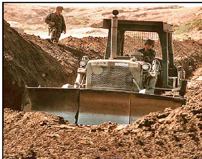
Figure 7.1. Berm Construction During Desert Operations.
