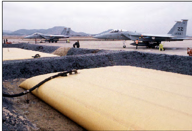
Figure 7.7. Dikes Placed Around Fuel Bladders.
