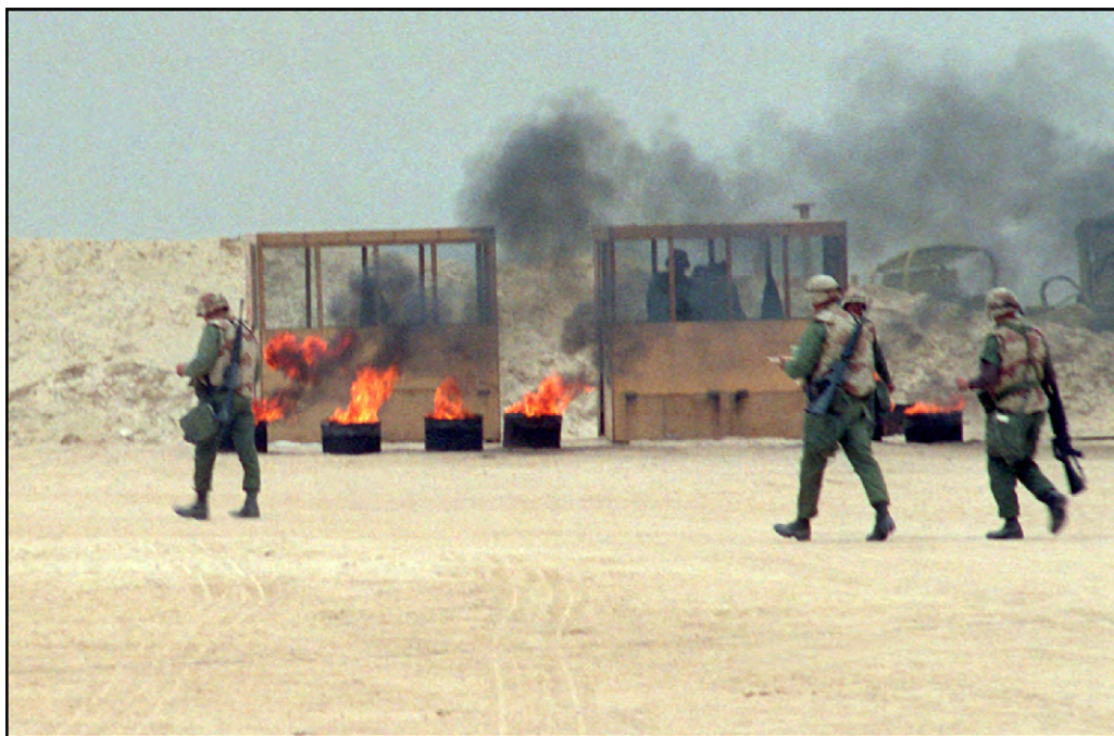
Figure 6.9. Multiple-Station Burn Out Latrines.
