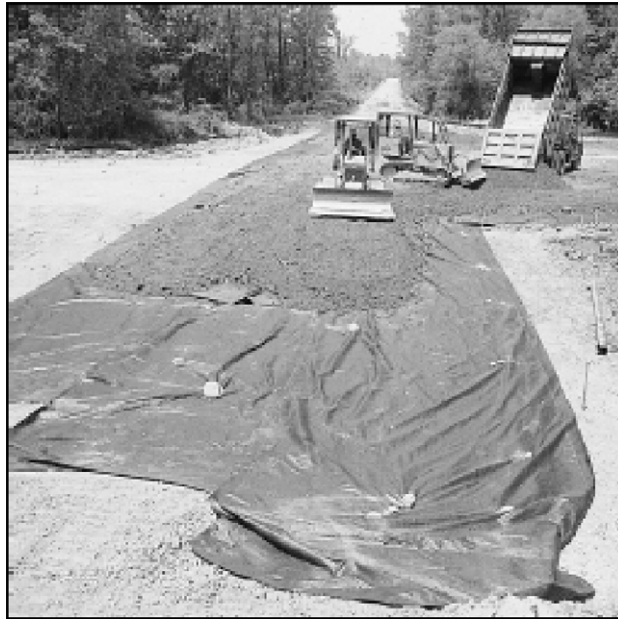
Figure 2.11. Using Geotextile During Road Construction.
