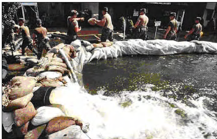
Figure 7.14. Poly Sheeting and Sandbags Reduce Water Absorption.
