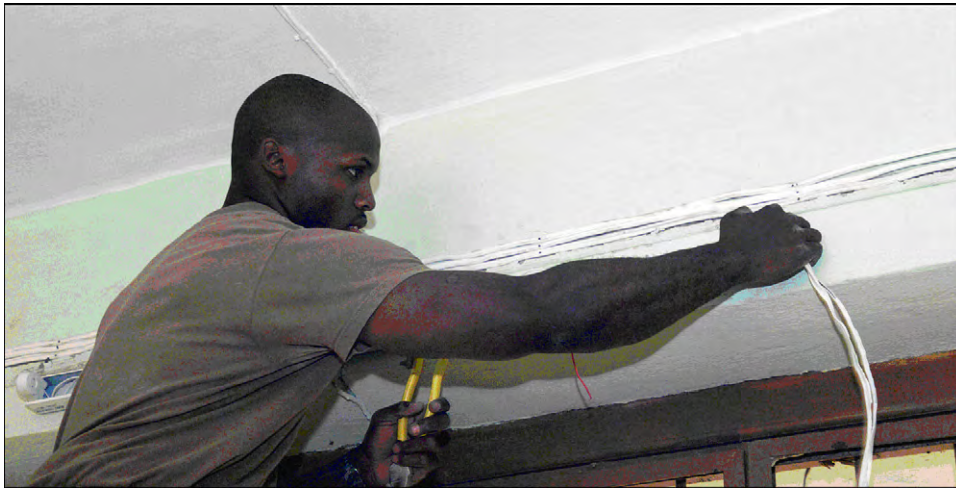
Figure 5.19. Installation of Temporary Interior Wiring.
