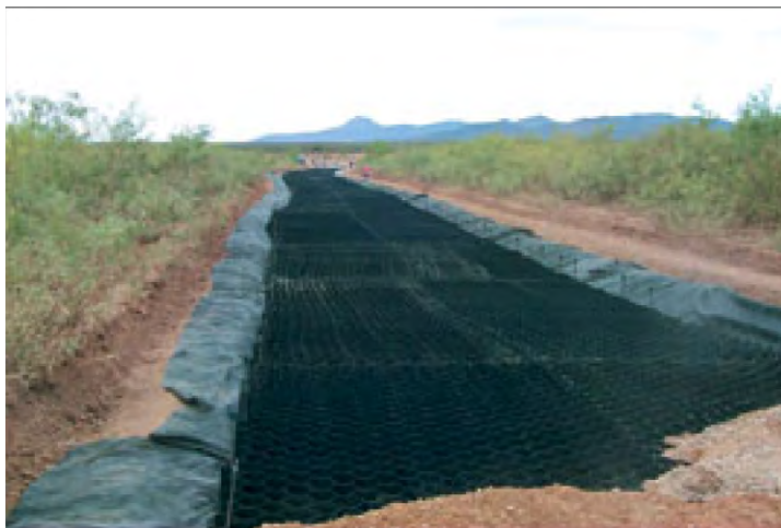
Figure 2.3. Sand-Grid Road Construction.
