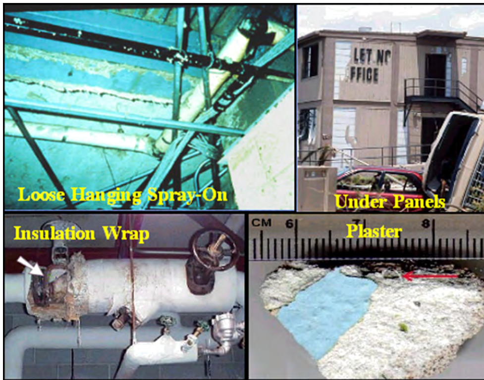
Figure 3.3. Examples of Asbestos Use in Construction.
