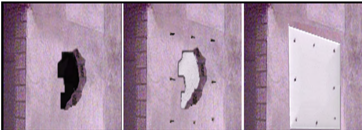
Figure 3.30. Masonry Wall Confining Sequence.
