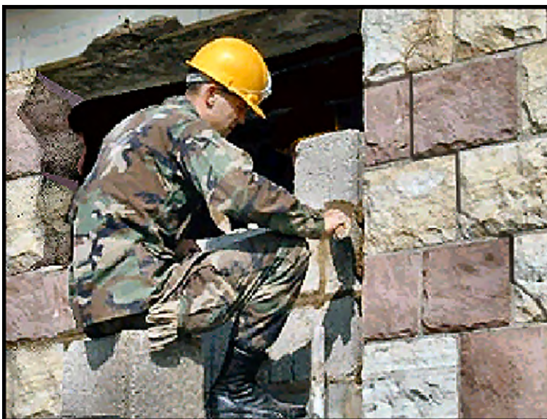
Figure 3.27. Correcting Damage With New Material.
