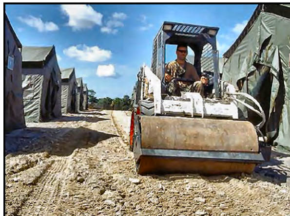
Figure 2.9. Stabilizing a Tent Area in French Guinea.
