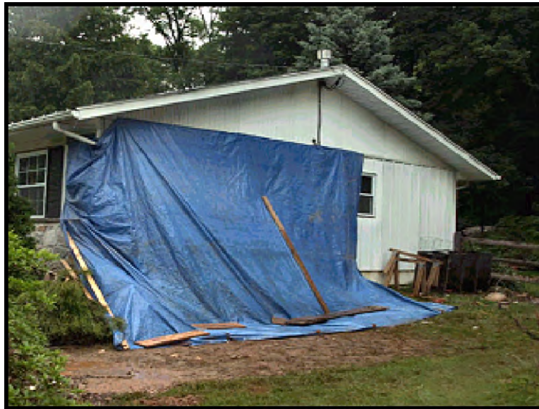
Figure 3.23. Temporary Tarpaulin Protection.
