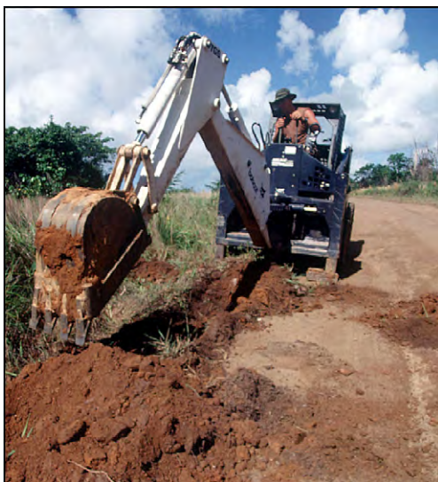
Figure 7.19. Creating a Drainage Ditch to Enhance Water Runoff.
