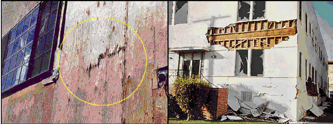
Figure 3.25. Examples of Sheathing Damage.
