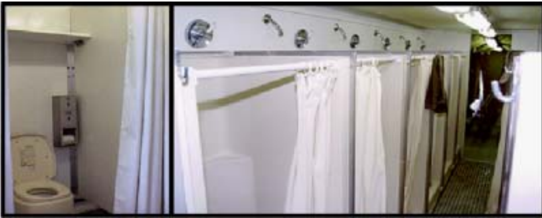
Figure 3.5. Force Provider Containerized Latrine and Shower Facilities.
