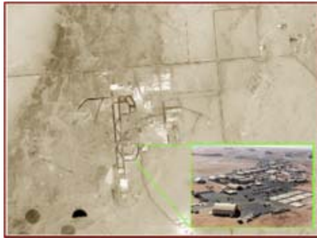
Figure 5.2. PSAB Airbase (Before and After Buildup).
