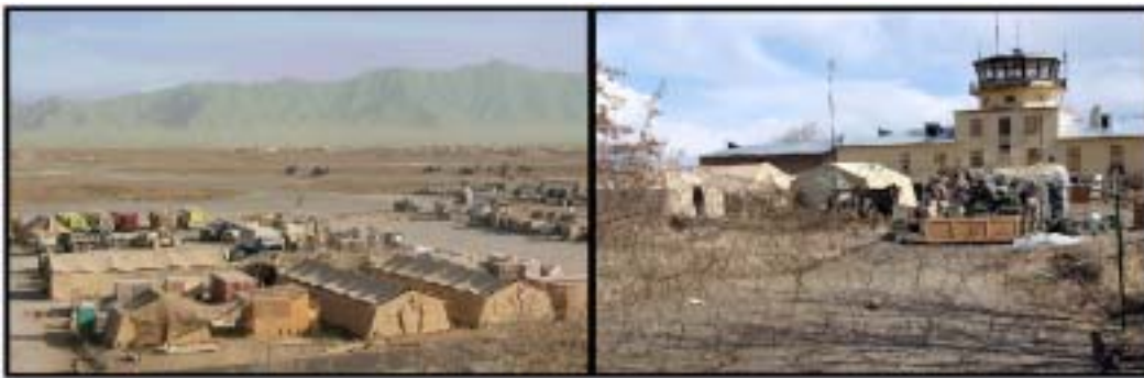
Figure 2.3. Initial Construction Standard at FOB in Afghanistan.
