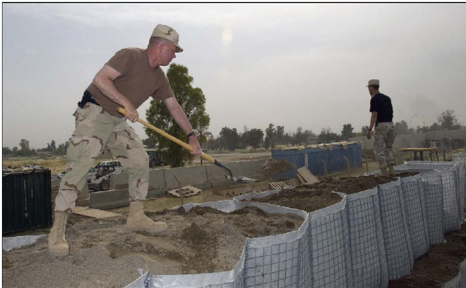
Figure 3.18. Engineers Fill HESCO Barrier Revetment With Soil.
