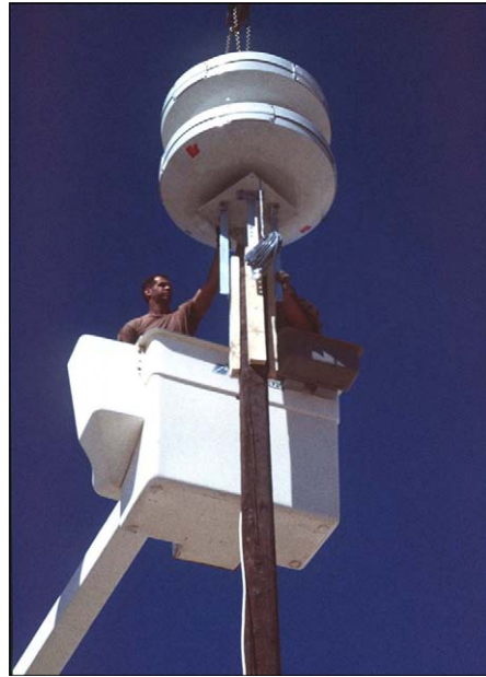
Figure 4.1. Engineers Install Giant Voice System at Deployed Location.
