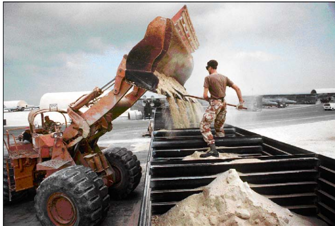
Figure 3.5. Engineers Build Aircraft Shelters from B-1 Steel Revetment Kits.
