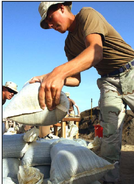
Figure 3.25. Airmen Use Sandbags to Enhance Shelter Survivability.
