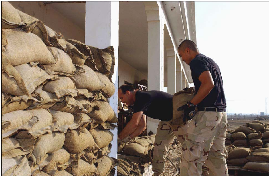
Figure 3.13. Fortifying Shelter with Sandbags.
