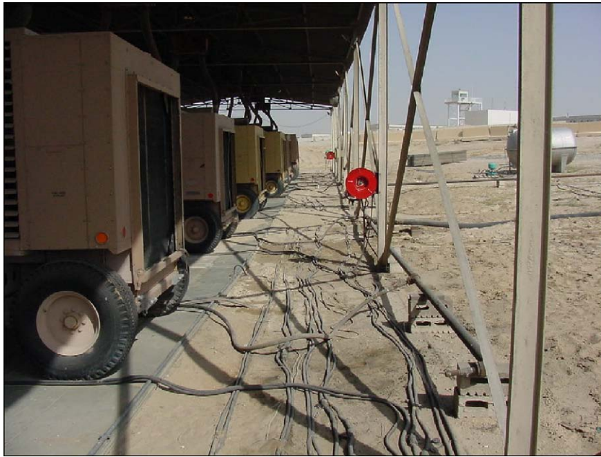
Figure 6.5. Sheltered Generators.
