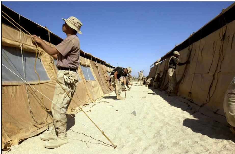
Figure 2.1. Services Squadron Personnel Erect Modular Tent in Iraq.
