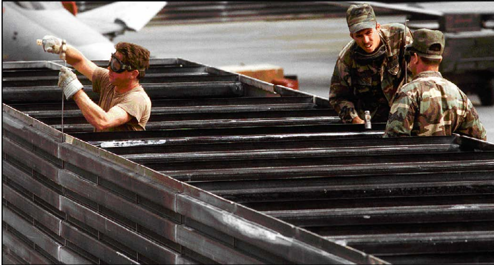
Figure 3.18. Engineers Fill HESCO Barrier Revetment With Soil.
