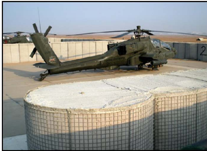
Figure 3.6. HESCO Barriers Provide Limited Shelter for Aircraft.
