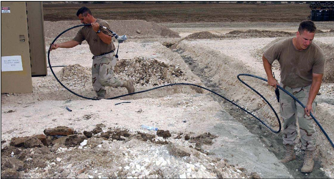
Figure 6.4. Engineers Lay Out Power Cables at Forward Operating Location.
