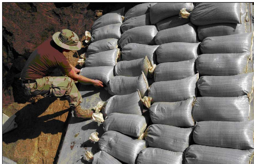
Figure 6.3. Sandbagging Overhead Cover of a Bare Base Shelter.
