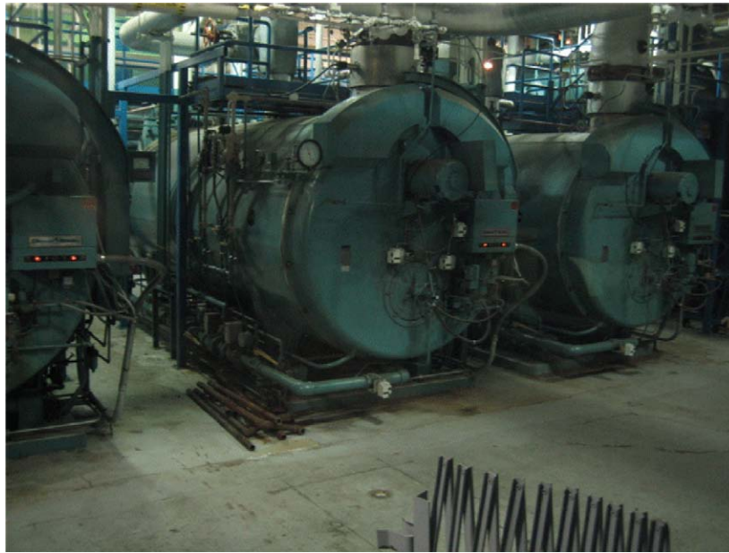
Figure 5.7. Central Heating System.
