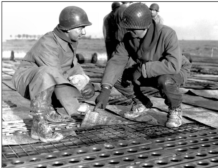
Figure A4.9. "Sandwich" Runway Surface.
