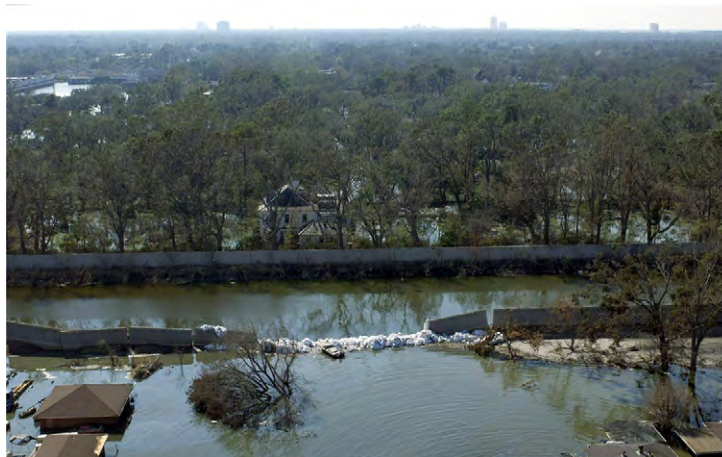
Figure 1.4. Levee Breach in New Orleans Caused by Hurricane Katrina.
