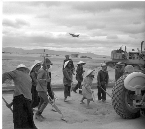
Figure A4.22. Vietnamese Civilians Helping Build Tuy Hoa Parallel Runway.
