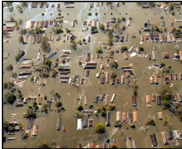
Figure 1.9. Flooded Homes in New Orleans After Hurricane Katrina.
