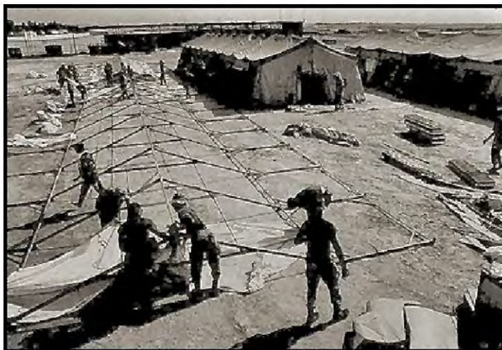
Figure A4.23. Erecting a TEMPER Tent (Operation DESERT STORM).
