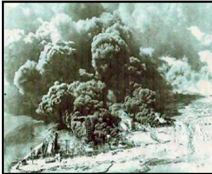
Figure 1.21. Explosion of the SS Grand Camp, Texas City, Texas 1947.
