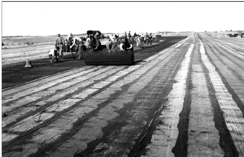
Figure A4.8. Square Mesh Track Being Unrolled on Top of Hessian Matting.
