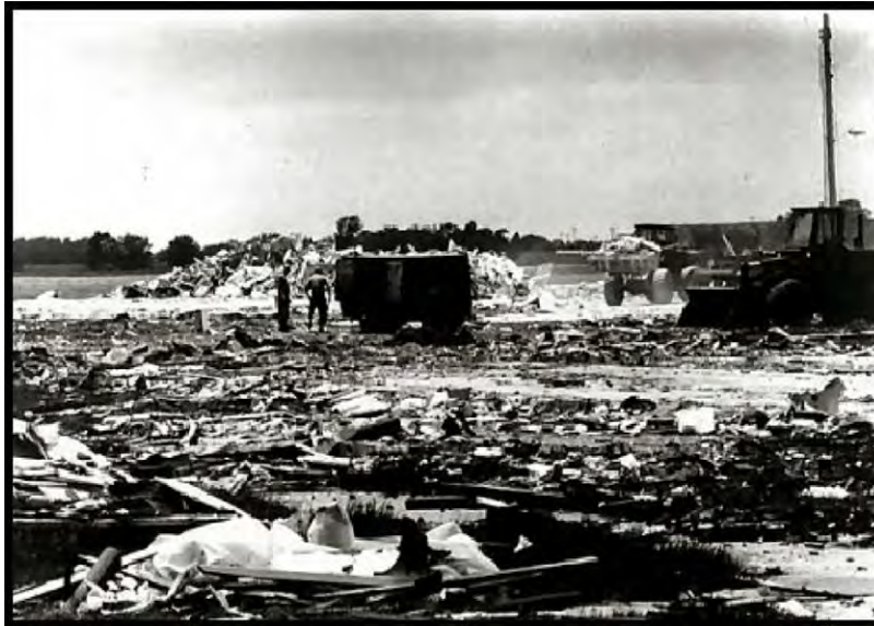
Figure 1.14. Aftermath of Explosion at Industrial Plant.
