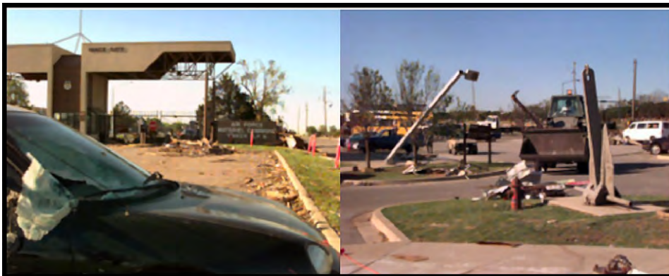
Figure 1.6. Tornado Damage at McConnell AFB, April 1991.
