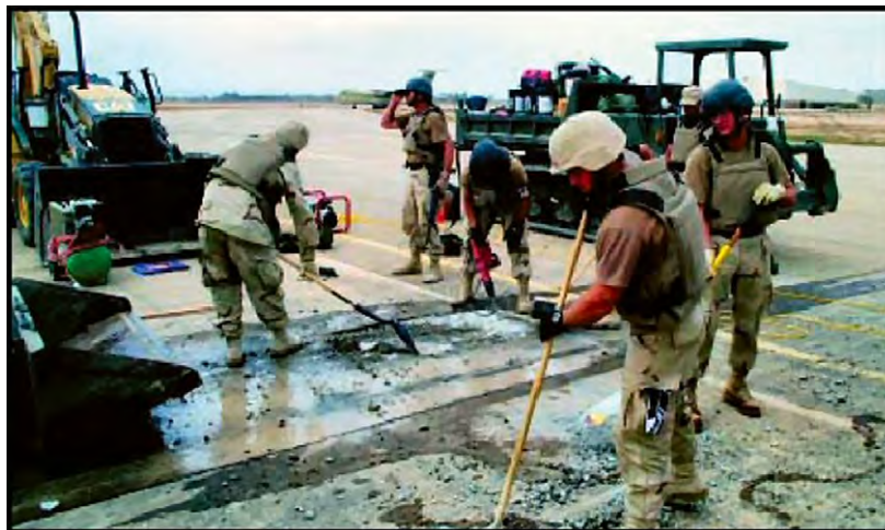
Figure A4.30. Engineers Repairing Runway in Southwest Asia.
