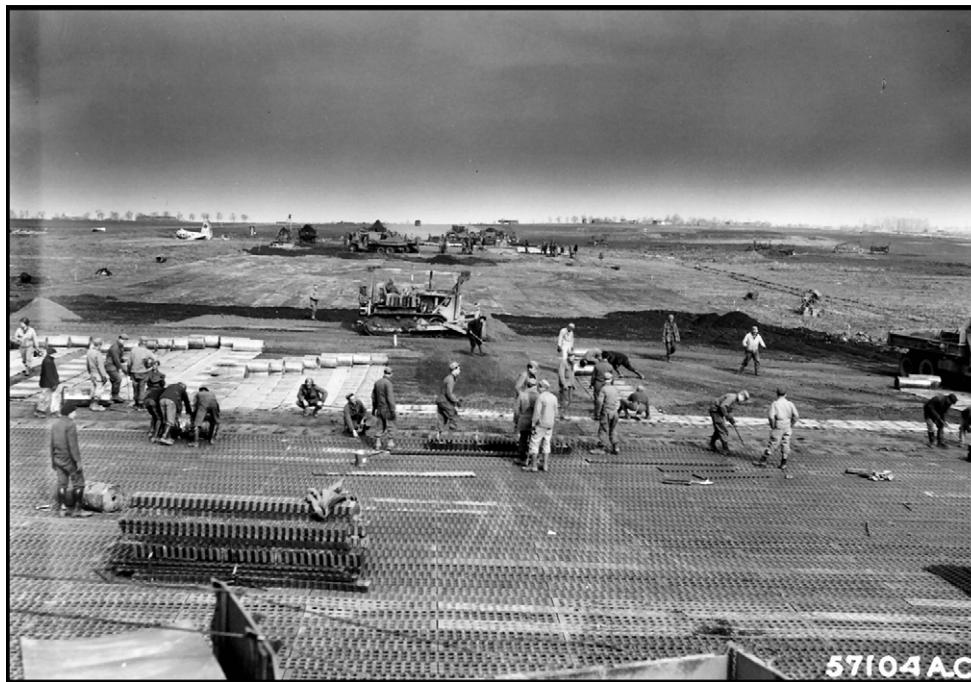
Figure A4.10. Assault Airfield Nearing Completion—Started From Each End.
