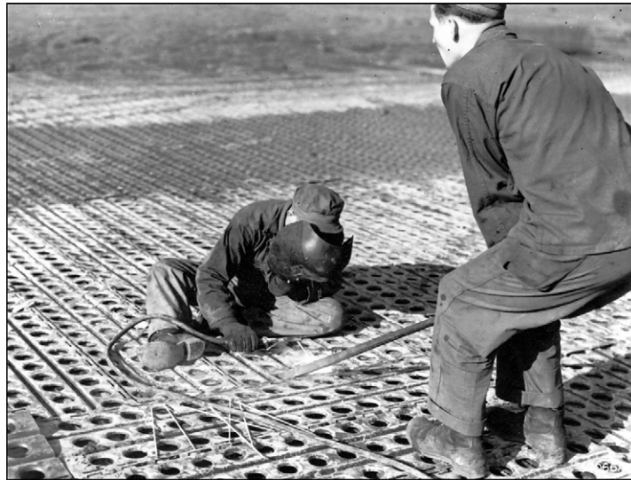
Figure A4.15. Damaged PSP Being Repaired.
