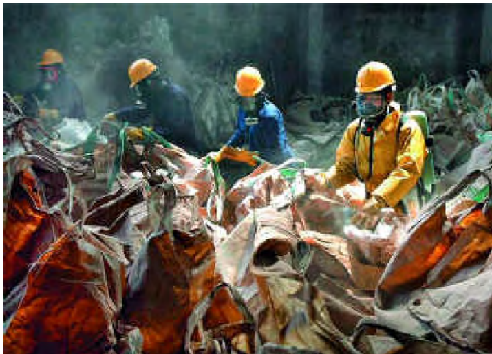
Figure 1.15. Clean Up After Union Carbide Plant Gas Leak in India.
