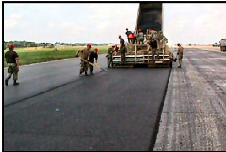
Figure A4.29. RED HORSE Taxiway Repair Work, Taszar Hungary.
