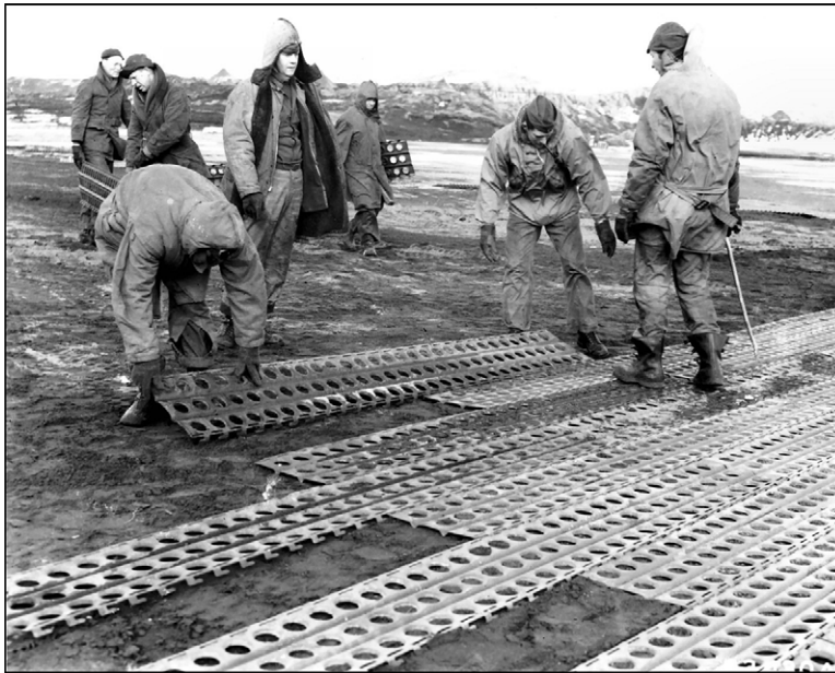
Figure A4.6. Engineers Laying Pierced Steel Planking.
