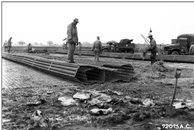
Figure A4.1. Constructing Expedient Airfields During WWII.
