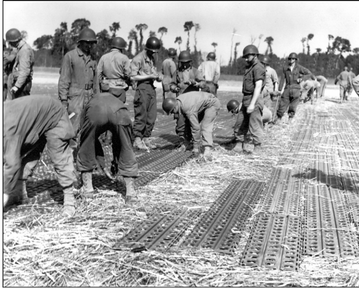
Figure A4.7. Using Straw Under PSP to Control Dust.
