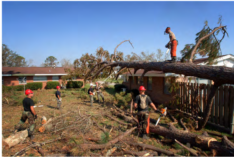
Figure 3.1. Engineers Conduct Hurricane Katrina Recovery Operations at Keesler AFB.
