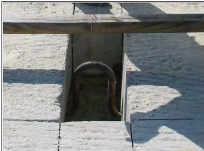
Figure 13. Hat-Type Tie-Down Prior to Concrete Placement.
