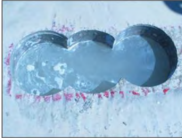
Figure 17. Three Adjacent 12-Inch (0.3-m) Cores Allow for Insertion of the Hat-Type Tie-Down.
