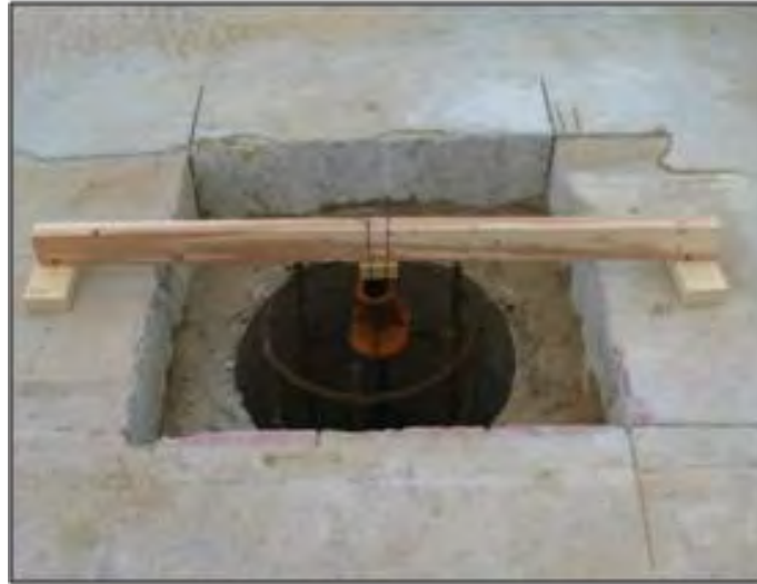
Figure 8. Neenah Anchor With 8-Foot (2.4-m) Pier Prior to Concrete Placement.
