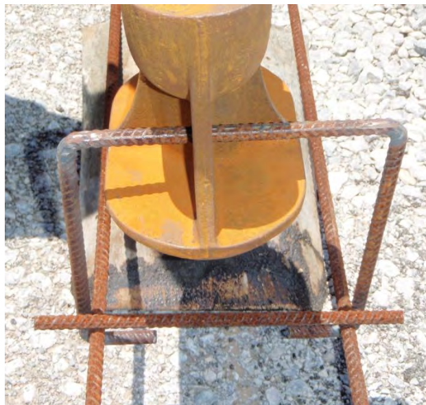
Figure 9. Neenah With Bent Rebar for Installation in HMA Pavement With Minimum 12-Inch (305-mm) -Thick PCC Underlay.
