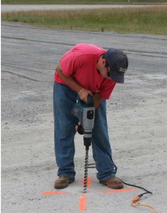
**Figure 2. Drilling Through the Overlying Stabilized Surface**
