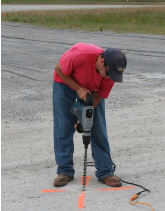
Figure 2. Drilling Through the Overlying Stabilized Surface
