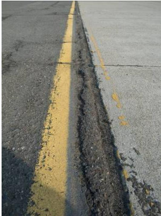
**Figure 7. Example of Low Reactivity ASR at Travis AFB.** Cracking is generally tight, with minor FOD issues in this pavement that is over 25 years old. Small volume change has caused minor upheaving of the AC shoulder. The only maintenance on this ramp has been sweeping to minimize the hazard cause by the slow generation of FOD.
