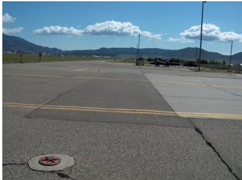
**Figure 6. Examples of Large Volume Changes Suggesting Highly Reactive ASR Pavements.** On the left, two pavement slabs are displaced by several inches. On the right, the PCC has grown from the visible joint in the AC and damaged the adjacent pavement. An AC repair patch to the damaged AC from this growth is visible to the left of the PCC.
