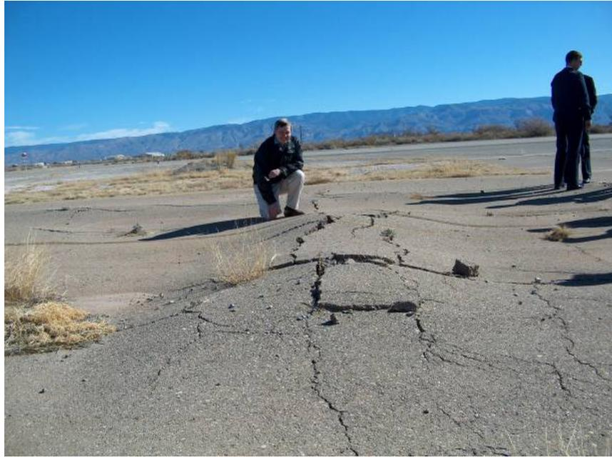
**Figure 2. Example of Localized Heaving in a Flexible Pavement Caused by Volume Change in the Underlying Base Course**
