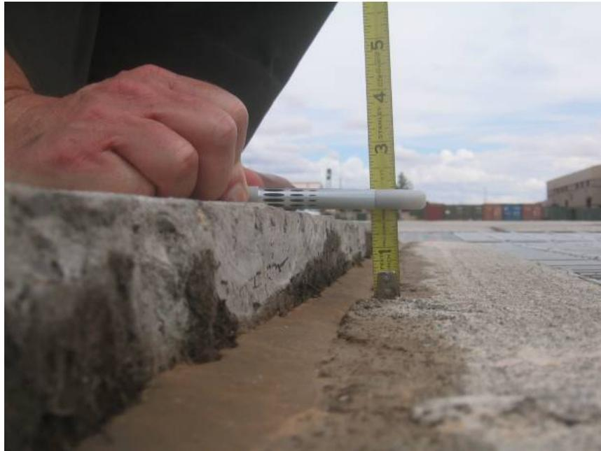
**Figure 1. Example of Differential Heaving on a Rigid Pavement Caused by Volume Change in Underlying Base and Fill Layers**
