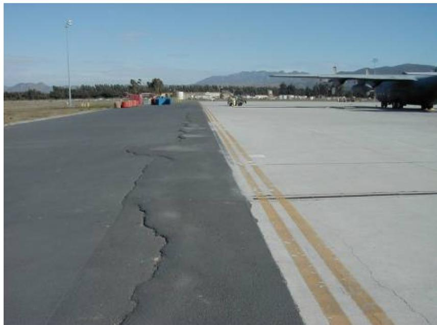
**Figure 5. Examples of Damage to Adjacent Asphalt from ASR-Induced Expansion in Adjacent PCC Pavement.** This suggests of a highly reactive pavement.
