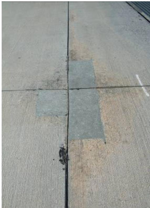
**Figure 4. Minor ASR Cracking in 5-Year-Old Pavement (Left Photograph); Patching Needed 3 Years Later (Right Photograph).** Because of the early development of ASR symptoms in this Holloman AFB pavement, it would be considered a highly reactive pavement.
