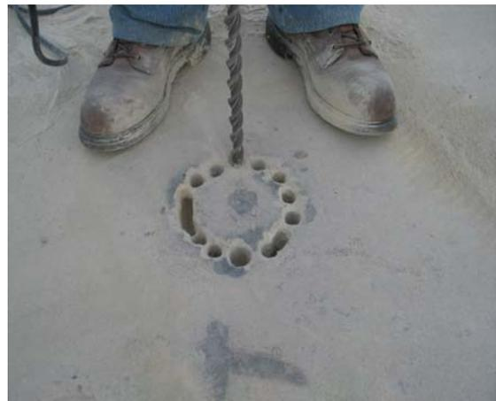
**Figure 8. Drilling Anchor Hole Perimeter**
