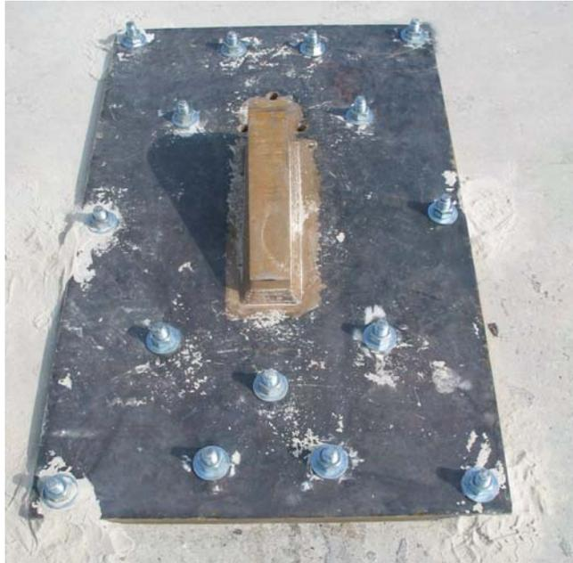
**Figure 14. Completed Anchor Plate**
