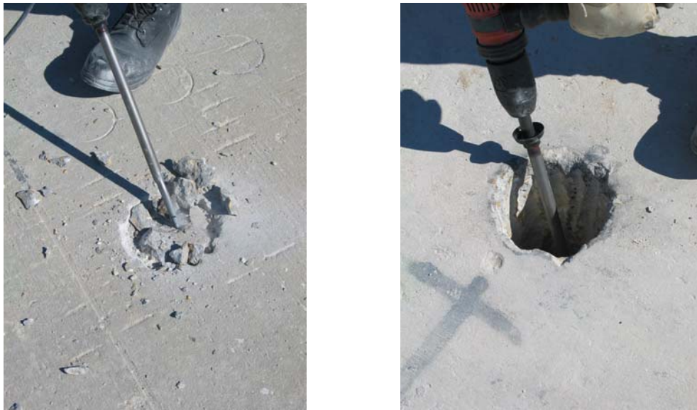
Figure 9. Chiseling Anchor Hole
