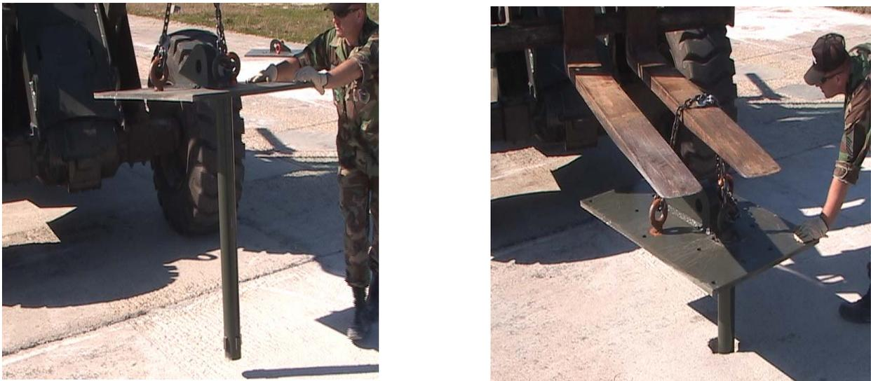
**Figure 11. Lowering the Expedient Anchor Plate into the Hole**
