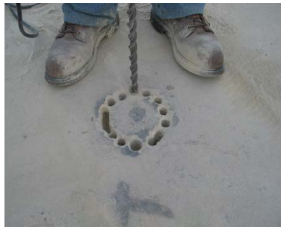
Figure 8. Drilling Anchor Hole Perimeter
