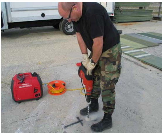
Figure 8. Drilling Anchor Hole Perimeter
