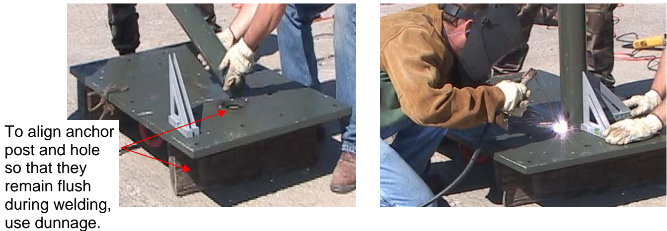
Figure 10. Welding Anchor Post to Anchor Plate
