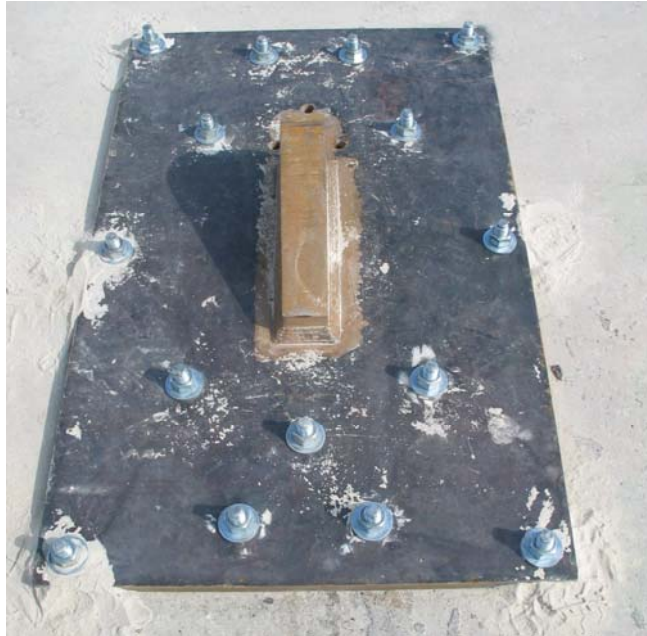
Figure 14. Completed Anchor Plate
