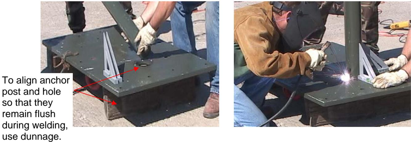
**Figure 10. Welding Anchor Post to Anchor Plate**
