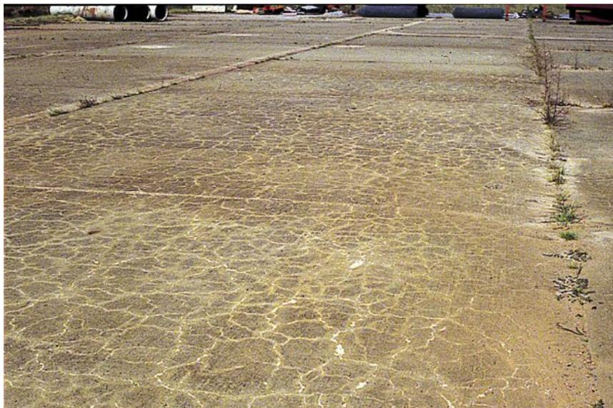
**Figure 4. ASR-induced Cracking in Ramp at Tinker AFB.** Note cracks are random (without the preferential longitudinal orientation seen in Figures 1 and 2) and continue across joints.
