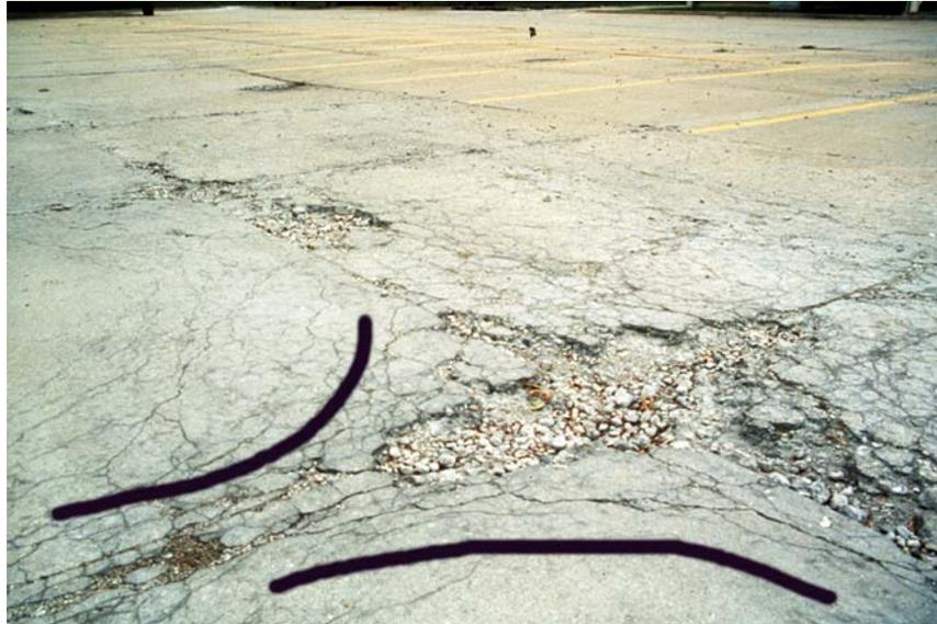
**Figure 6. D-cracking at Grissom AFB (Not to be Confused with ASR-induced Cracking).** Note general C-shape of cracks that are roughly asymptotic to joints and that do not cross transverse joints as seen in Figures 2 and 3.
