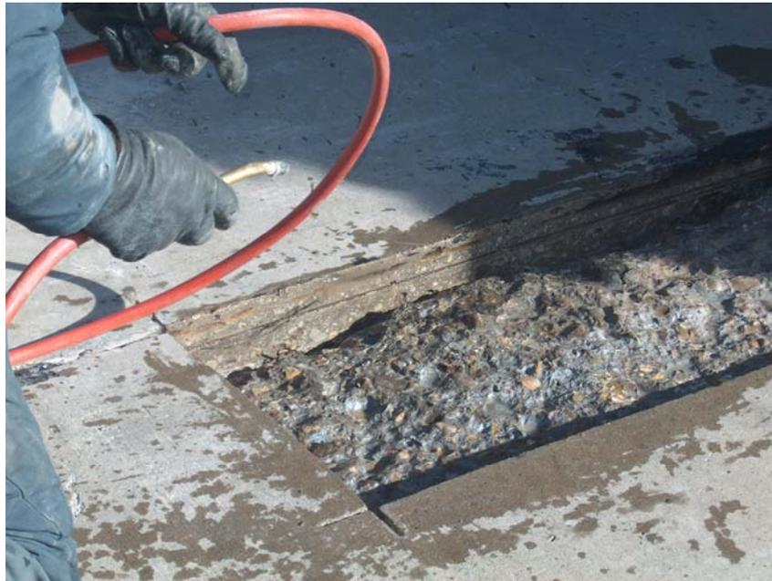
**Figure 11. ASR Gel—Appearing as Light, Hazy Coating on Shallow Patching Repairs at Holloman AFB—Was Impossible to Remove and Caused Many Patch Bond Failures.**
