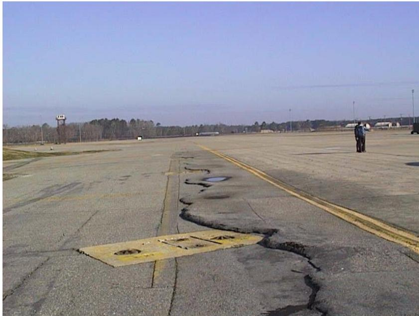
**Figure 8. Asphalt Shoulder Heaving Caused by ASR Expansion in Adjacent Concrete at Seymour-Johnson AFB.**
