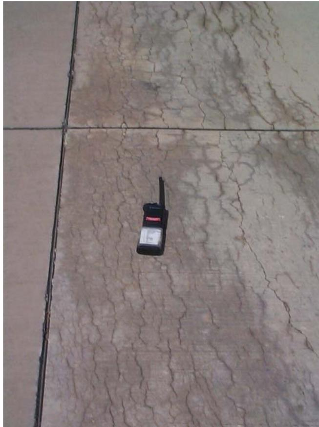
**Figure 2. ASR-induced Cracking on Taxiway, Holloman AFB.** Note cracks are preferentially longitudinal and continue across transverse joints.
