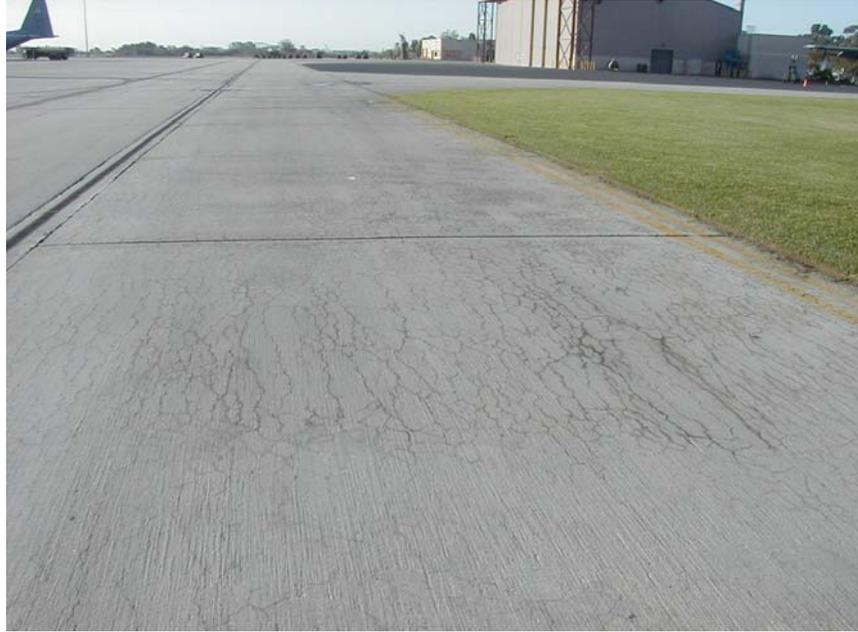
**Figure 3. ASR-induced Cracking in Taxiway at Channel Island ANG Facility.** Note cracks are preferentially longitudinal and continue across transverse joints.
