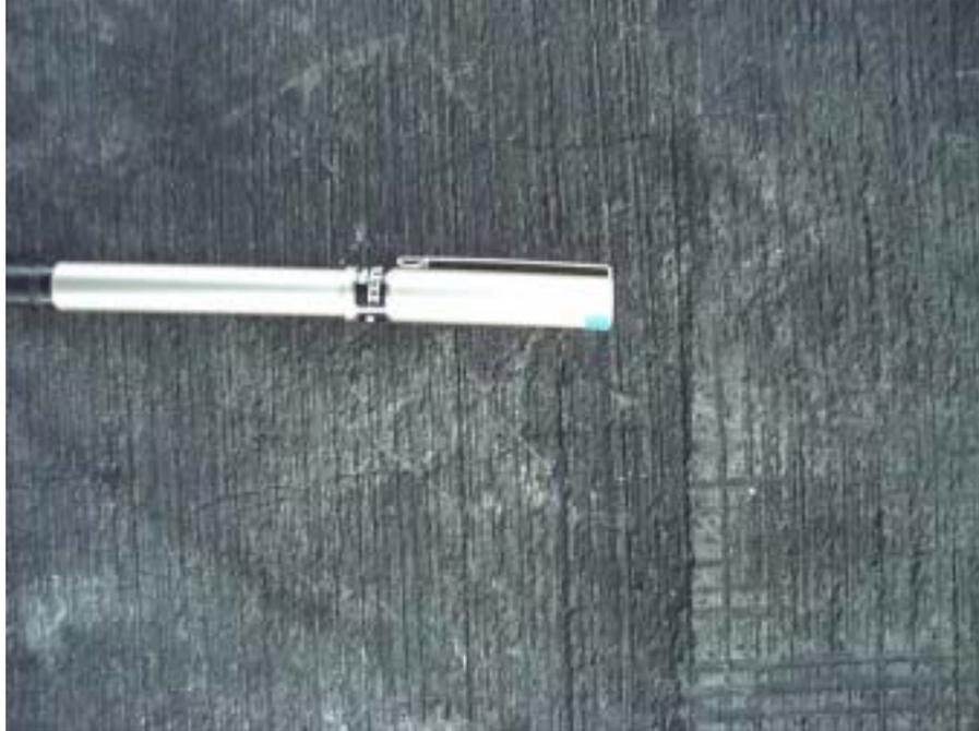
**Figure A1.5. Spot 2 Shrinkage Cracks**
