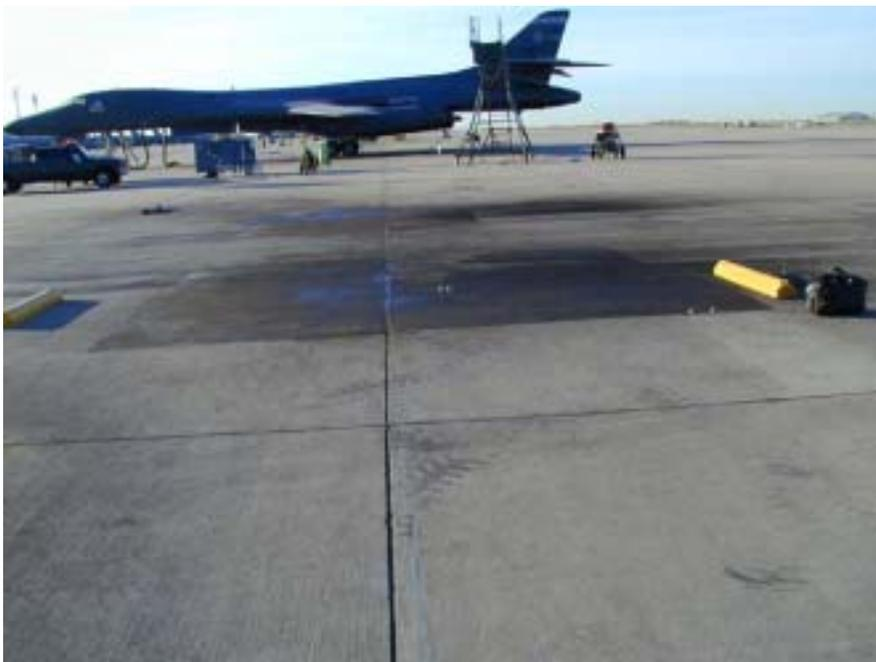
**Figure A1.2. Pad B10 Soaked with Hydraulic and Turbine Fluid**
