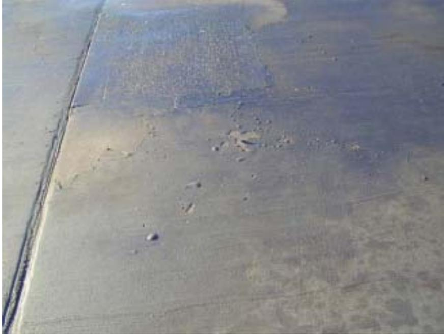
**Figure A1.3. Pad B11 Joint, Showing Delamination and Blistering**
