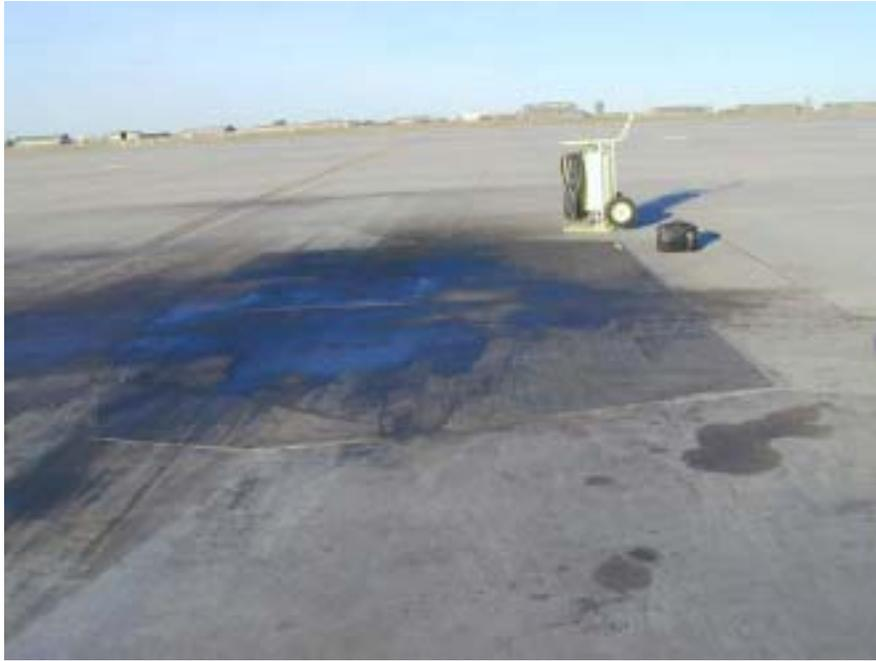
**Figure A1.1. Pad B11 Soaked with Hydraulic and Turbine Fluid**
