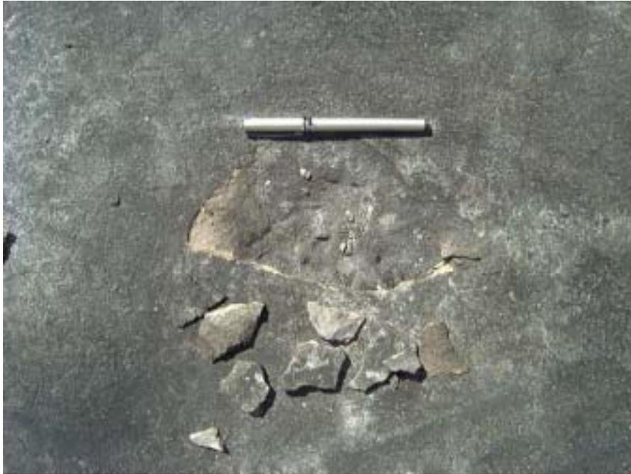
**Figure A1.6. Close-up View of Scaling at Old Alert Apron**
