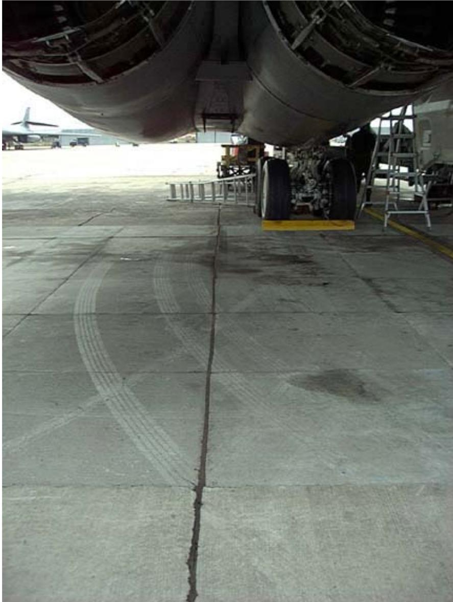
**Figure A1.8. MPC “Checkerboard” Repair Area**
