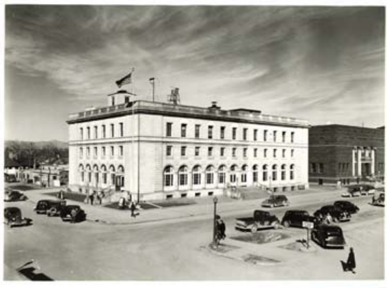
Figure J-3. 1938 addition post construction.
