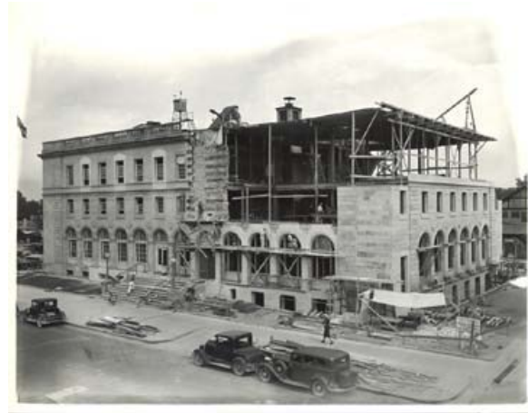
Figure J-2. 1938 addition, in construction.
