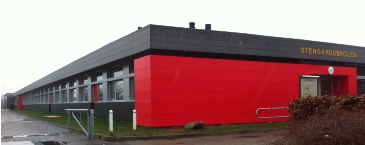
Figure B-13. Photo of renovated façade.
