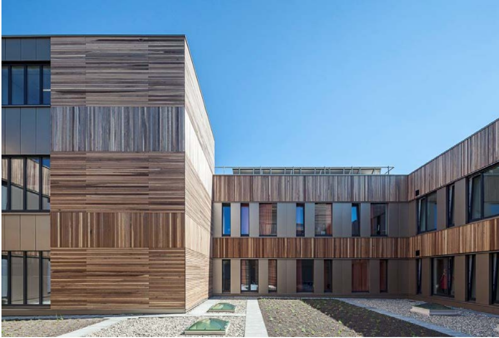
Figure H-6. Roof terrace.
