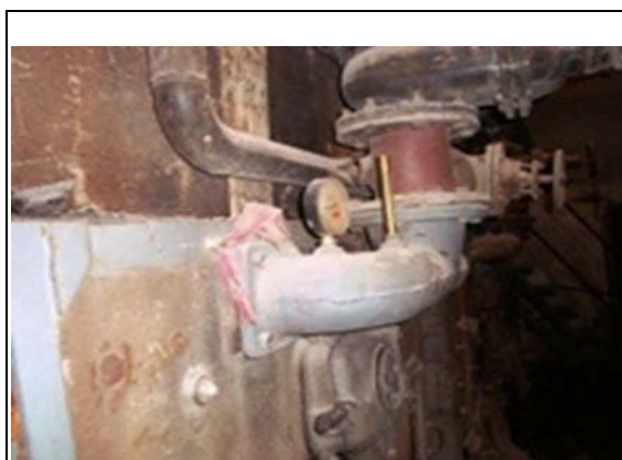
Figure G-23. Hot-water boiler – temperature and pressure measuring and hollow boiler rib.
