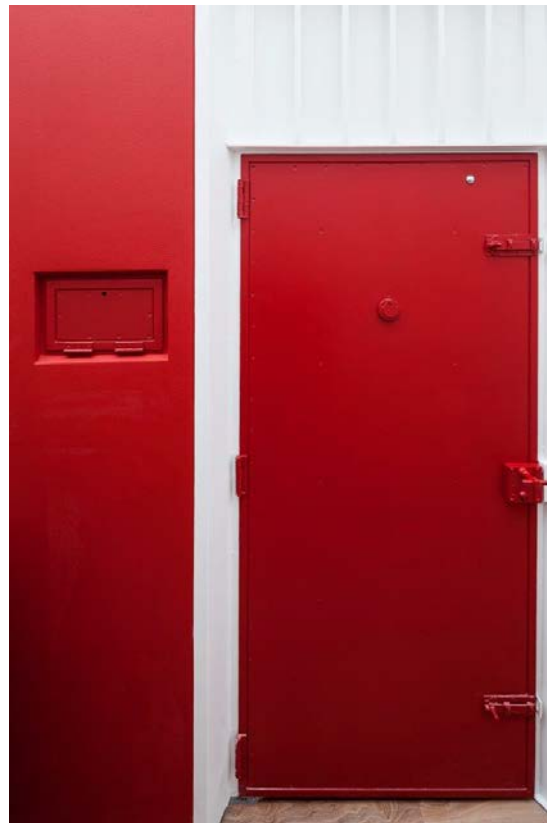
Figure H-7. Old cell doors are kept and painted.
