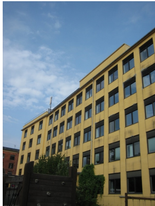
Figure B-22. Facade before renovation.
