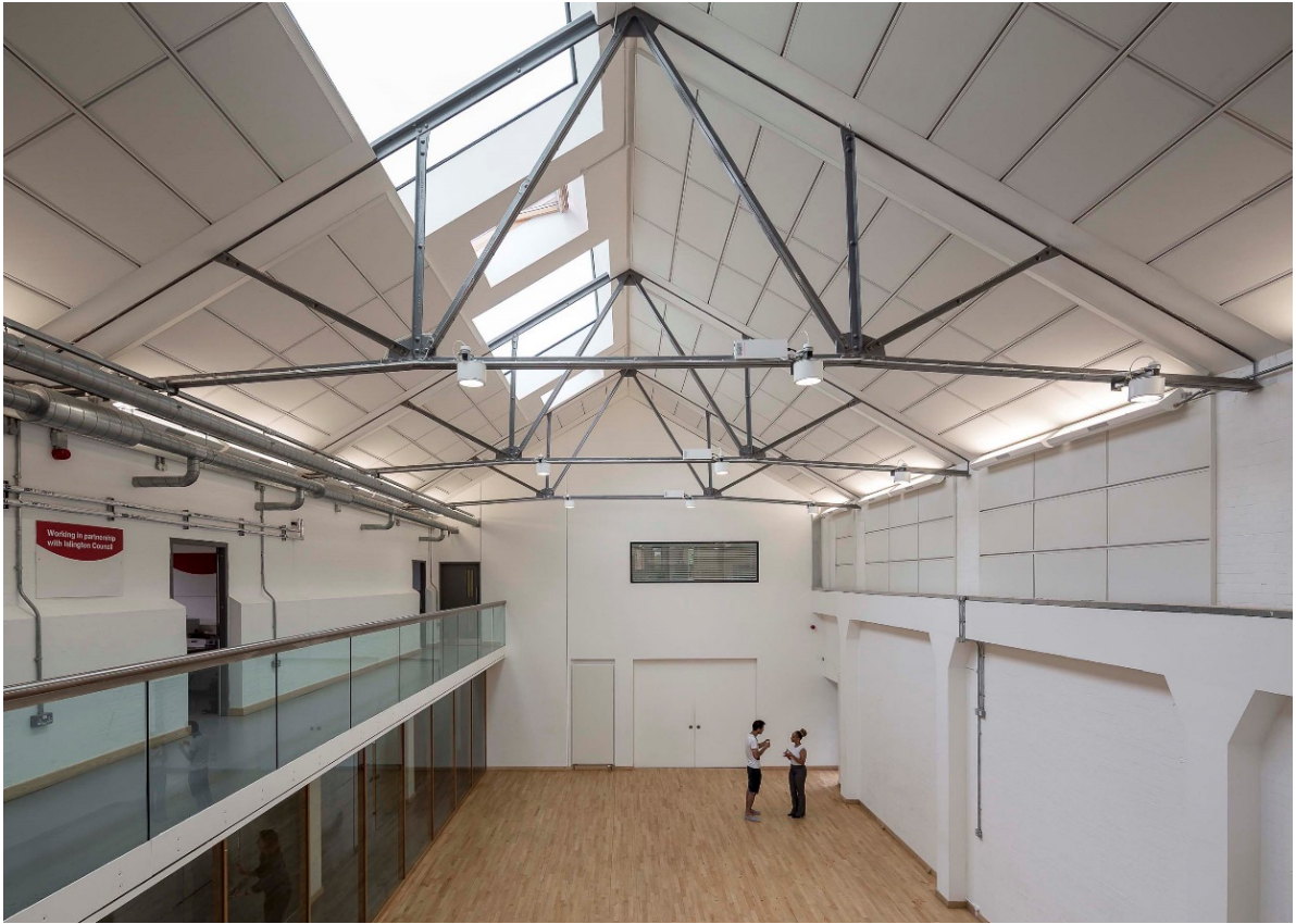
Figure I-2. After retrofit: Interior of main hall with offices to left.
