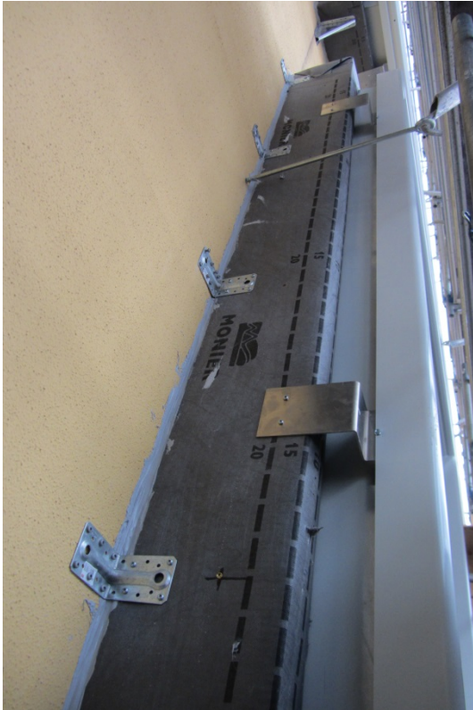
Figure B-25. Windows fastened to the existing facade
