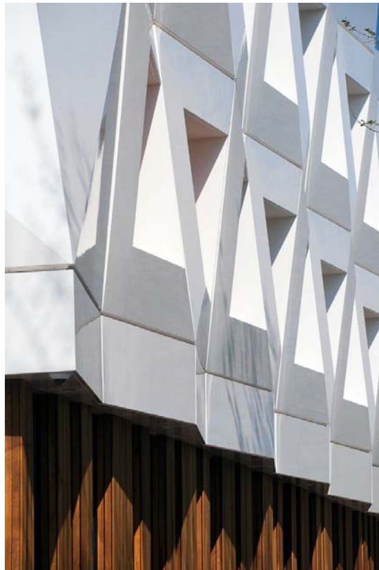
Figure H-3. Detail of paneling.
