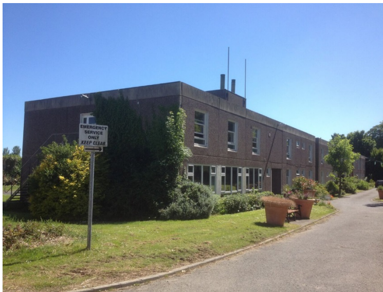
Figure E-4. Building after retrofit.
