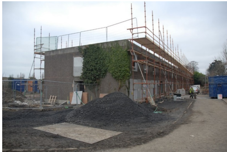
Figure E-2. Key figure during renovation process.
