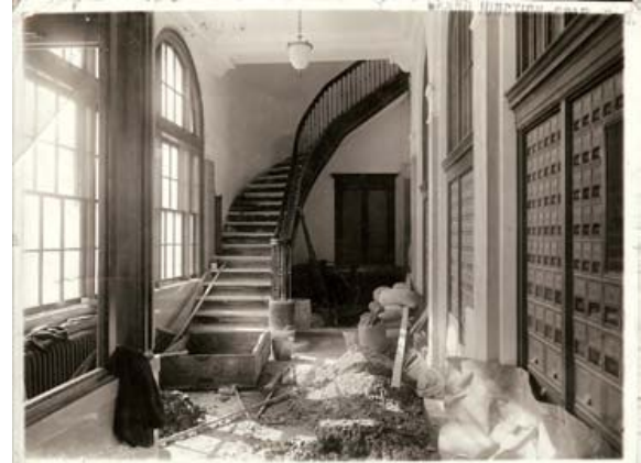
Figure J-4. 1918 interior construction.
