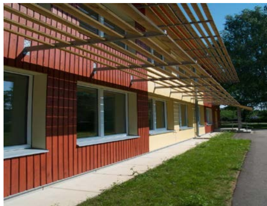
Figure C-6. After refurbishment – overhangs for summer heat protection.
