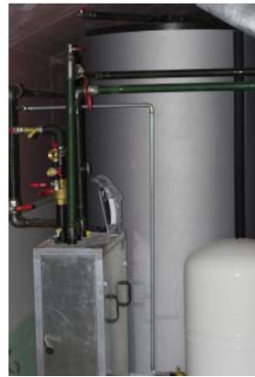
Figure C-11. Installed solar thermal system
