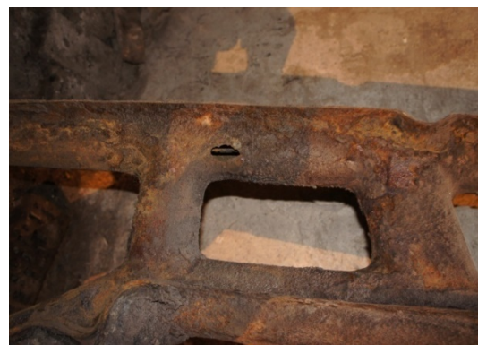
Figure G-24. Water boiler – temperature and pressure measuring and hollow boiler rib.
