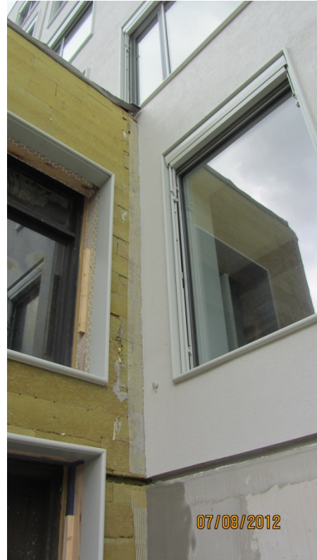
Figure B-26. Insulation and new windows installed.
