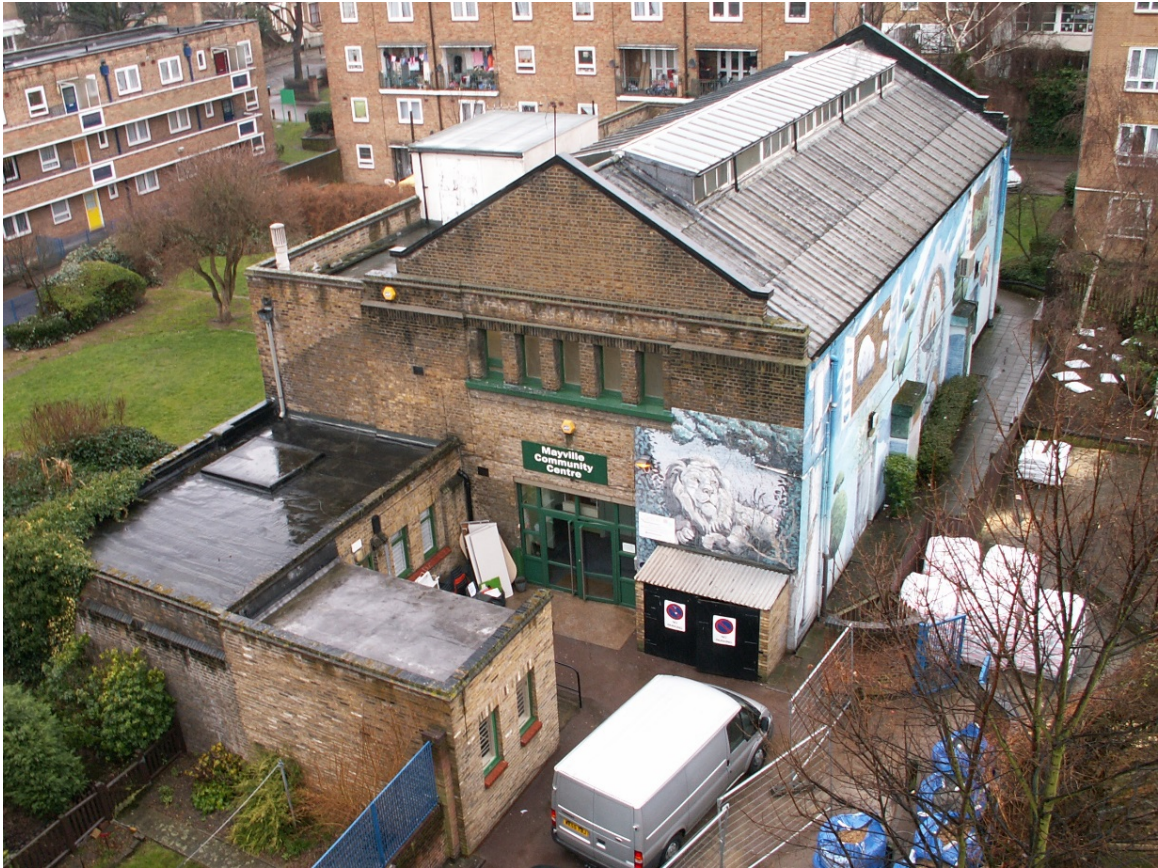
Figure I-4. Before retrofit: East elevation.
