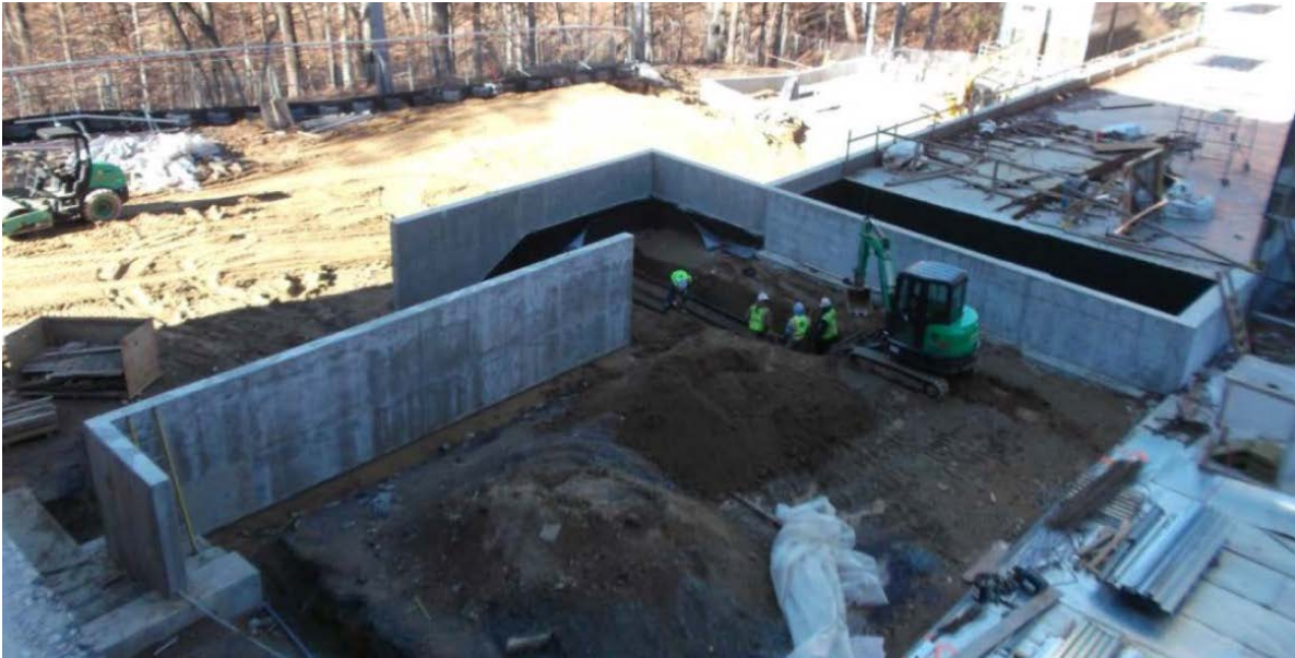
Figure J-26. Utilities installation.
