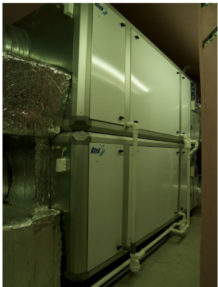
Figure C-12. Ventilation with heat recovery.
