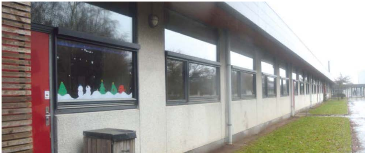
Figure B-12. Photo of existing façade.
