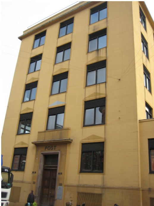
Figure B-21. Facade before renovation.
