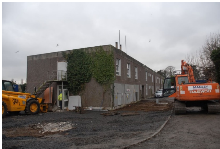
Figure E-1. Building before retrofit.
