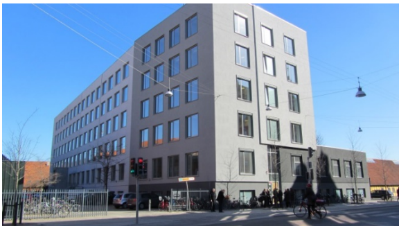
Figure B-23. Facade after renovation.
