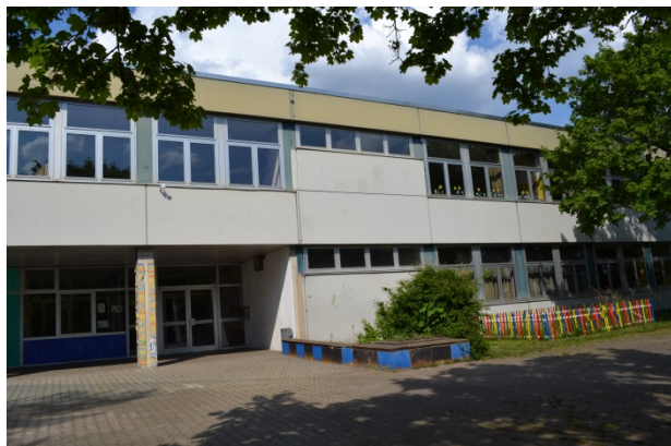
Figure D-8. The building in its original state.
