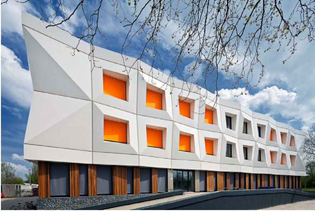
Figure H-2. Entrance, renovated façade.
