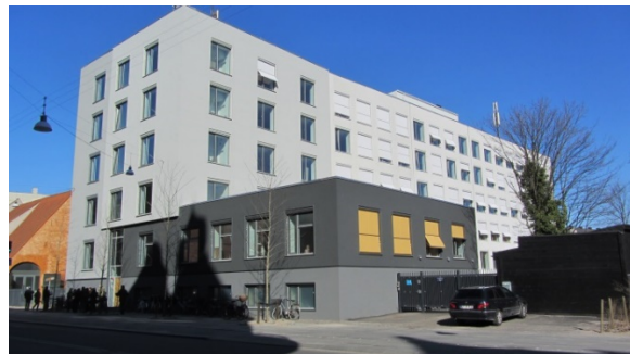
Figure B-24. Facade after renovation.
