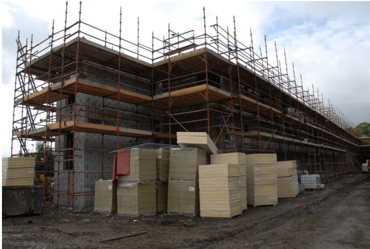
Figure E-3. Key figure during renovation process.
