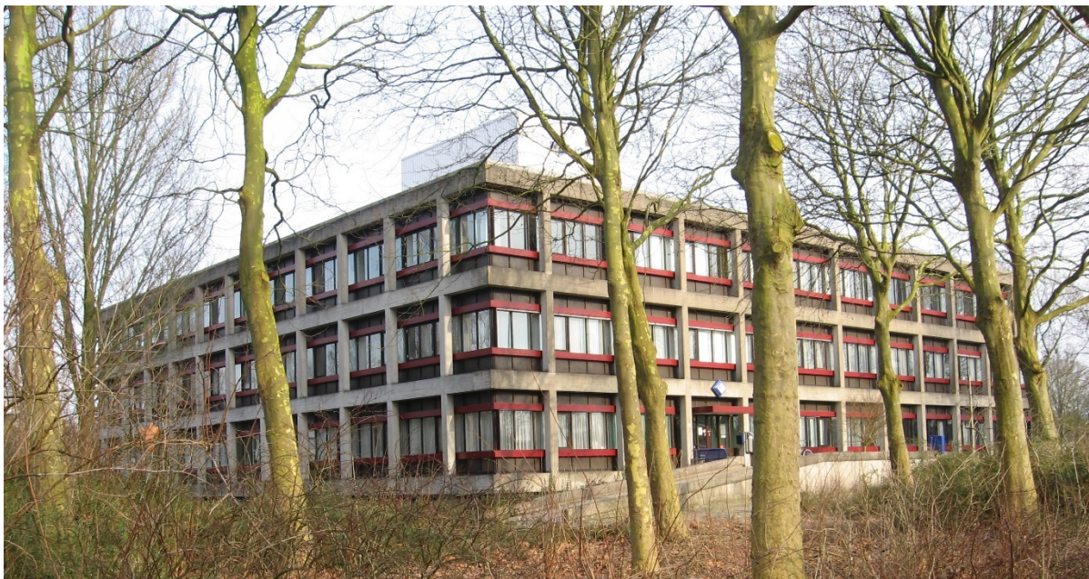
Figure H-1. Facade before retrofit.
