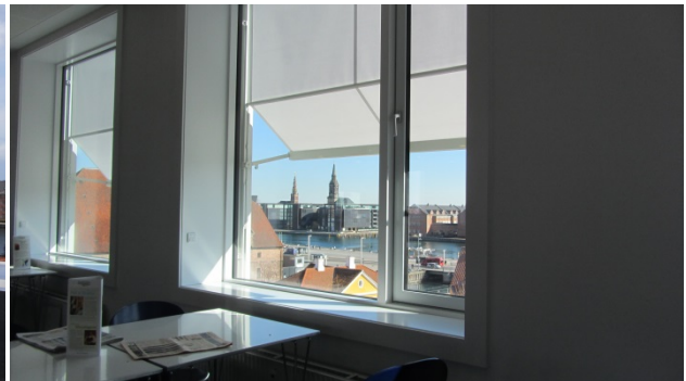
Figure B-28. Solar shading, adjustable vertical/horizontal.
