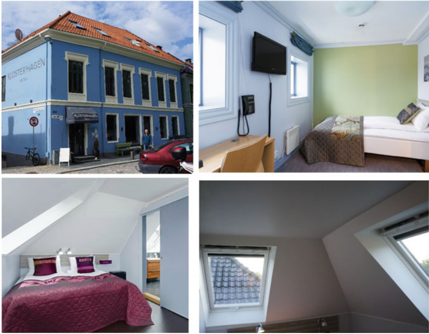
Fig. 3.17 Example of attic renovation at the Klosterhagen Hotel in Bergen
