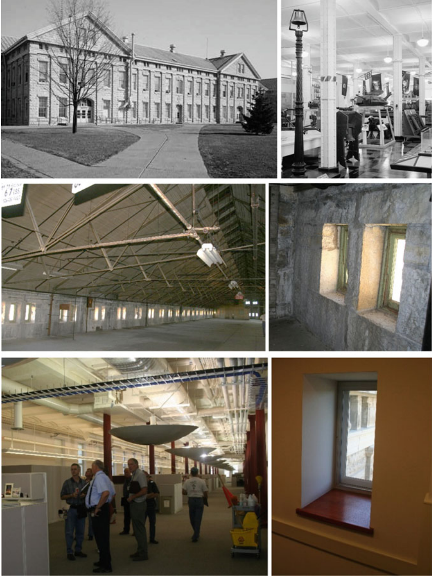
Fig. 3.18 Example of attic renovation of the building at Rock Island Arsenal. Source Library of Congress (a, b); Alexander Zhivov (c-f)
