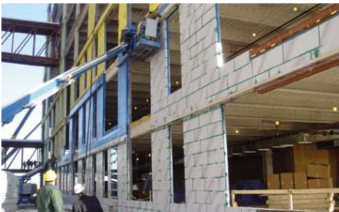
ABAA on-site audit in progress. Children's Hospital, Wauwatosa, WI.
