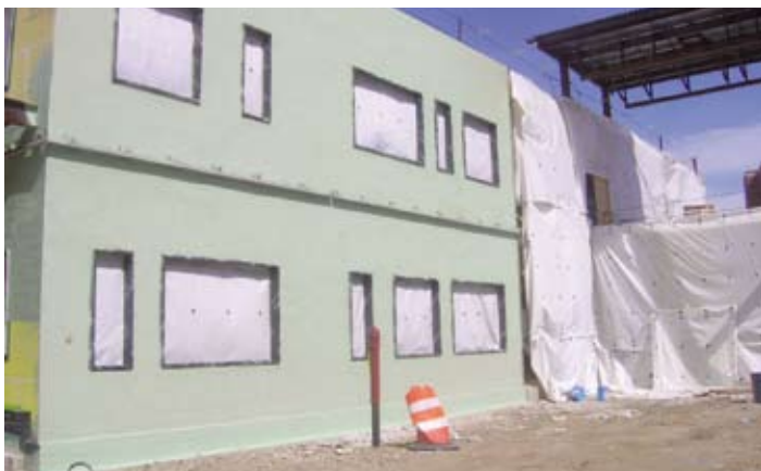
ABAA specified project. Milford Hospital project in Milford, MA.
