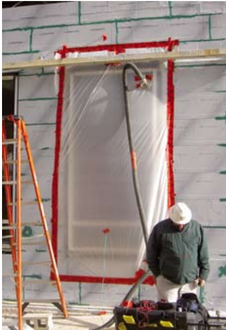
ASTM 1186 Smoke Test performed on the actual building enclosure.
